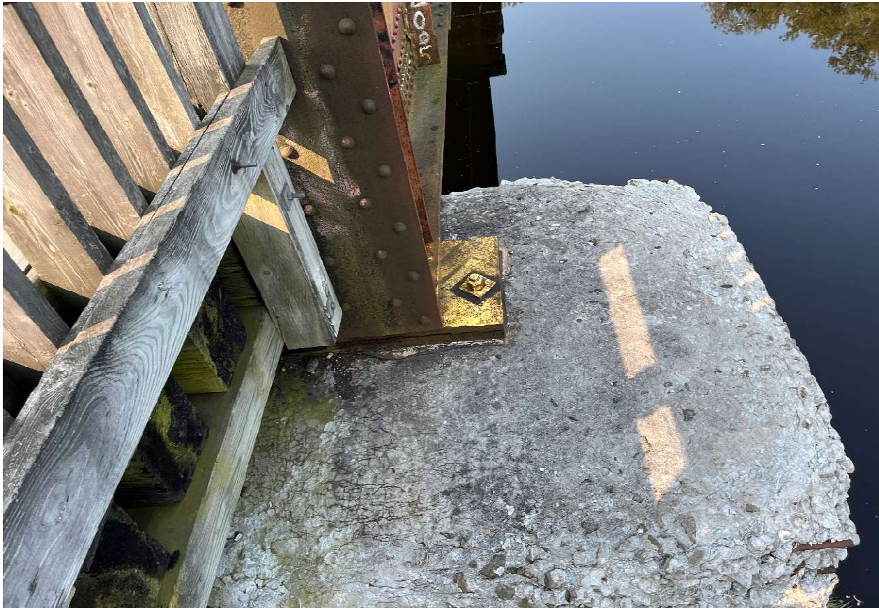
Description of Photo: Pier bearings
