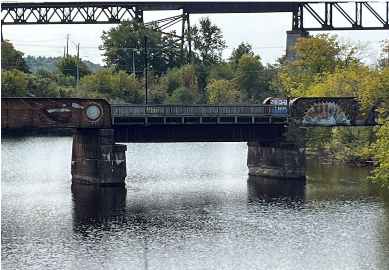
Description of Photo: Deck Plate girder span
