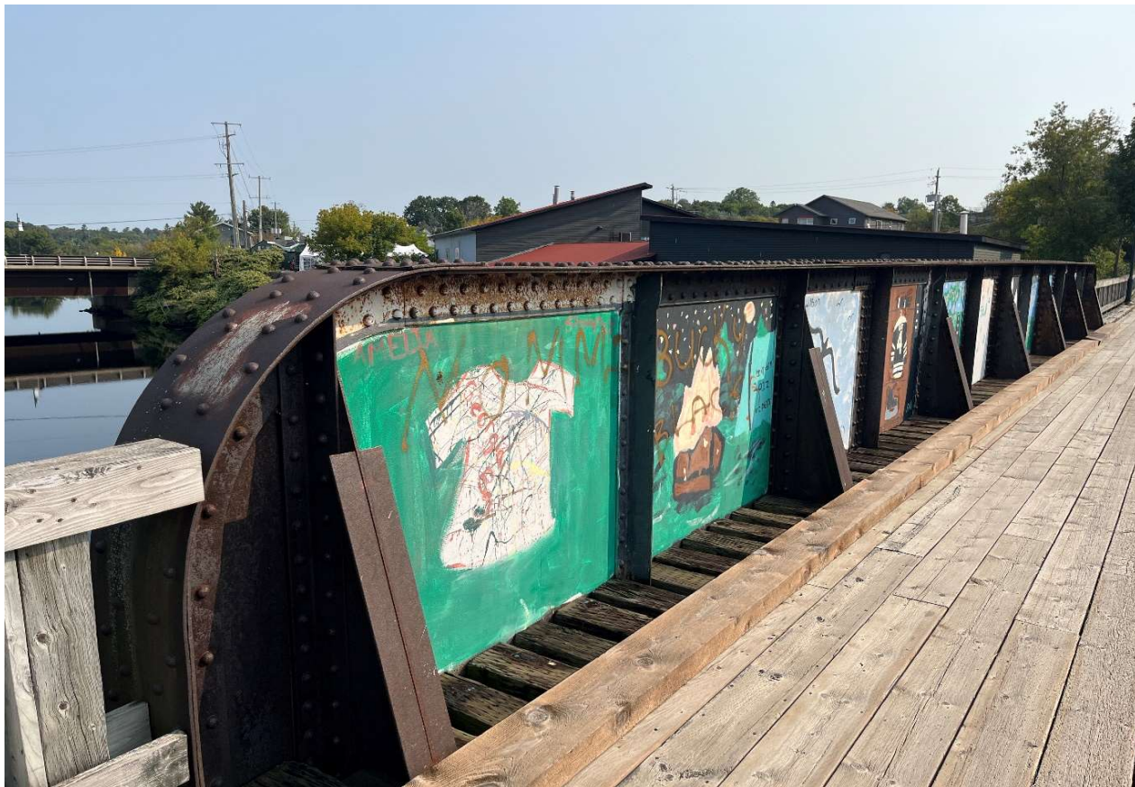
Description of Photo: Inside face of girder
