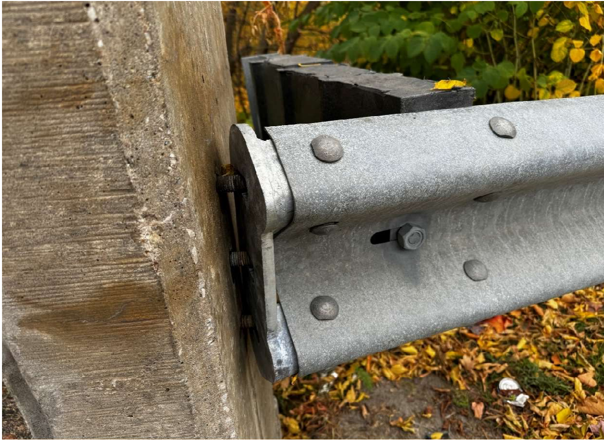
Description of Photo: Northwest approach railing
