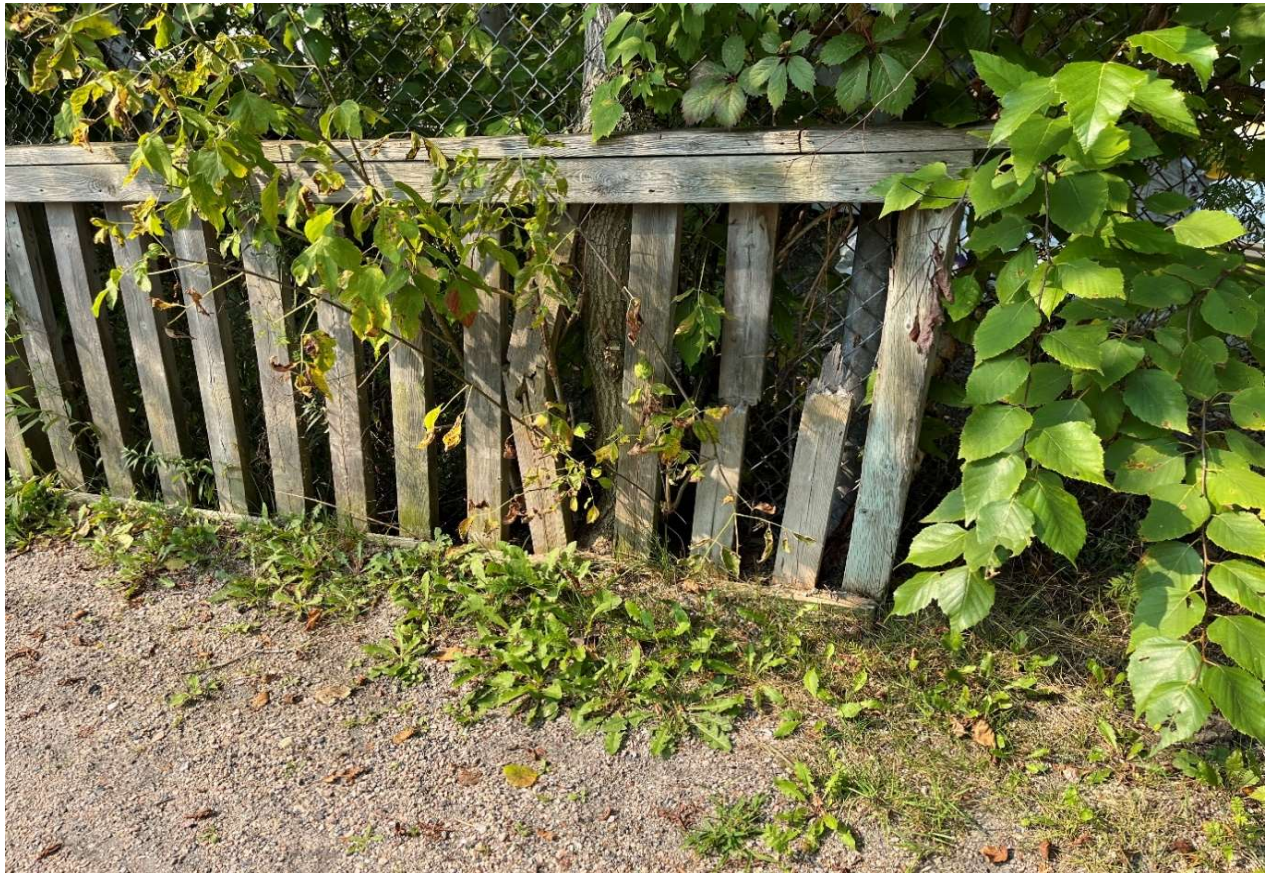
Description of Photo: Railing system
