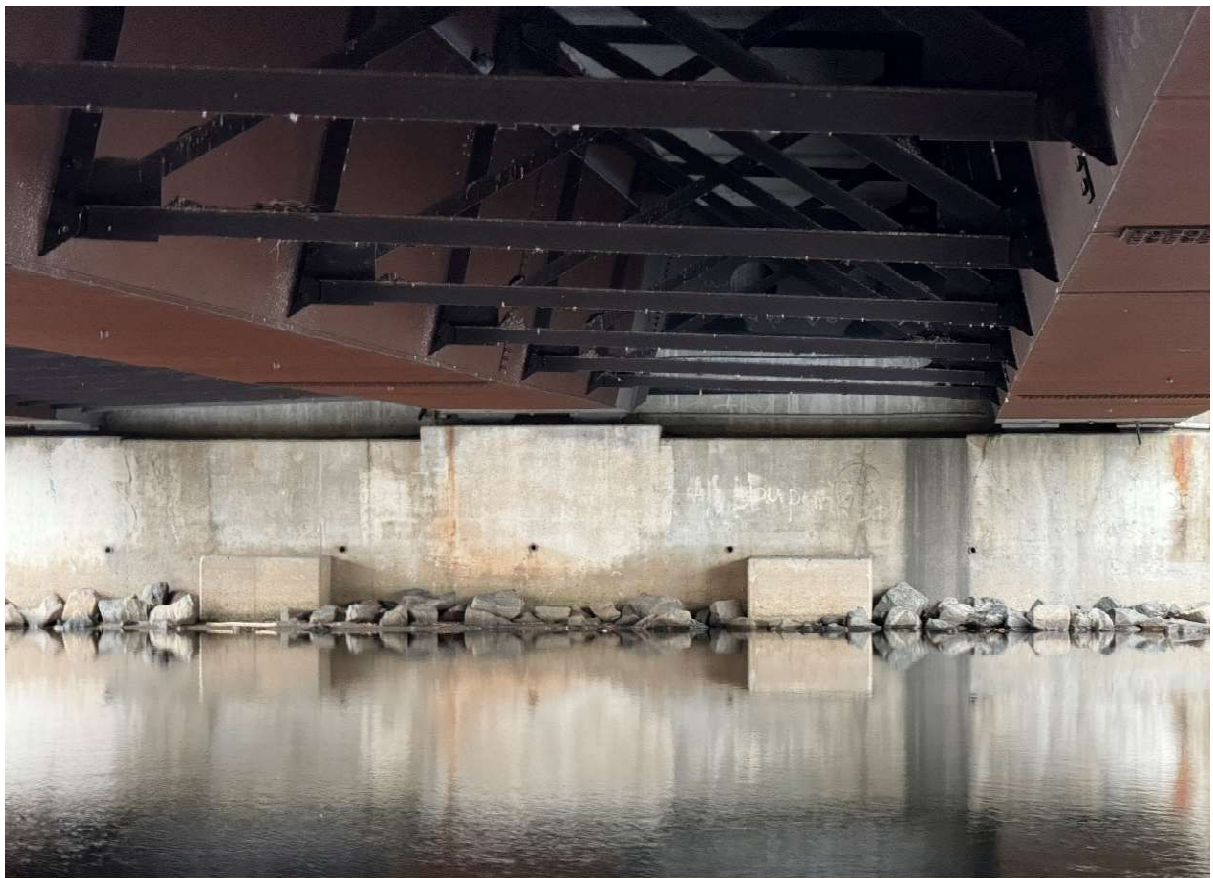
Description of Photo: Rock protection
