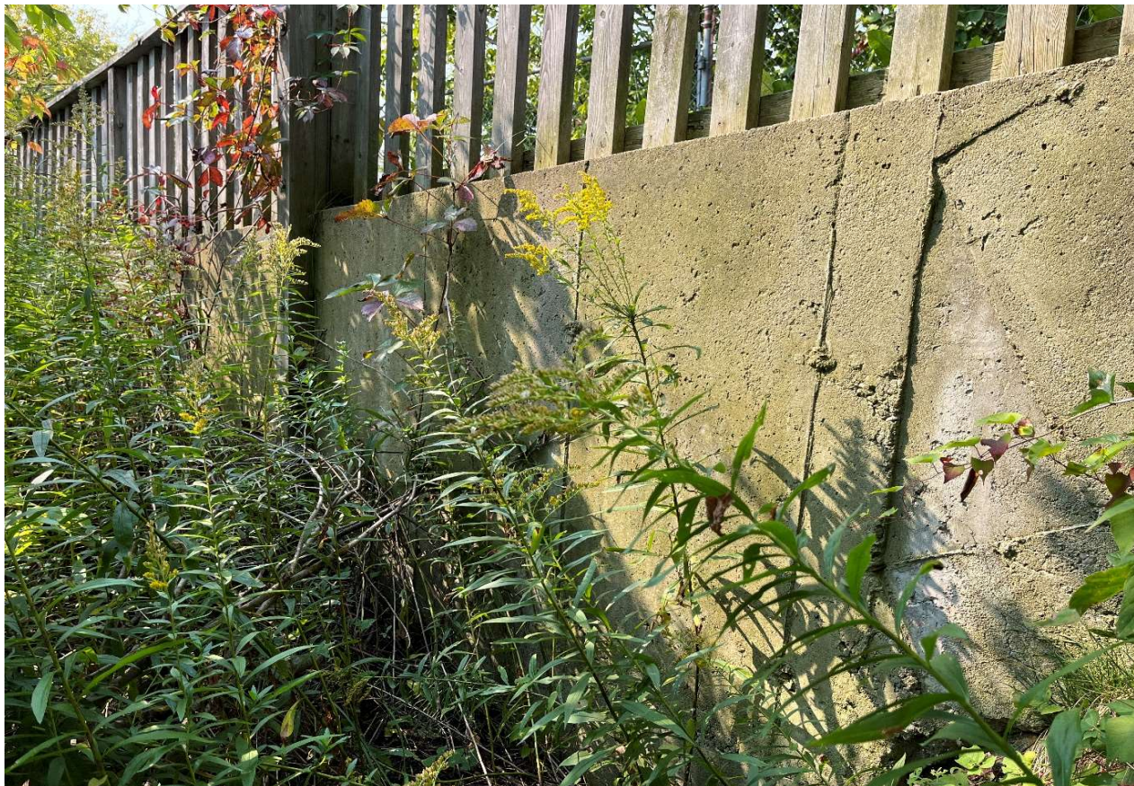
Description of Photo: Retaining wall
