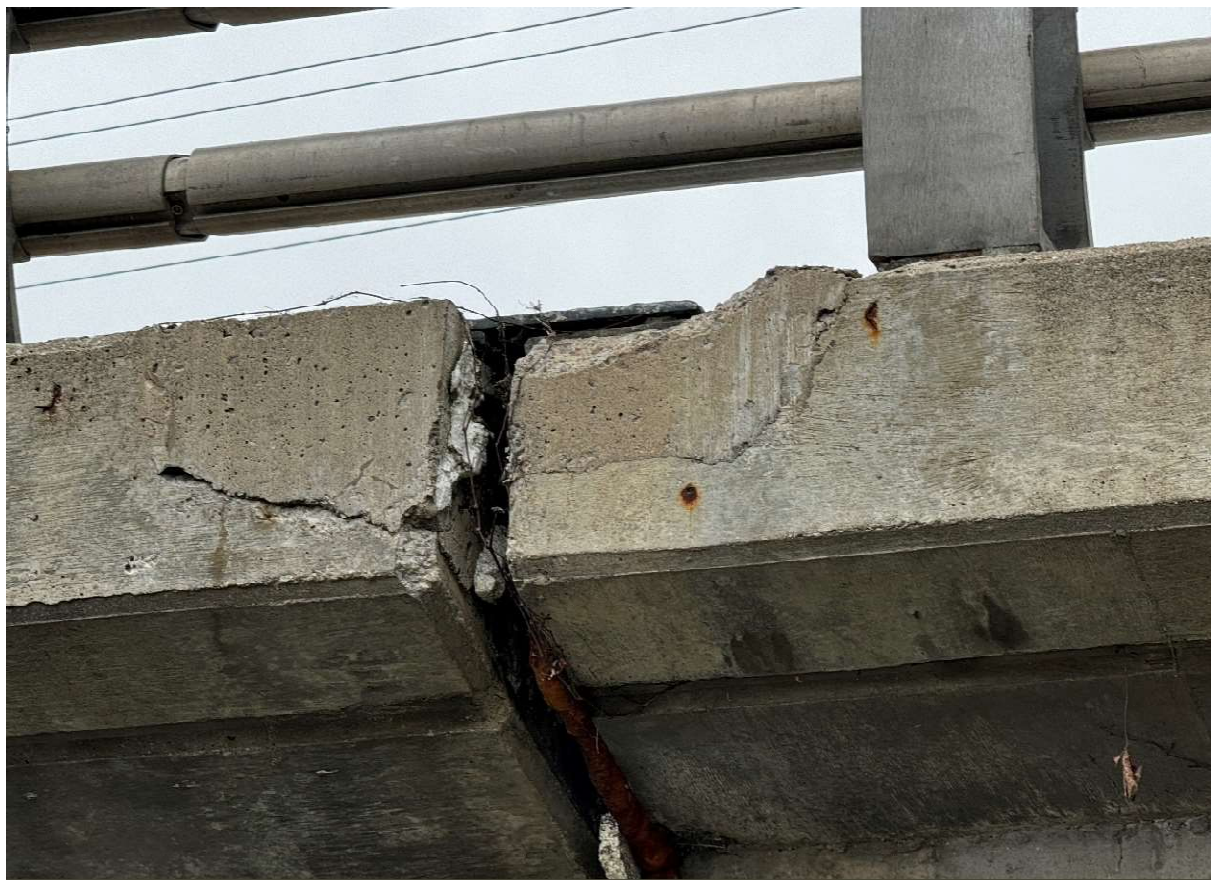
Description of Photo: Exterior soffit
