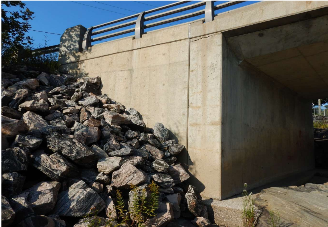
Description of Photo: Northwest wingwall
