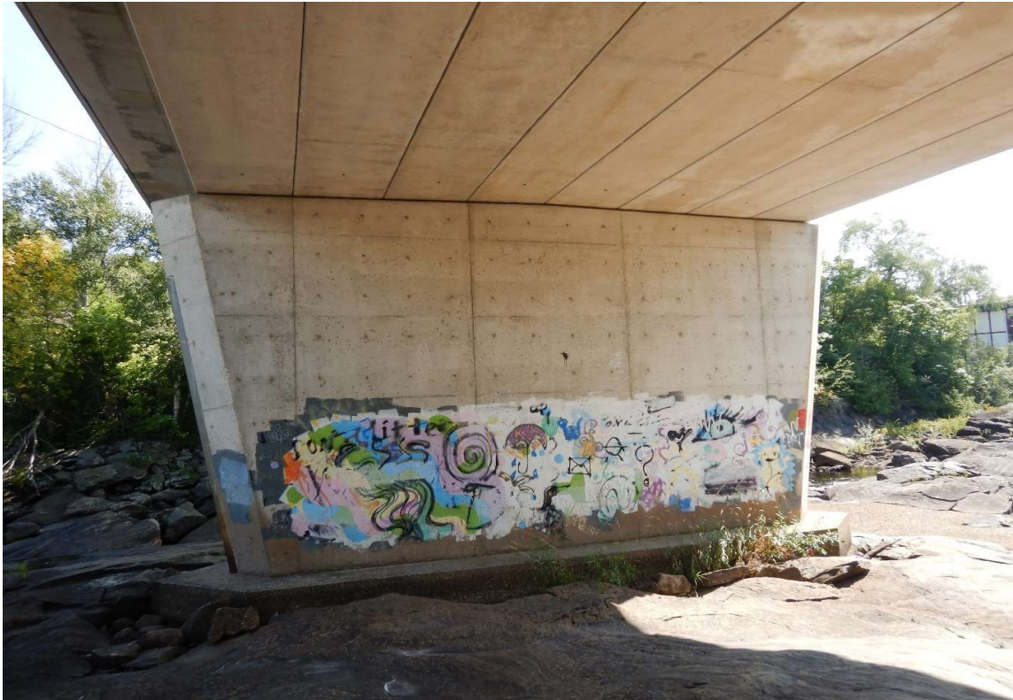
Description of Photo: Pier
