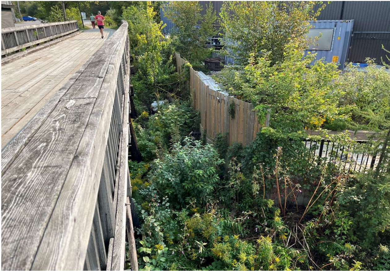
Description of Photo: Embankment
