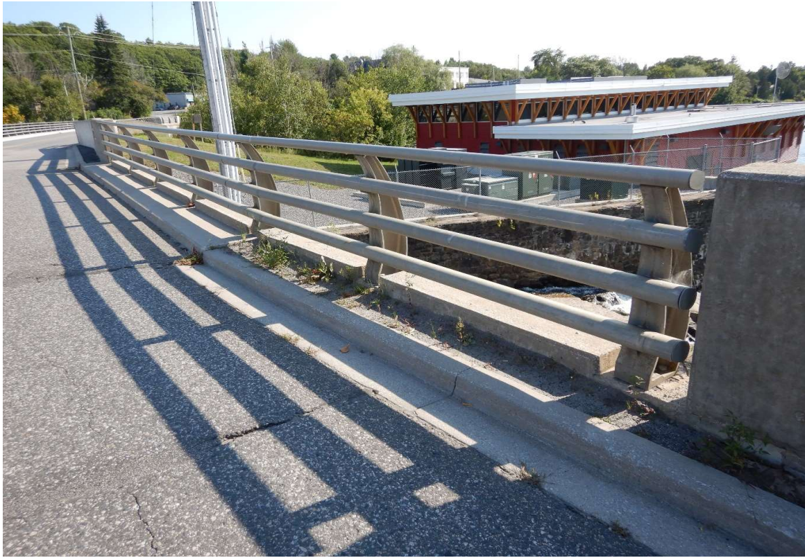
Description of Photo: West Railing System
