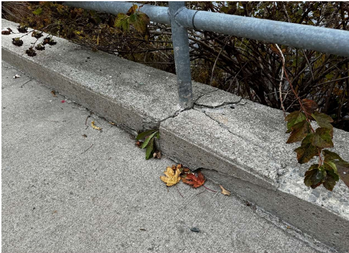
Description of Photo: Retaining wall
