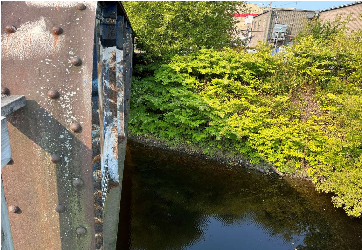
Description of Photo: Embankment
