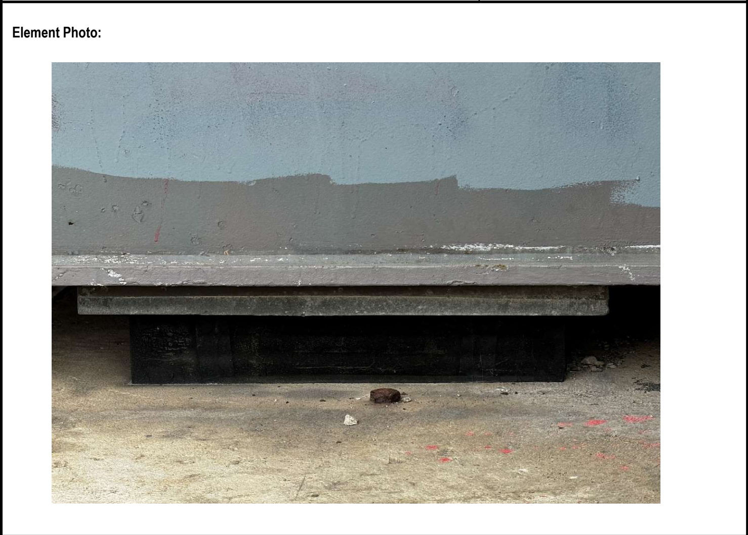
Description of Photo: Bearings
