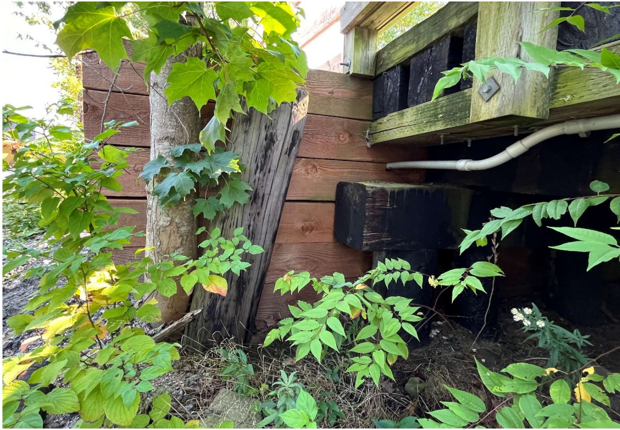
Description of Photo: East abutment
