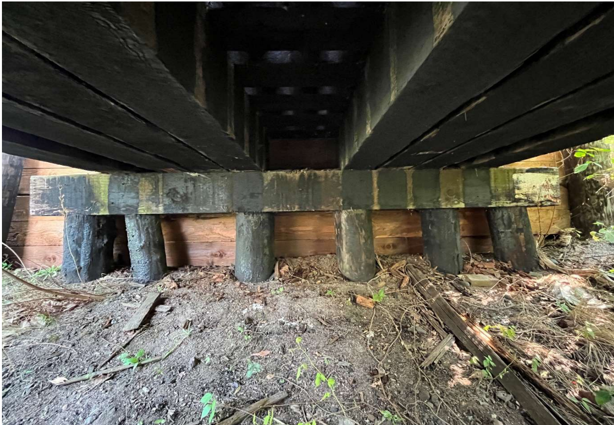
Description of Photo: Abutment piles
