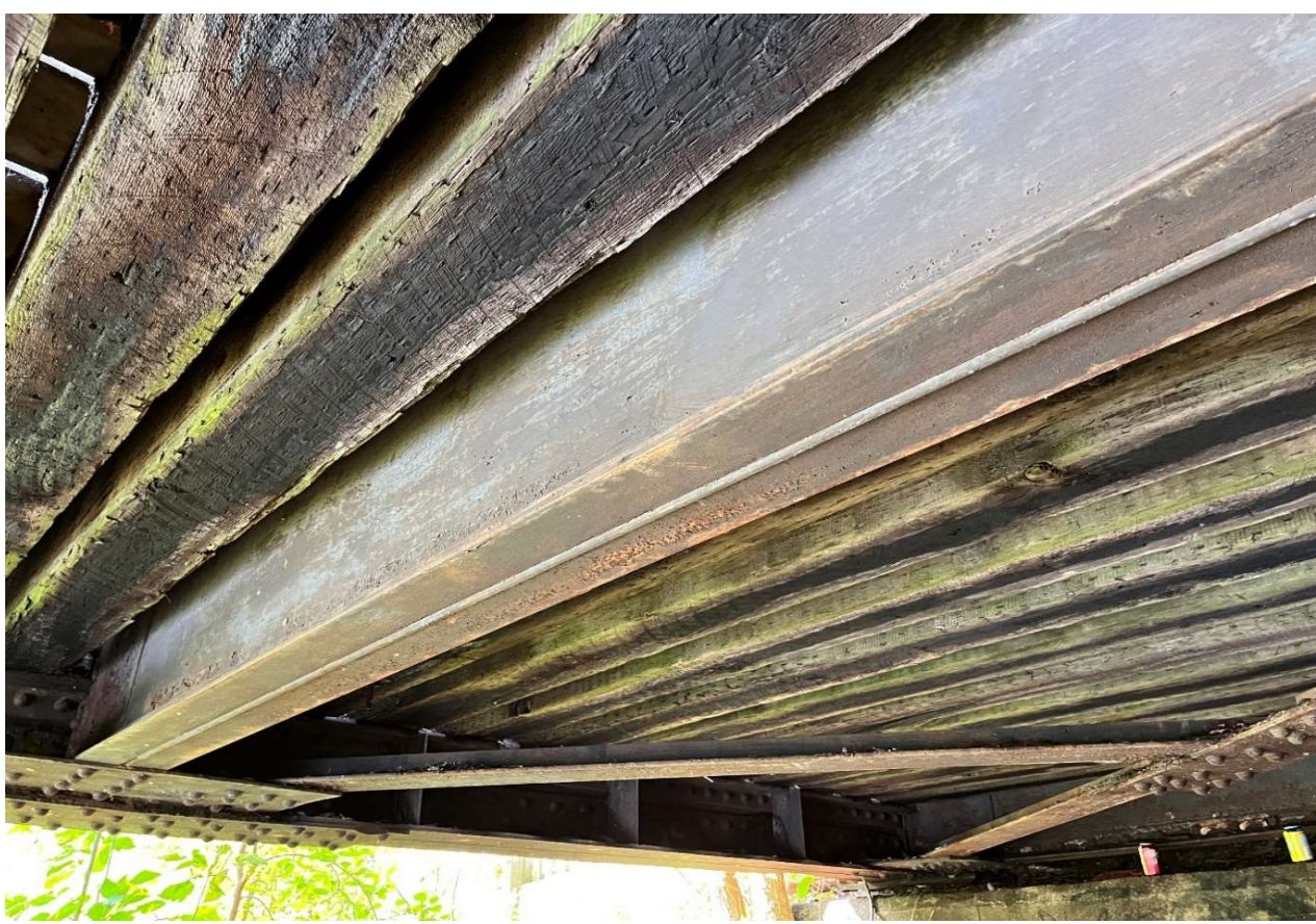
Description of Photo: Floor beams
