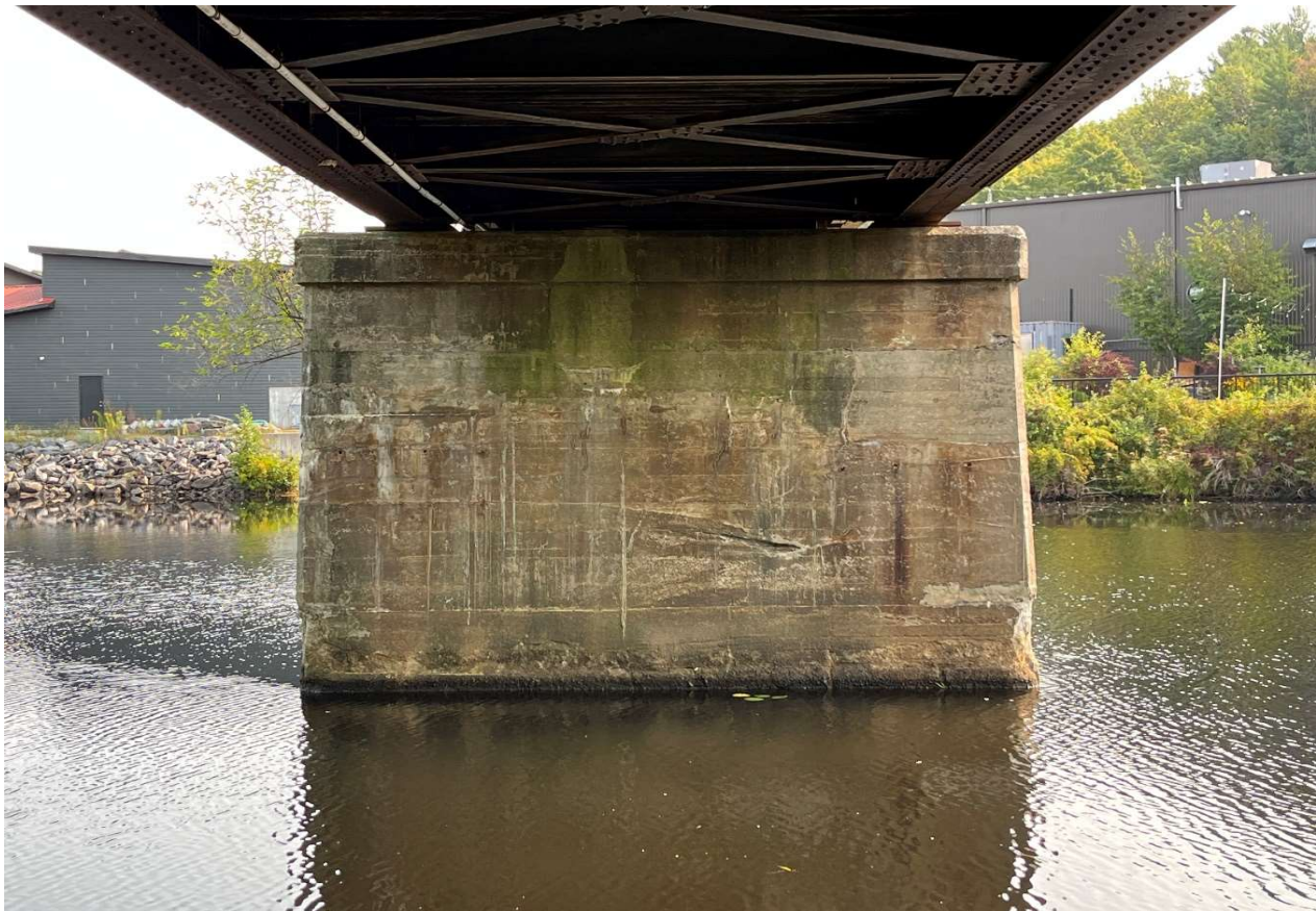
Description of Photo: West pier west face
