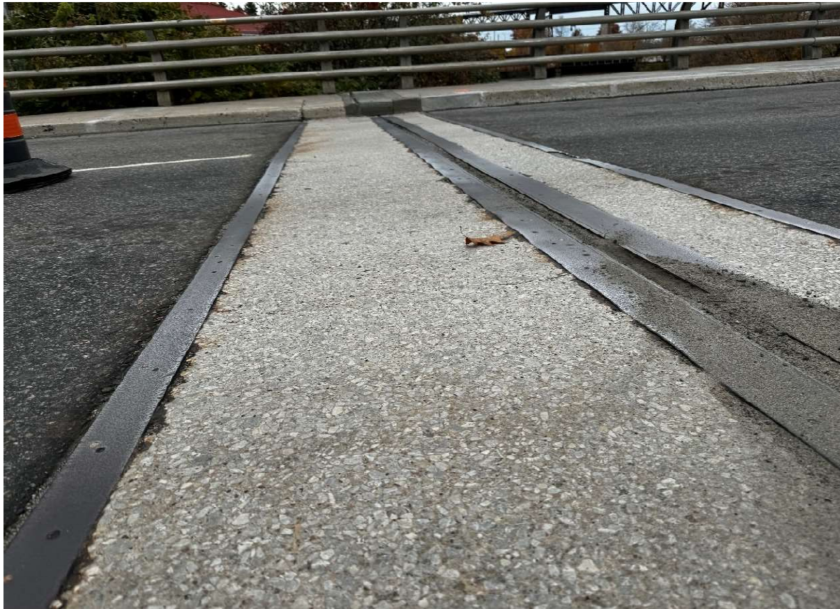
Description of Photo: Concrete end dams
