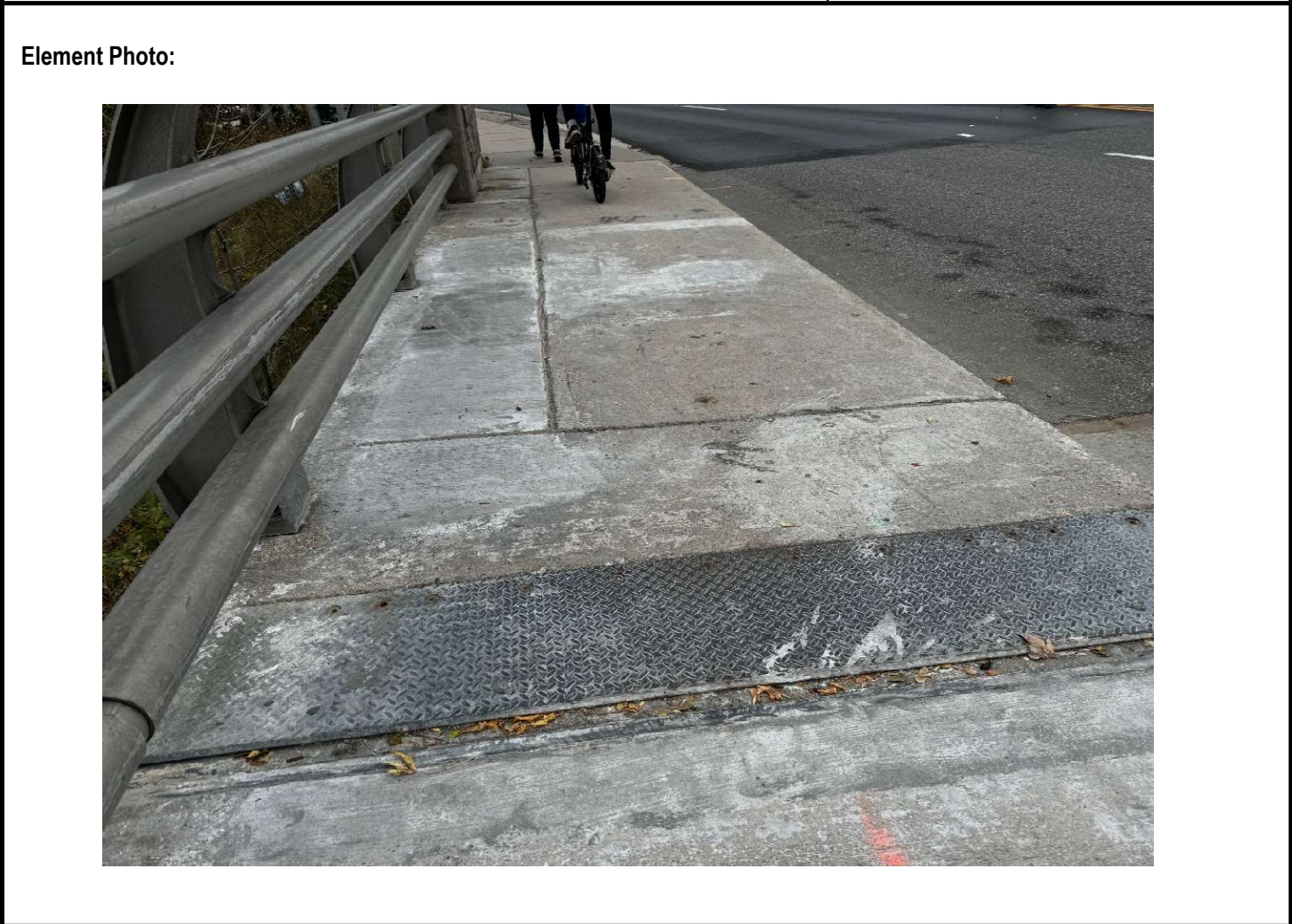
Description of Photo: Approach sidewalk
