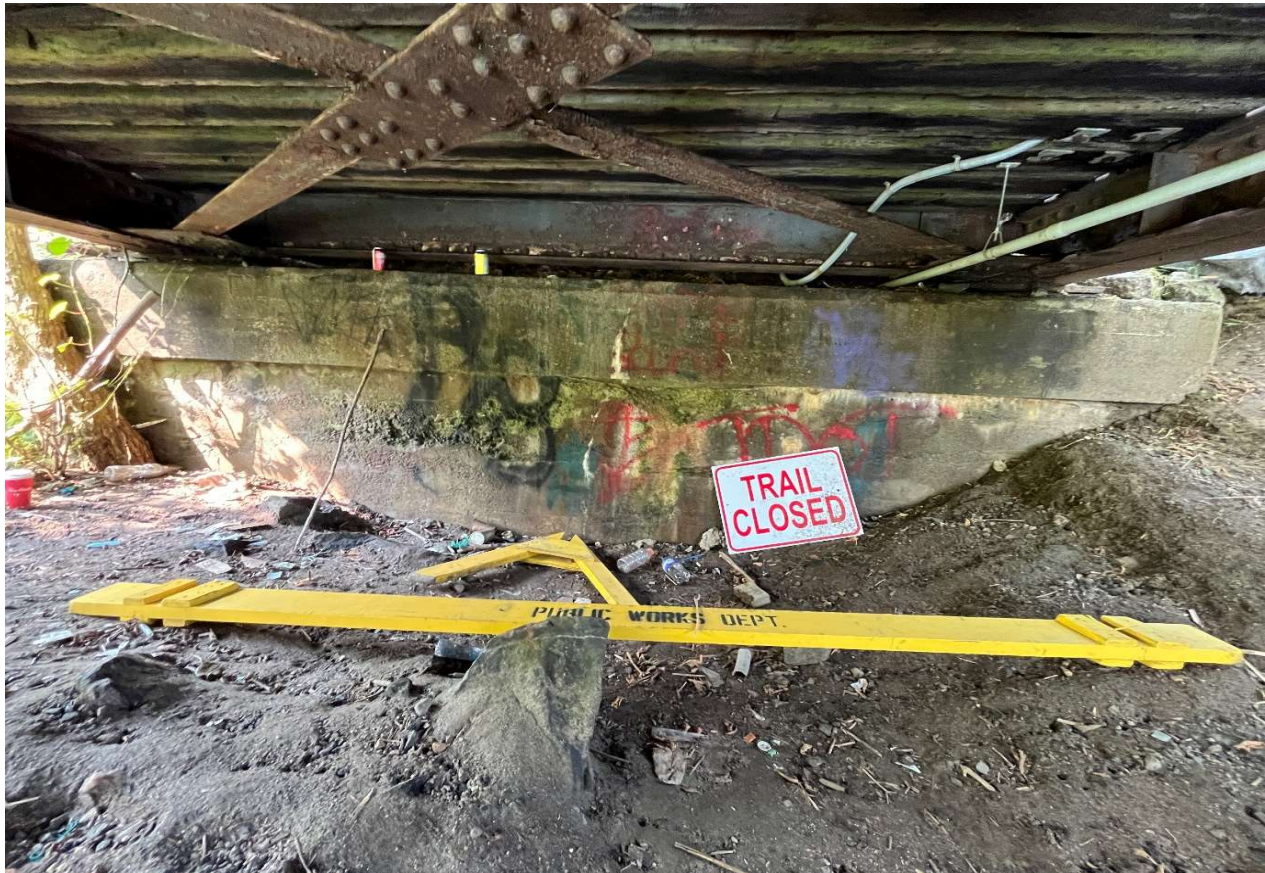
Description of Photo: West abutment
