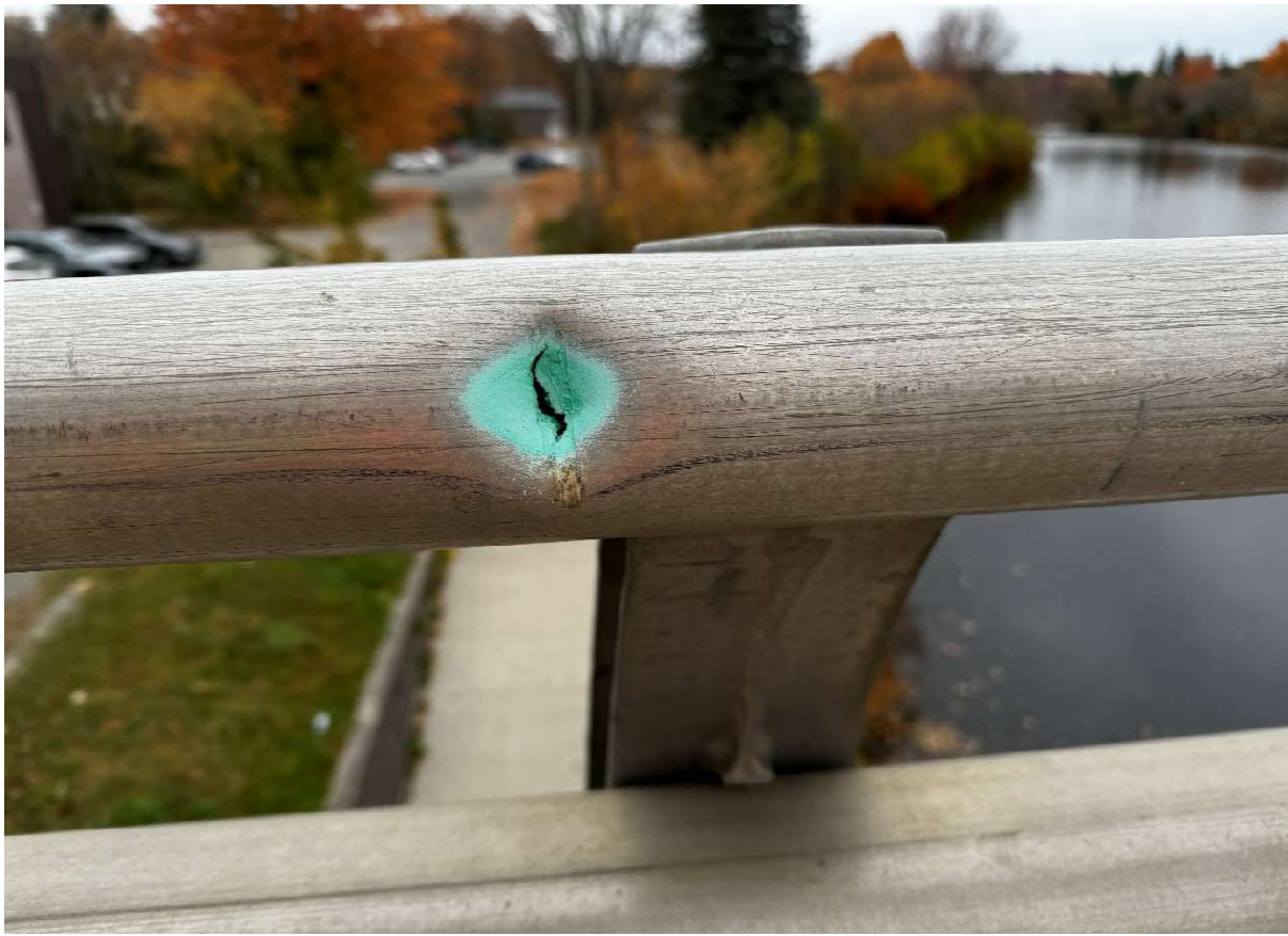
Description of Photo: North rail perforations
