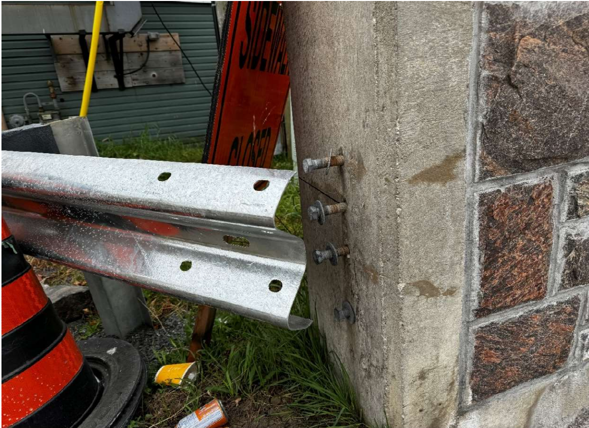
Description of Photo: Southwest approach railing, to be installed in January 2025
