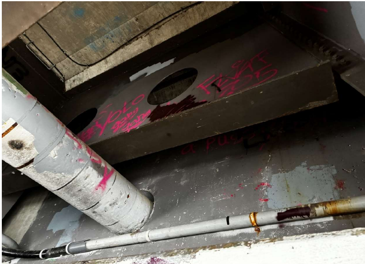
Description of Photo: Ballast wall
