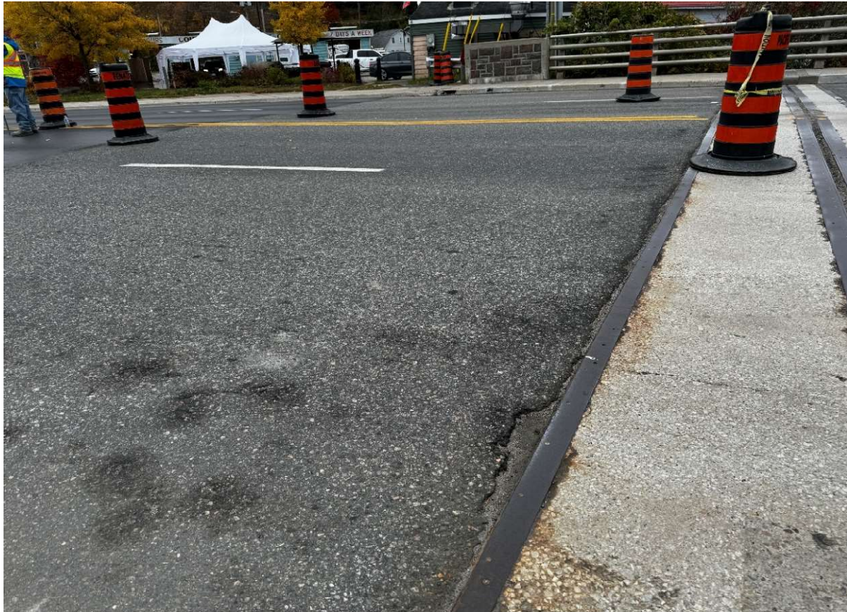
Description of Photo: East approach
