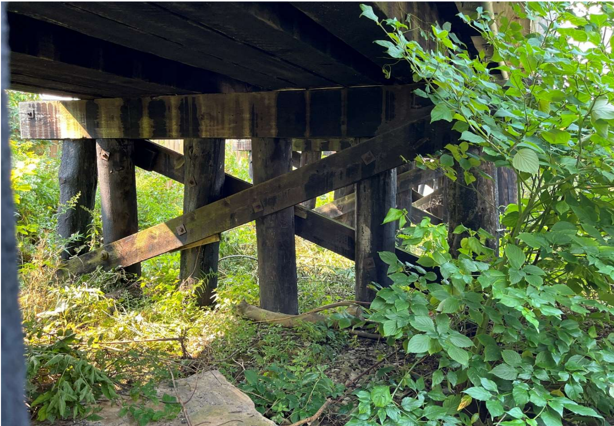
Description of Photo: Pier column bracings
