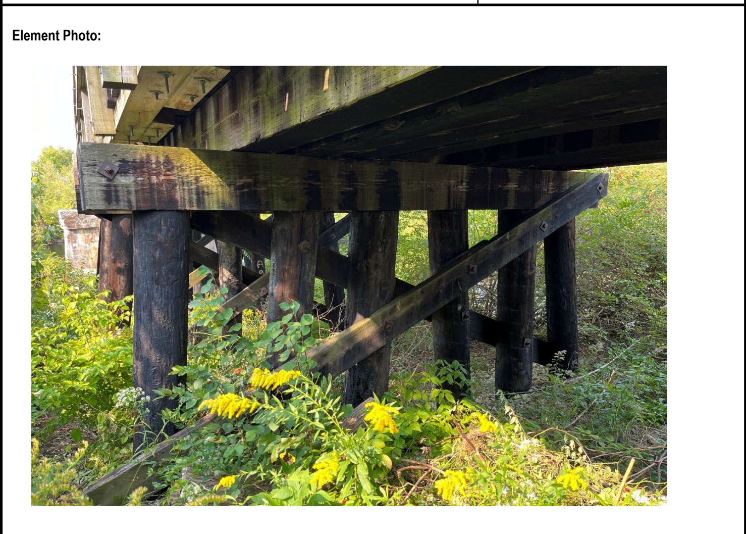
Description of Photo: Pier cap
