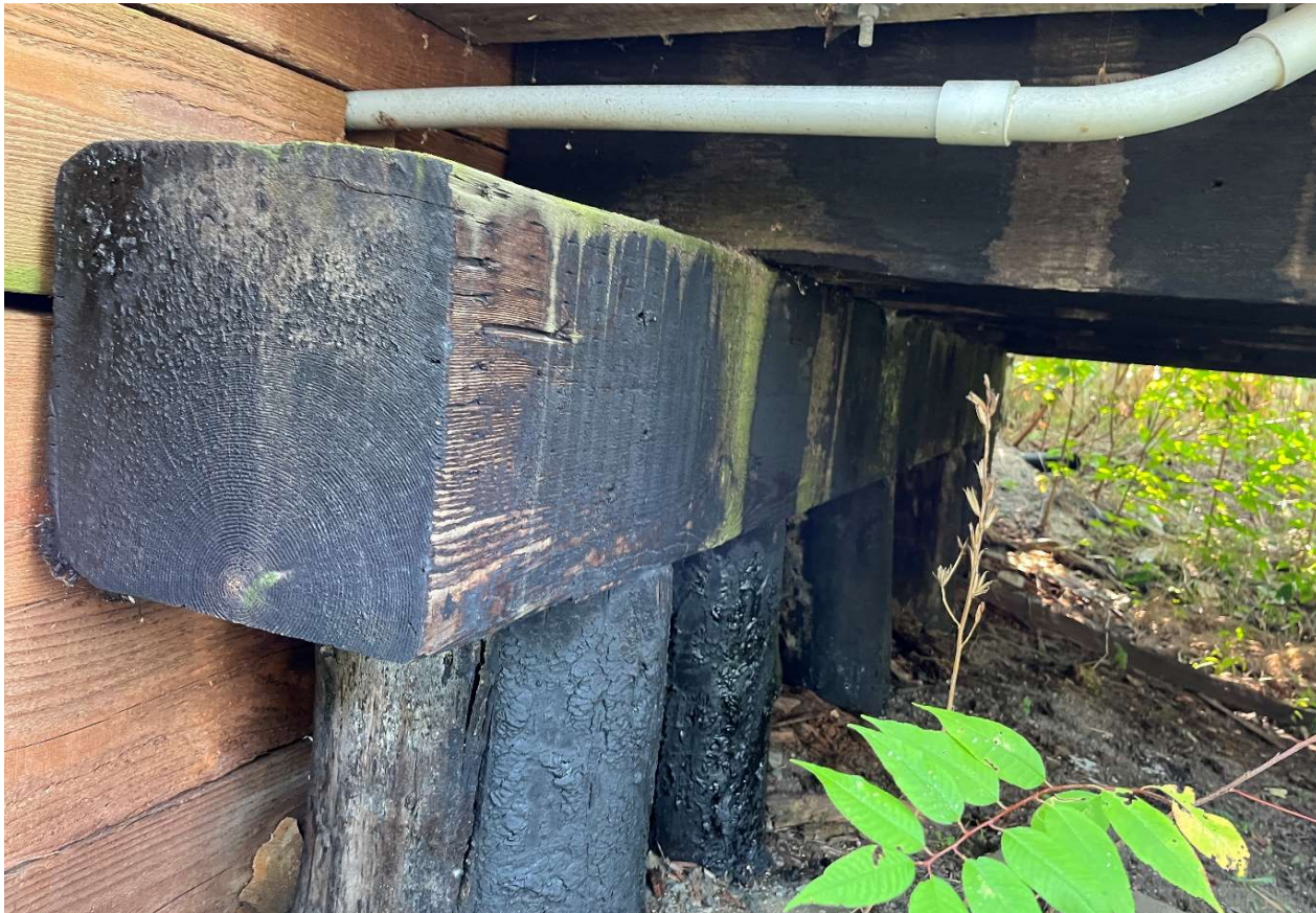
Description of Photo: Abutment cap
