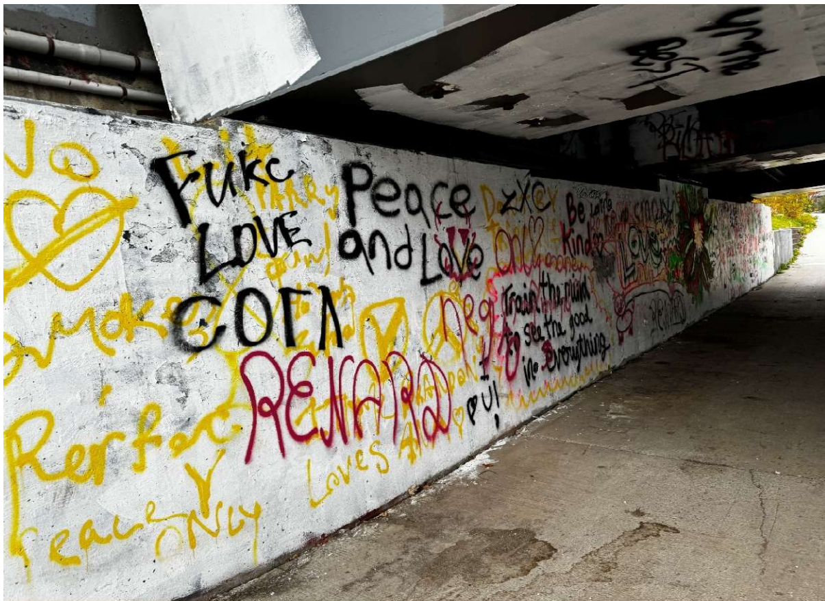
Description of Photo: Abutment wall
