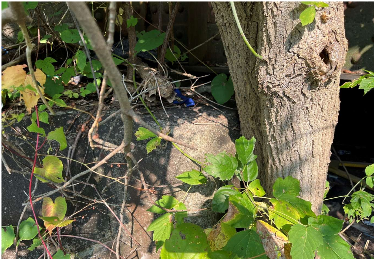
Description of Photo: Wingwall
