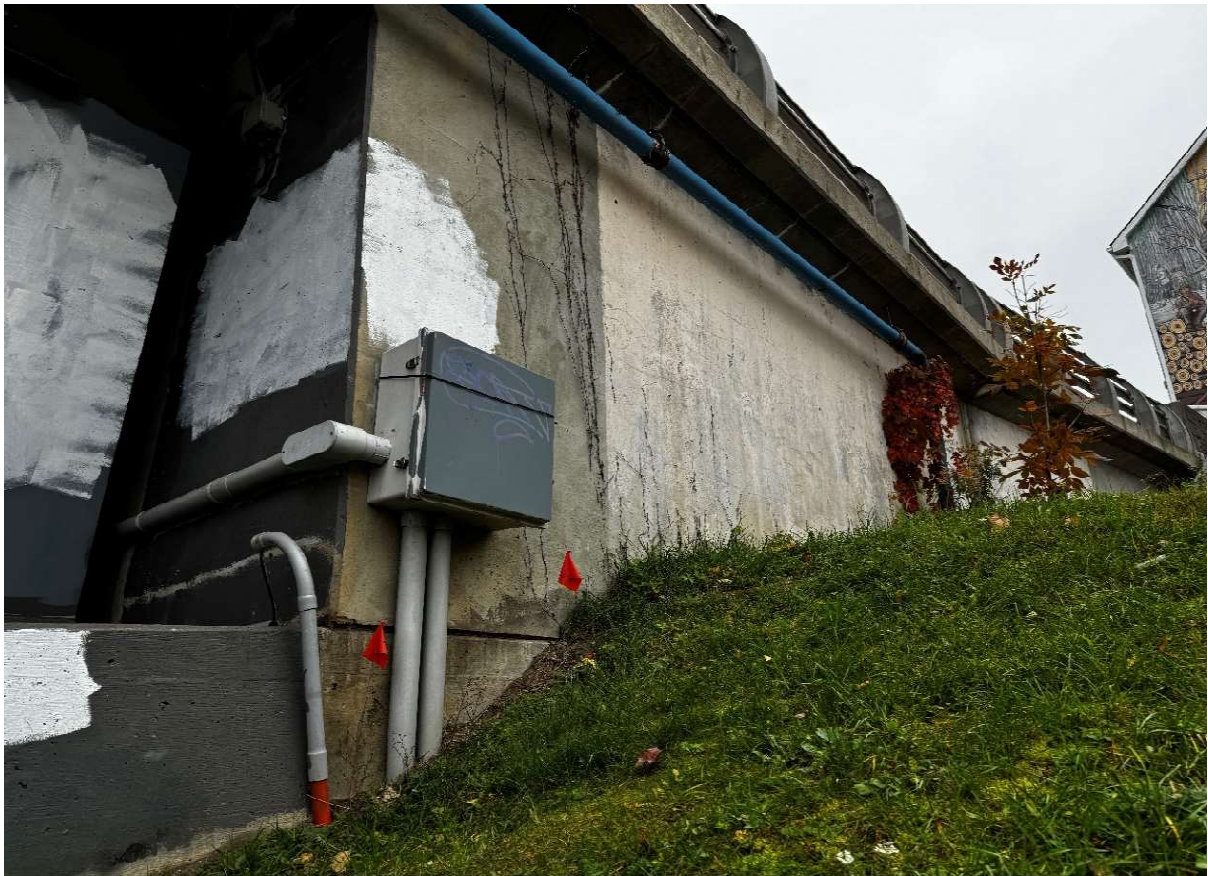
Description of Photo: Wingwall
