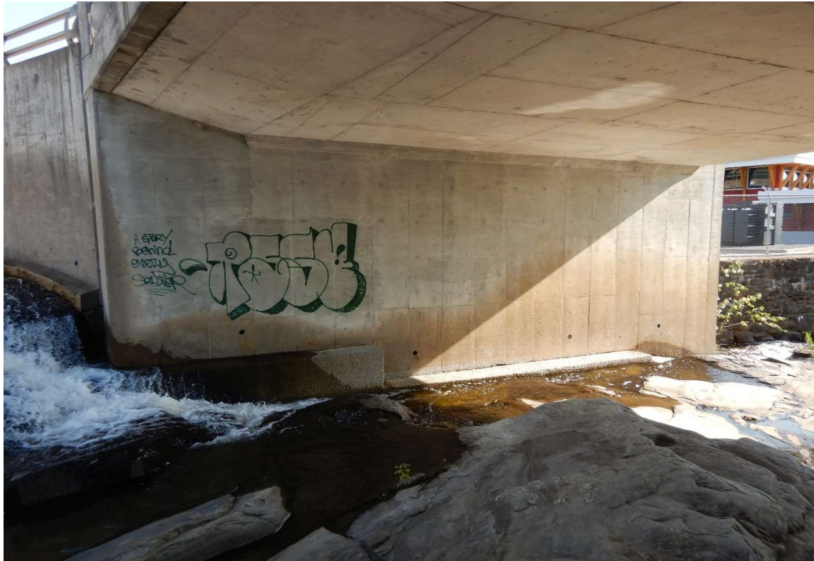
Description of Photo: South Abutment
