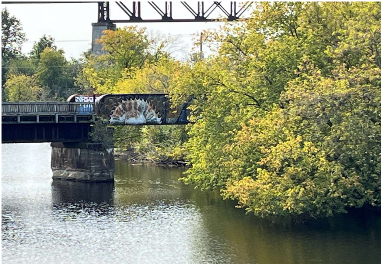
Description of Photo: West through plate girder span
