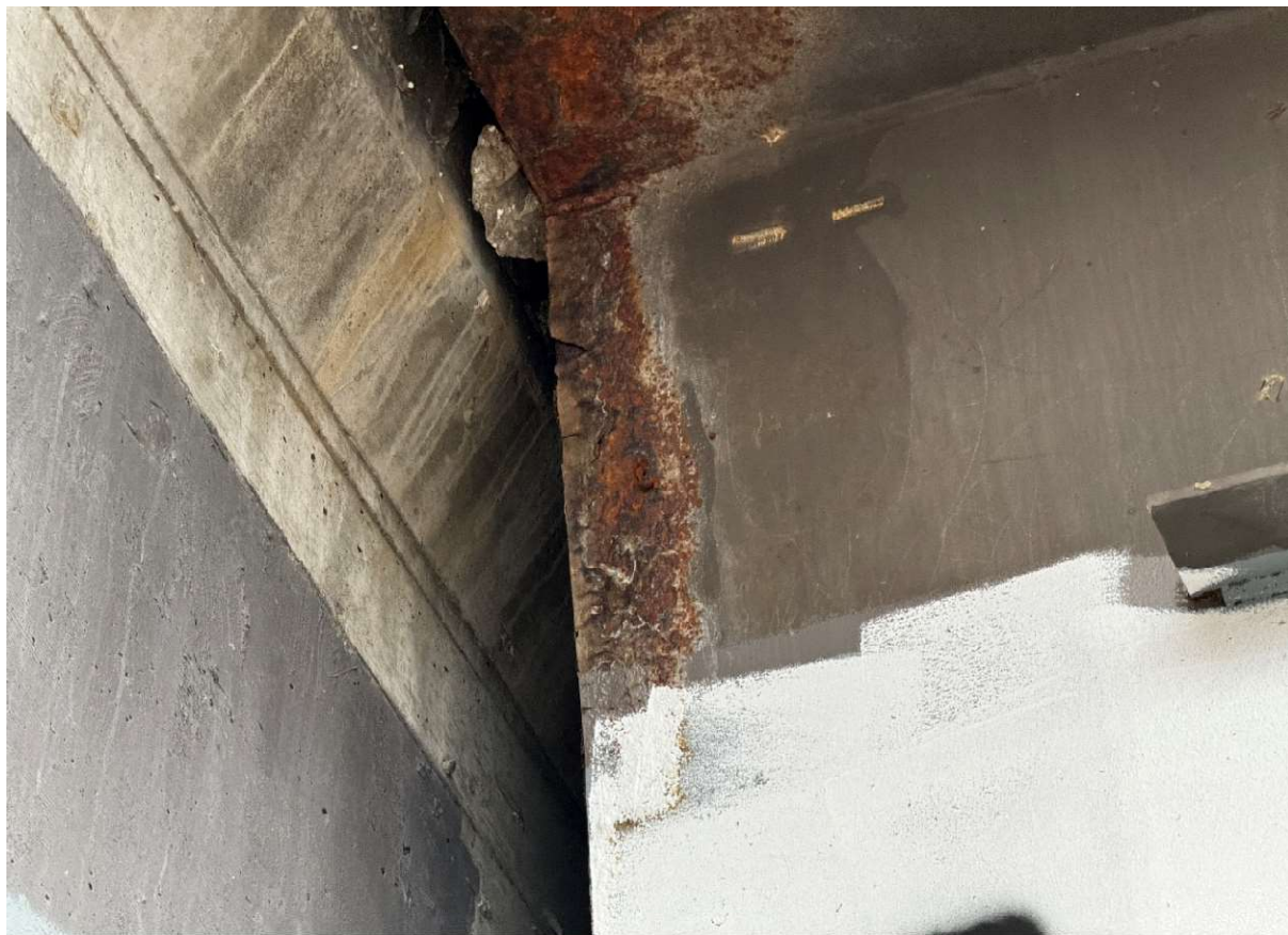
Description of Photo: Girder - Exterior end
