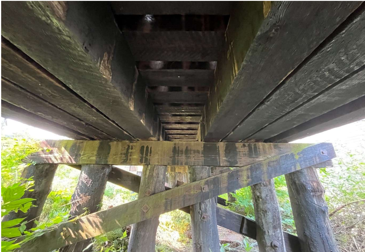
Description of Photo: Stringers
