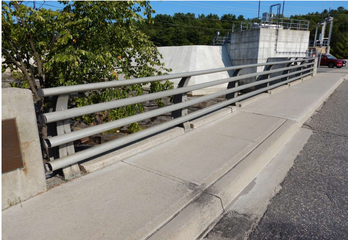
Description of Photo: East Railing System
