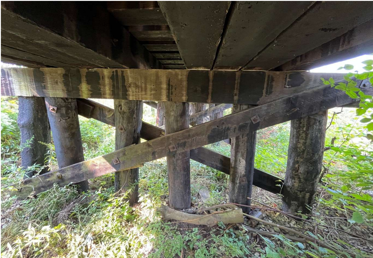
Description of Photo: Pier piles
