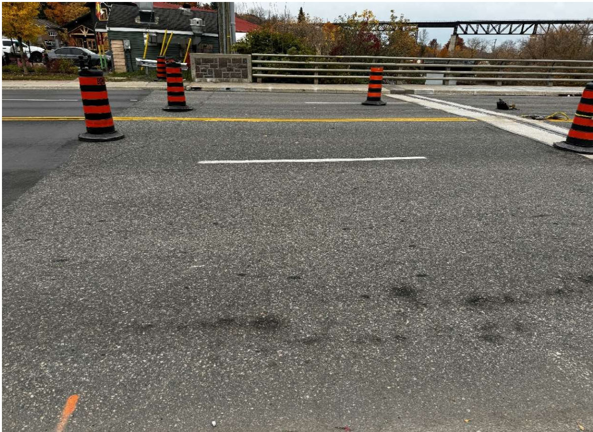
Description of Photo: East approach
