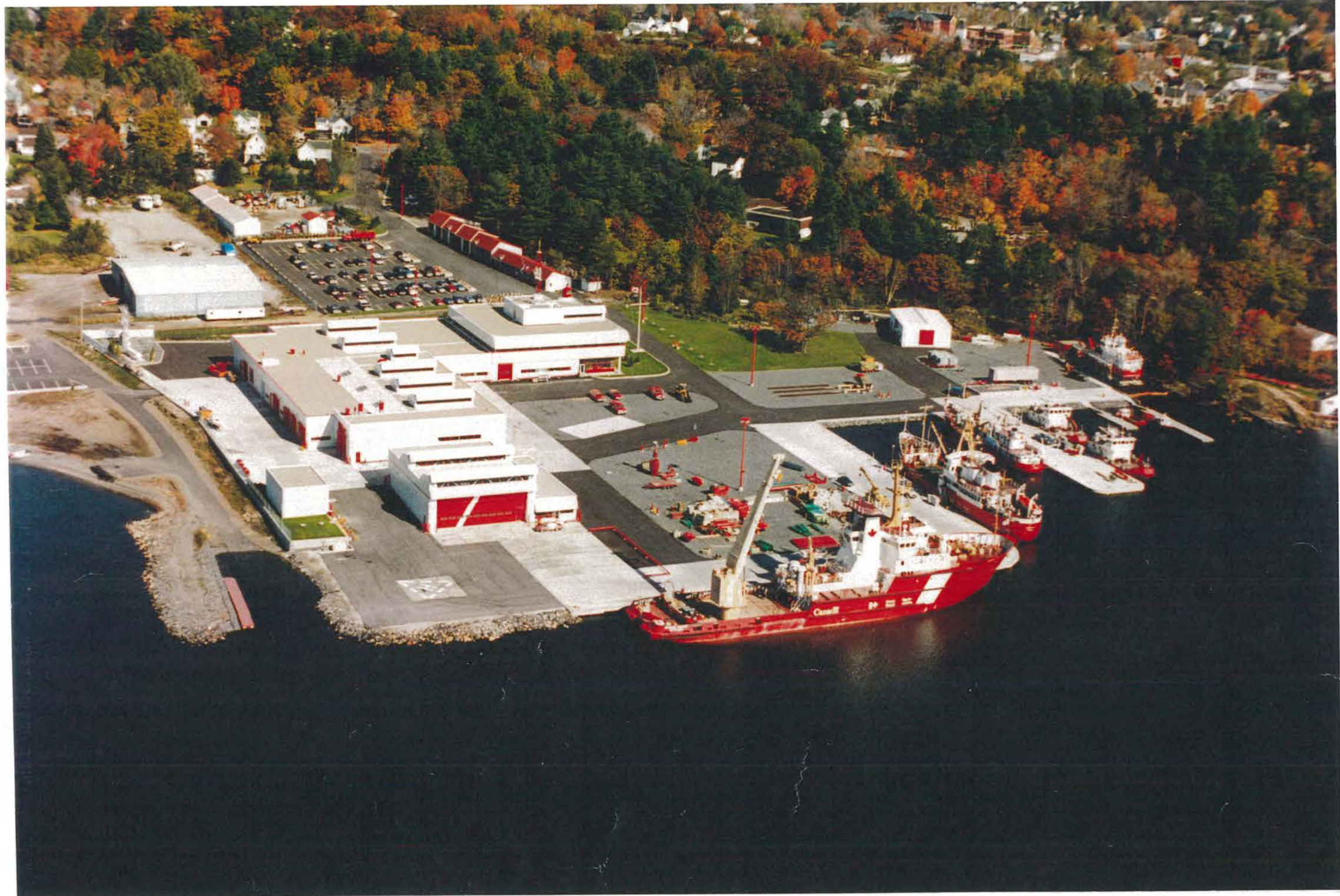
COAST GUARD FACILITY
