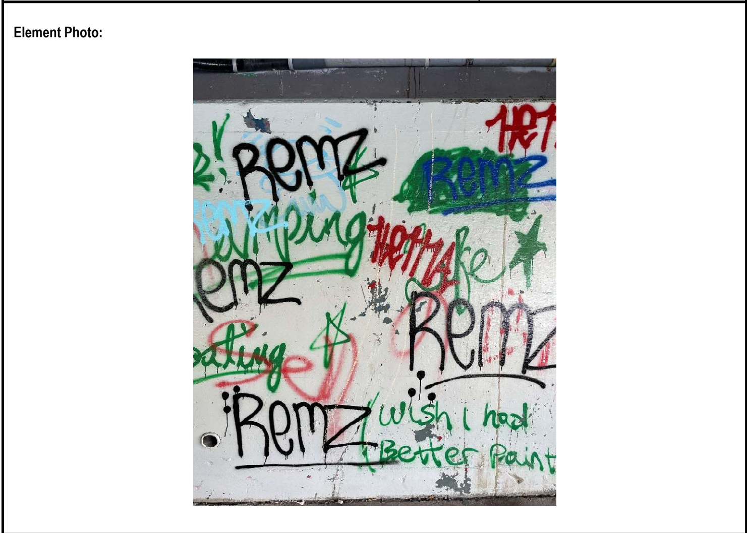
Description of Photo: Abutment Wall
