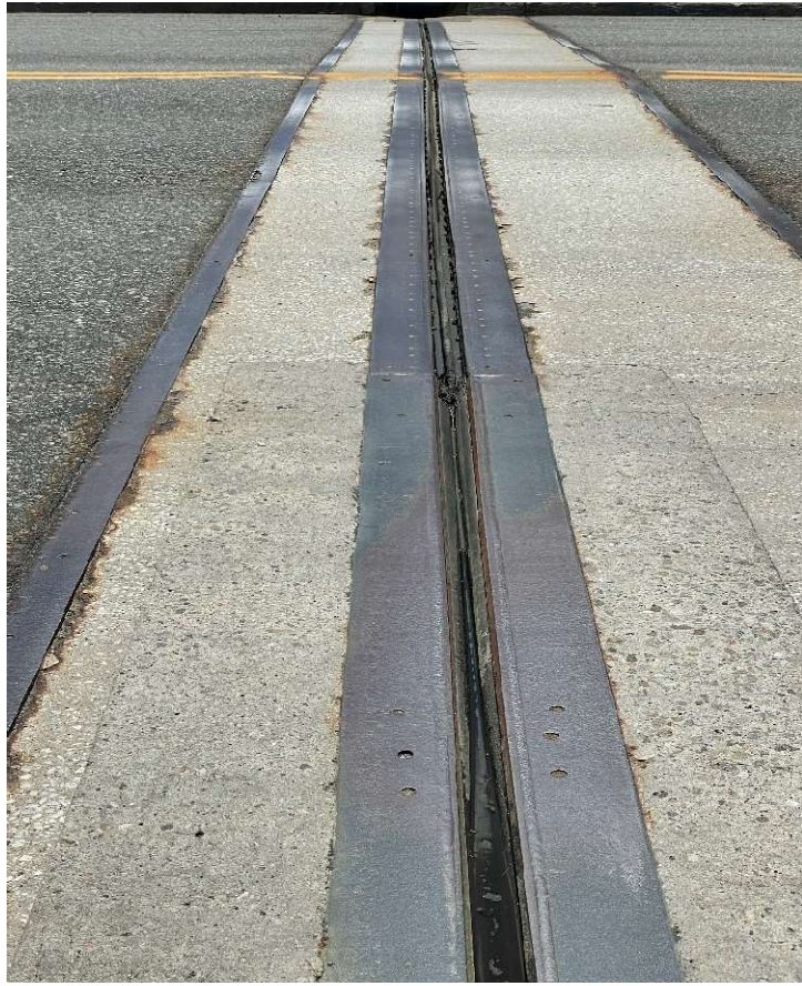
Description of Photo: Joint Armour
