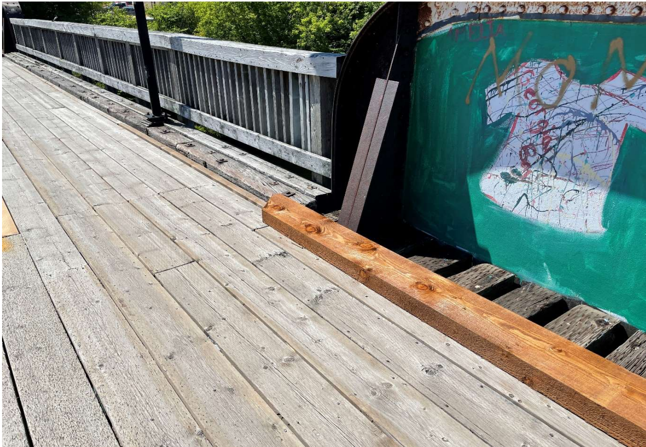
Description of Photo: Curb
