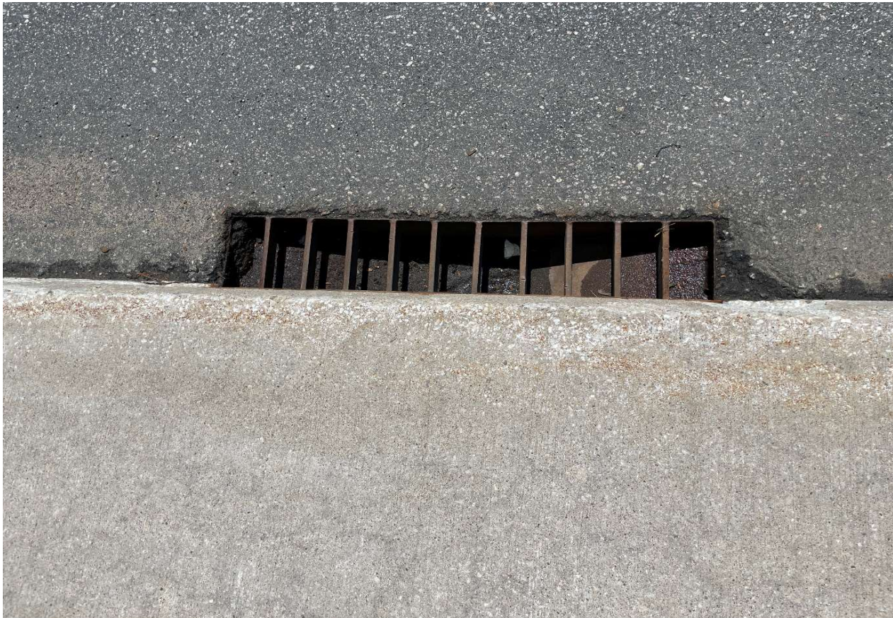
Description of Photo: Drainage
