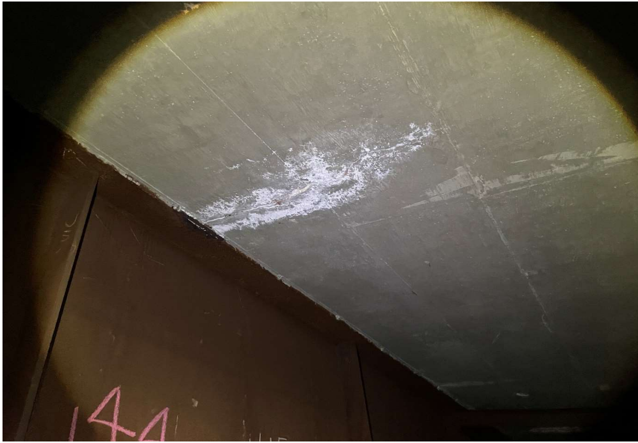
Description of Photo: North Girder Interior Soffit
