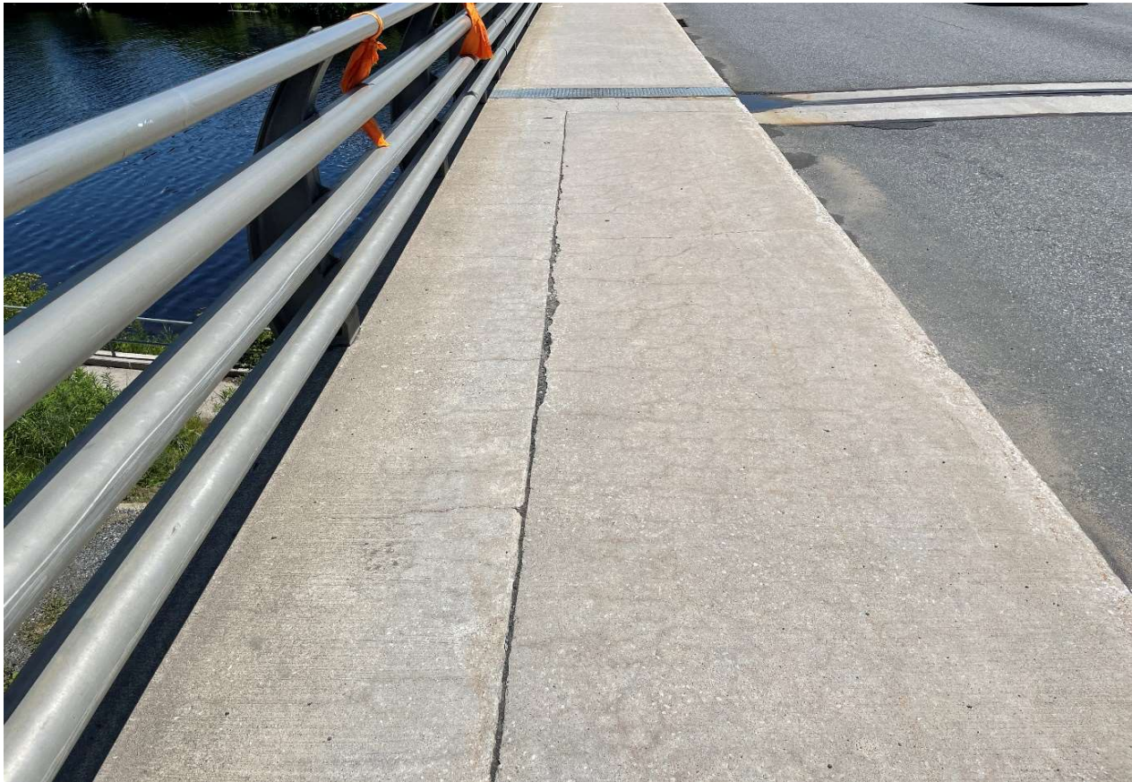
Description of Photo: Approach Sidewalk
