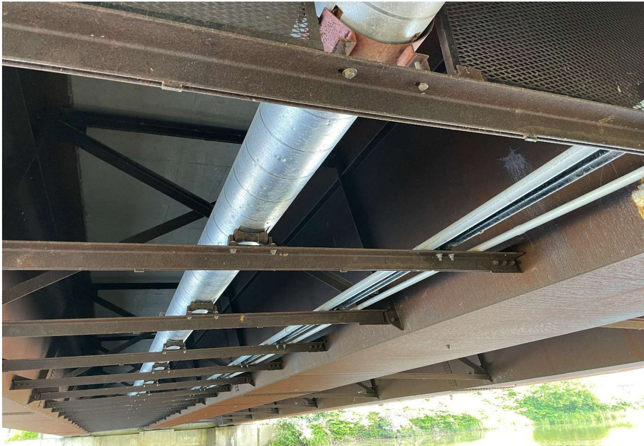
Description of Photo: Utilities
