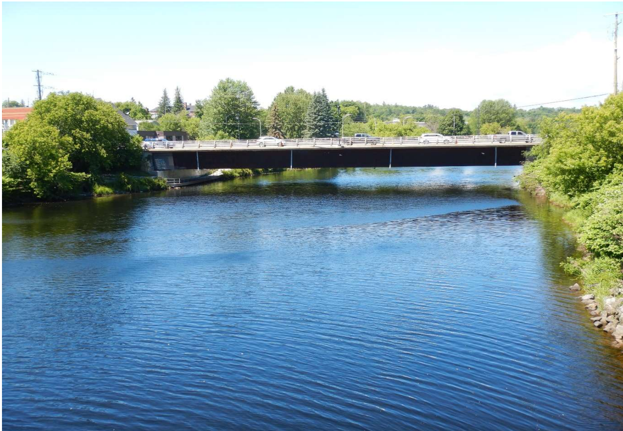
Description of Photo: Embankments
