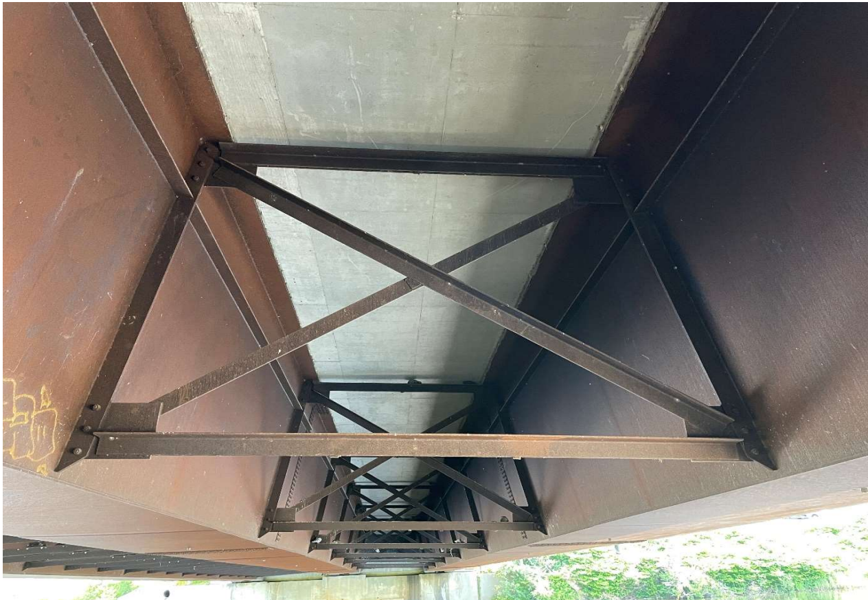
Description of Photo: Diaphragms
