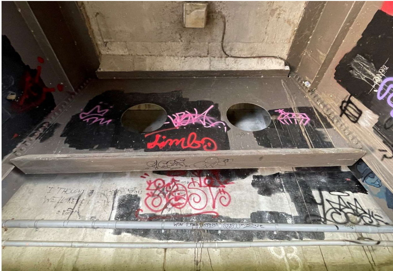
Description of Photo: End Diaphragms
