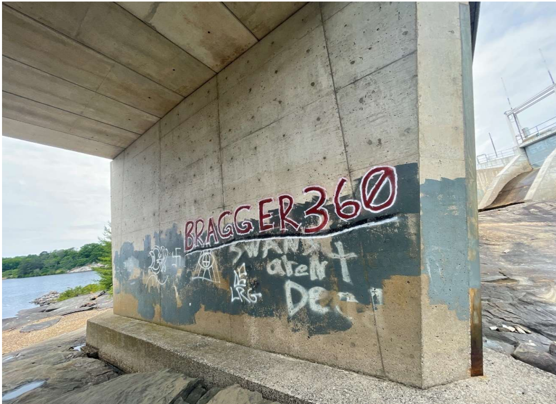
Description of Photo: Pier
