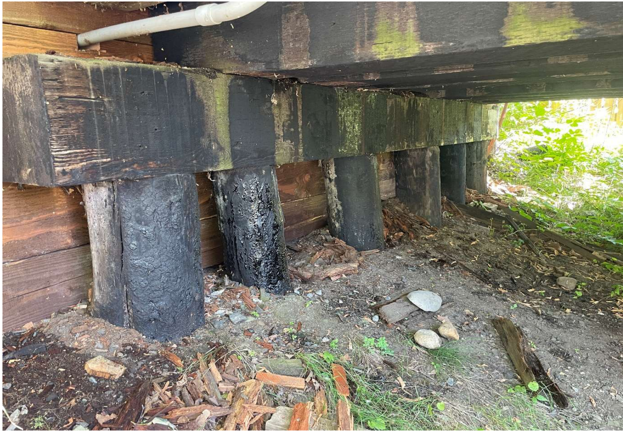
Description of Photo: Piles
