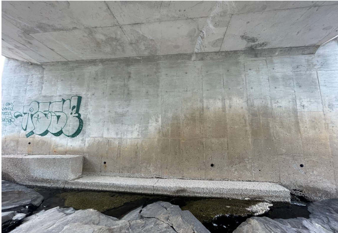
Description of Photo: South Abutment
