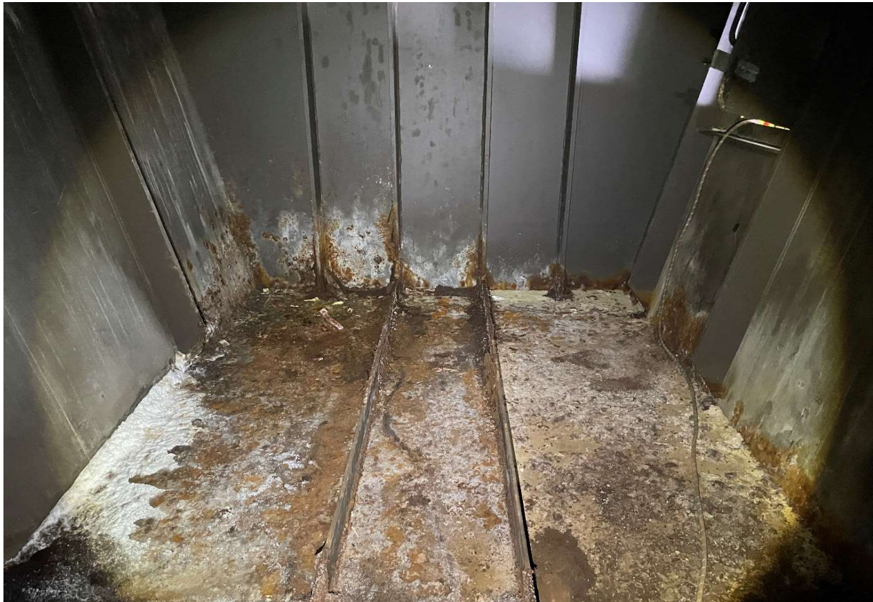
Description of Photo: Girder West End
