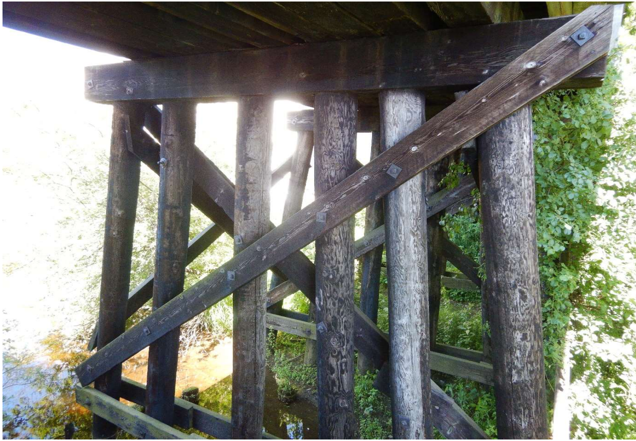
Description of Photo: Bracing
