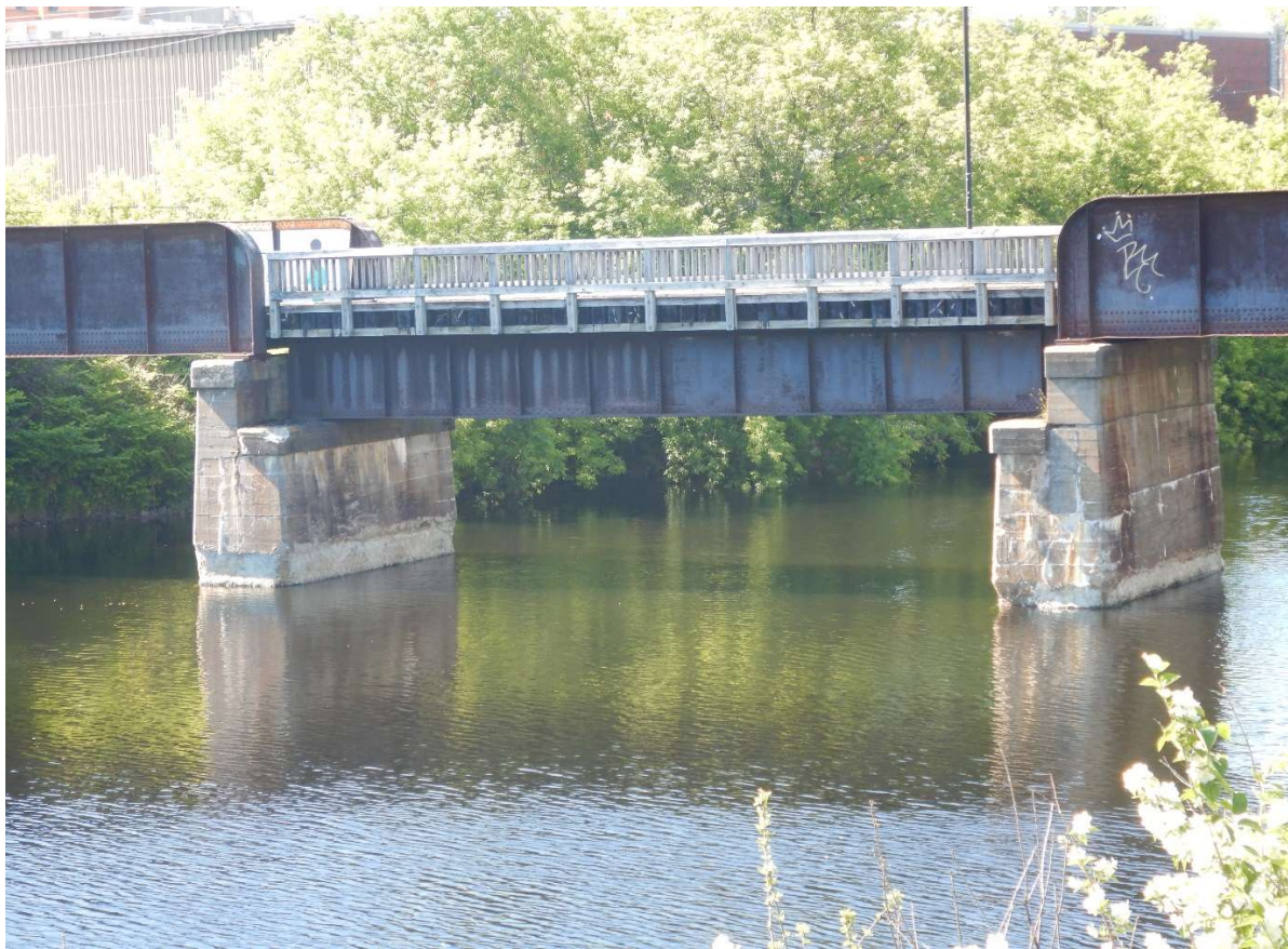
Description of Photo: Elevation View
