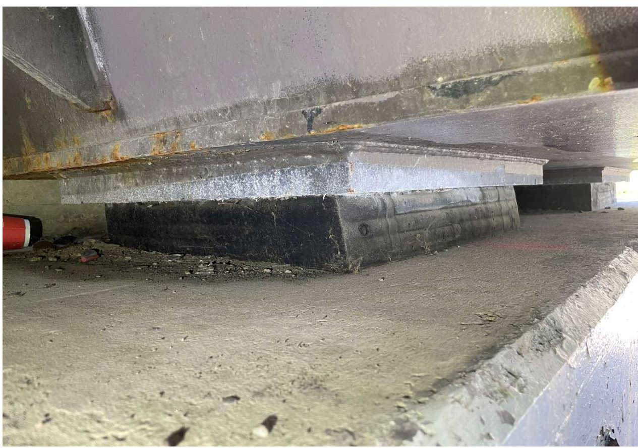
Description of Photo: Bearings
