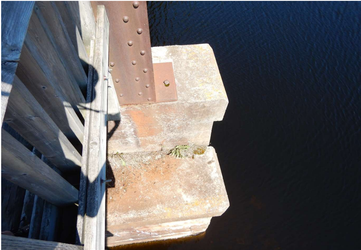
Description of Photo: Pier Bearings
