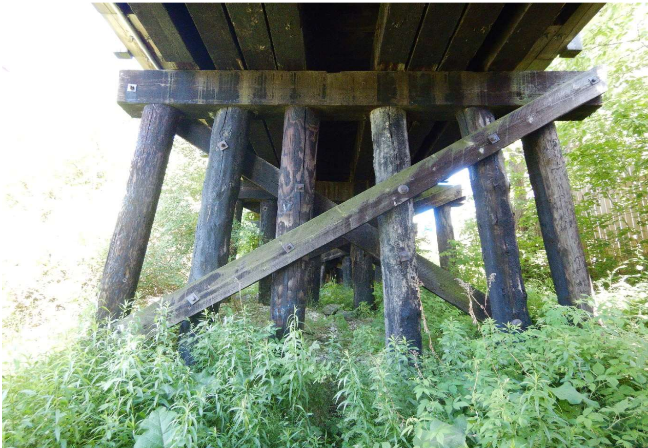
Description of Photo: Piles
