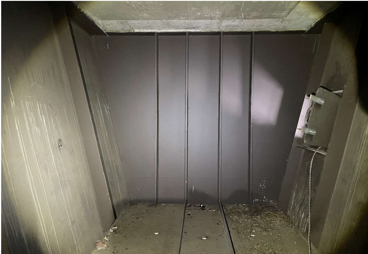
Description of Photo: Center Girder West End
