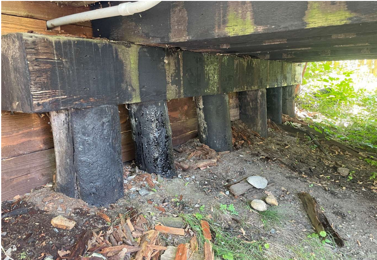
Description of Photo: Pile Cap
