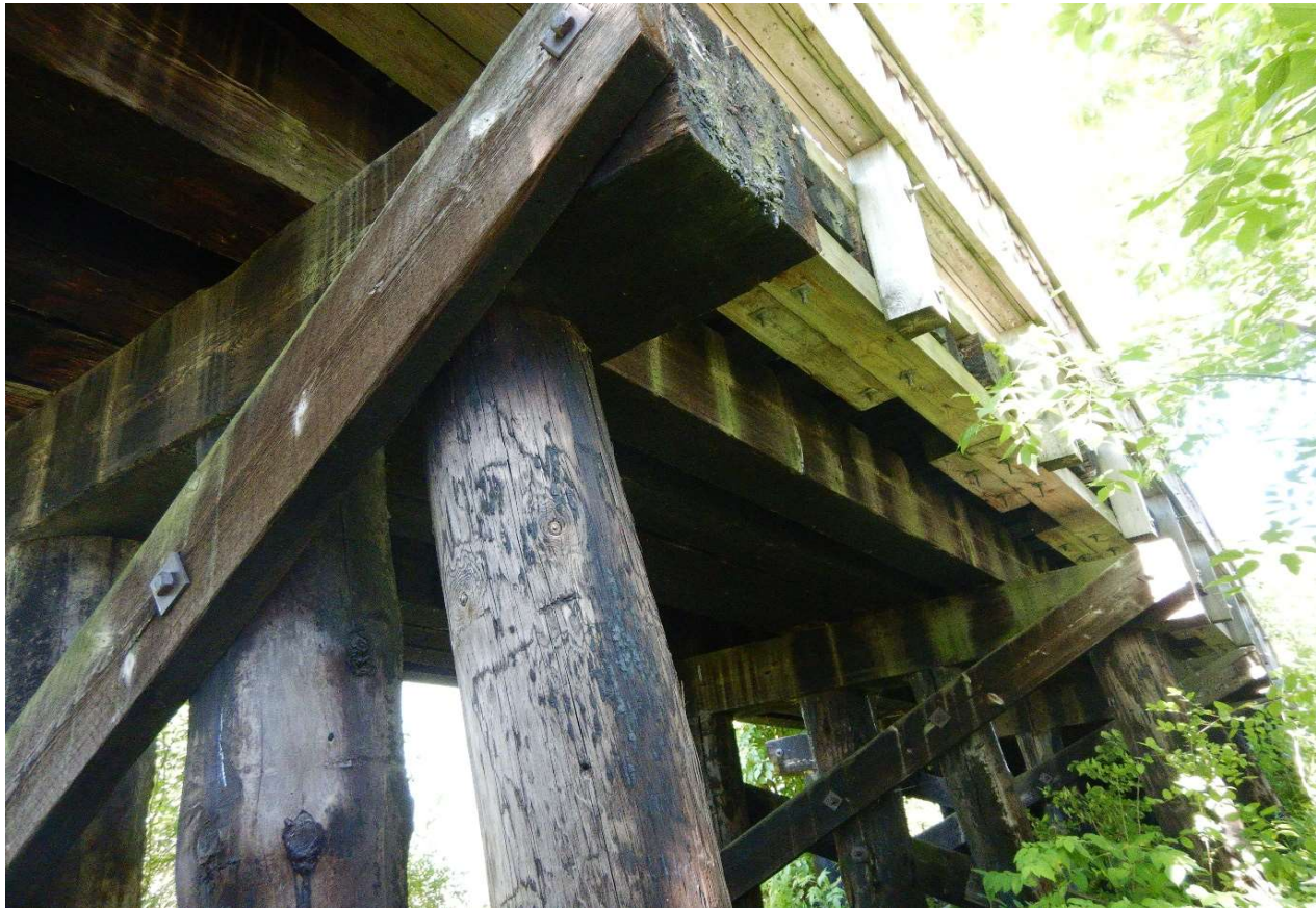
Description of Photo: Pile Cap
