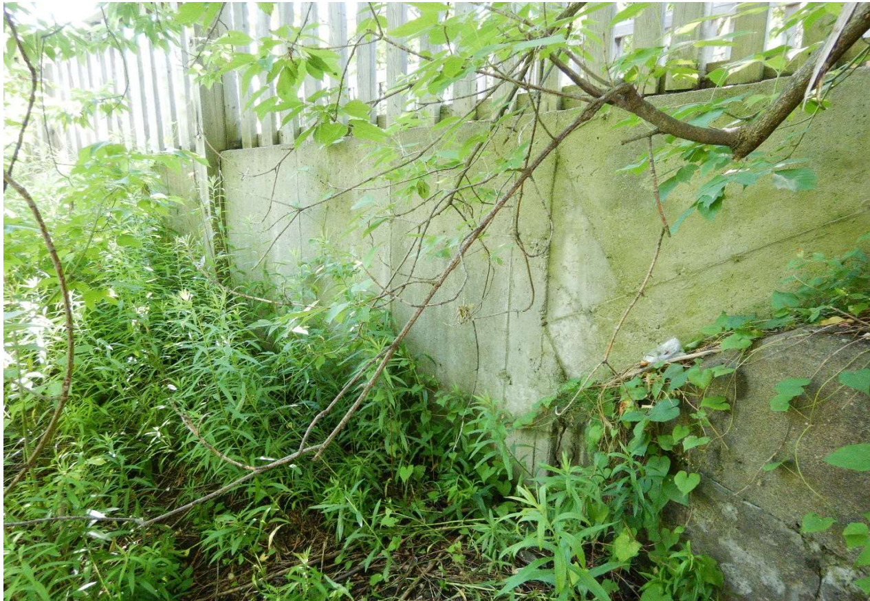
Description of Photo: Retaining Wall
