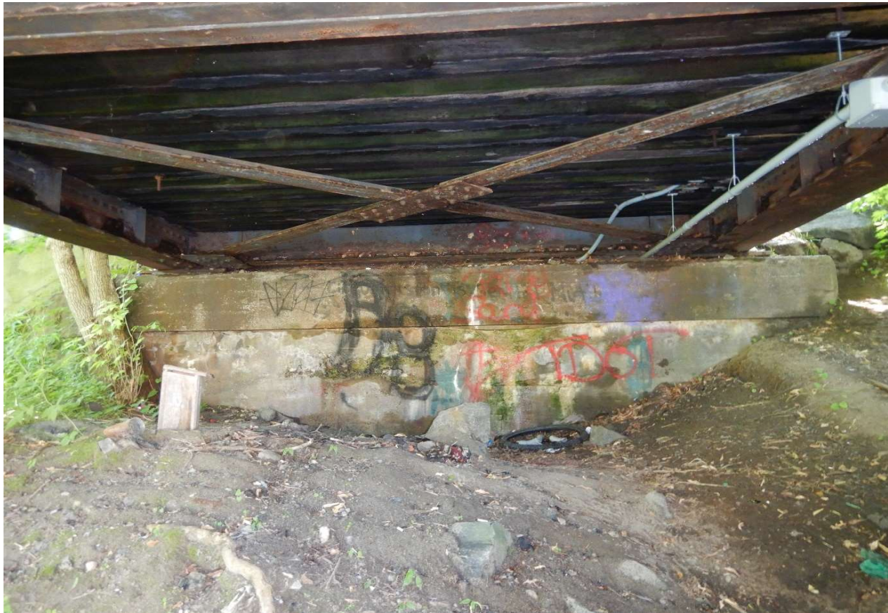
Description of Photo: West Abutment
