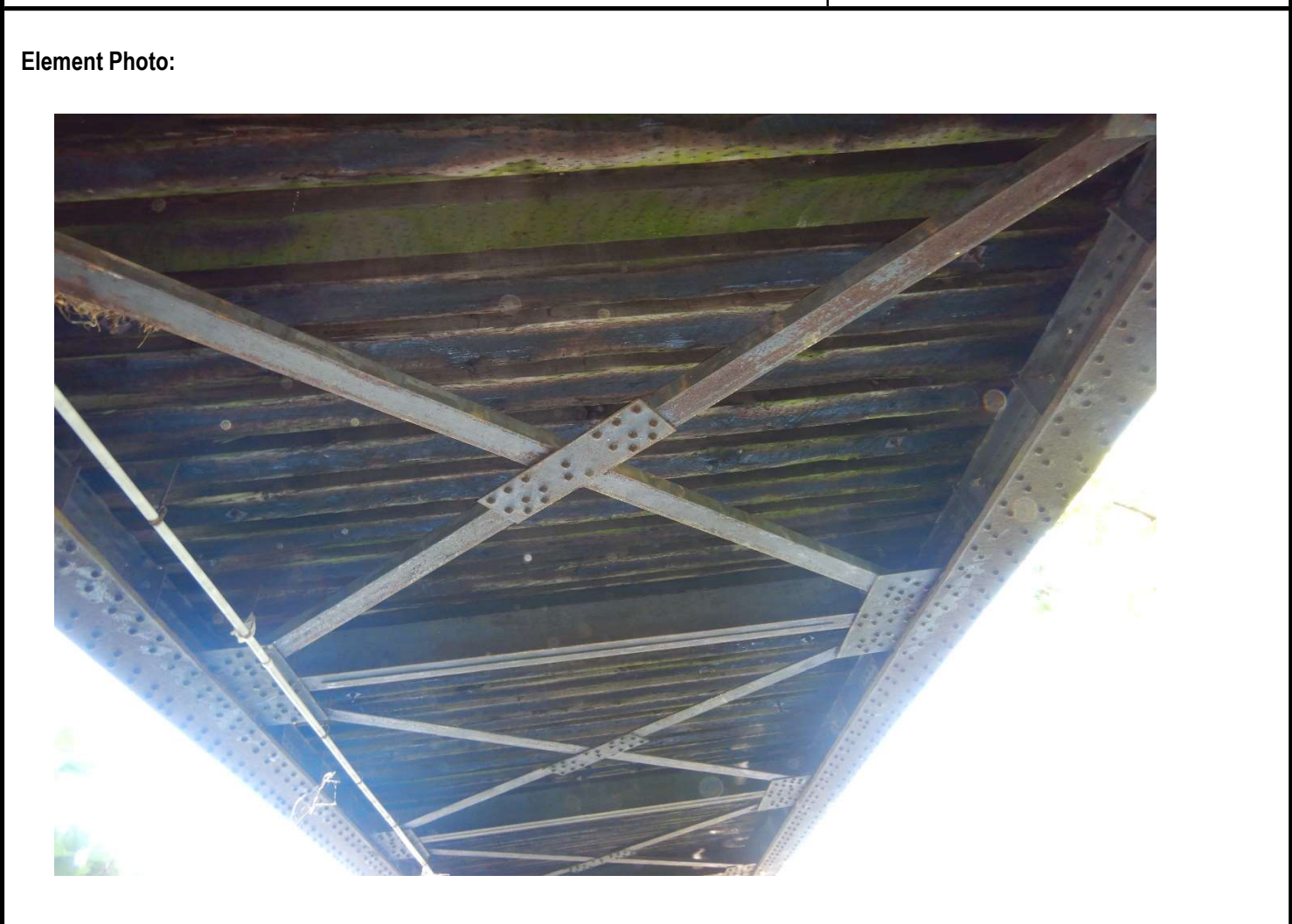
Description of Photo: Floor Beams
