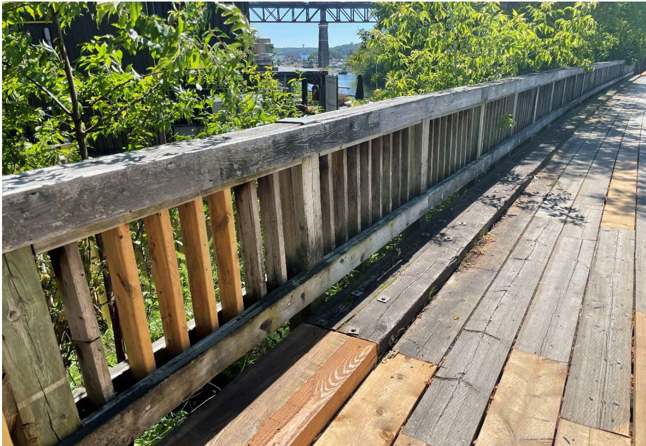
Description of Photo: Railing System
