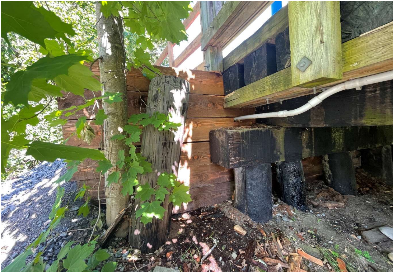
Description of Photo: East Abutment
