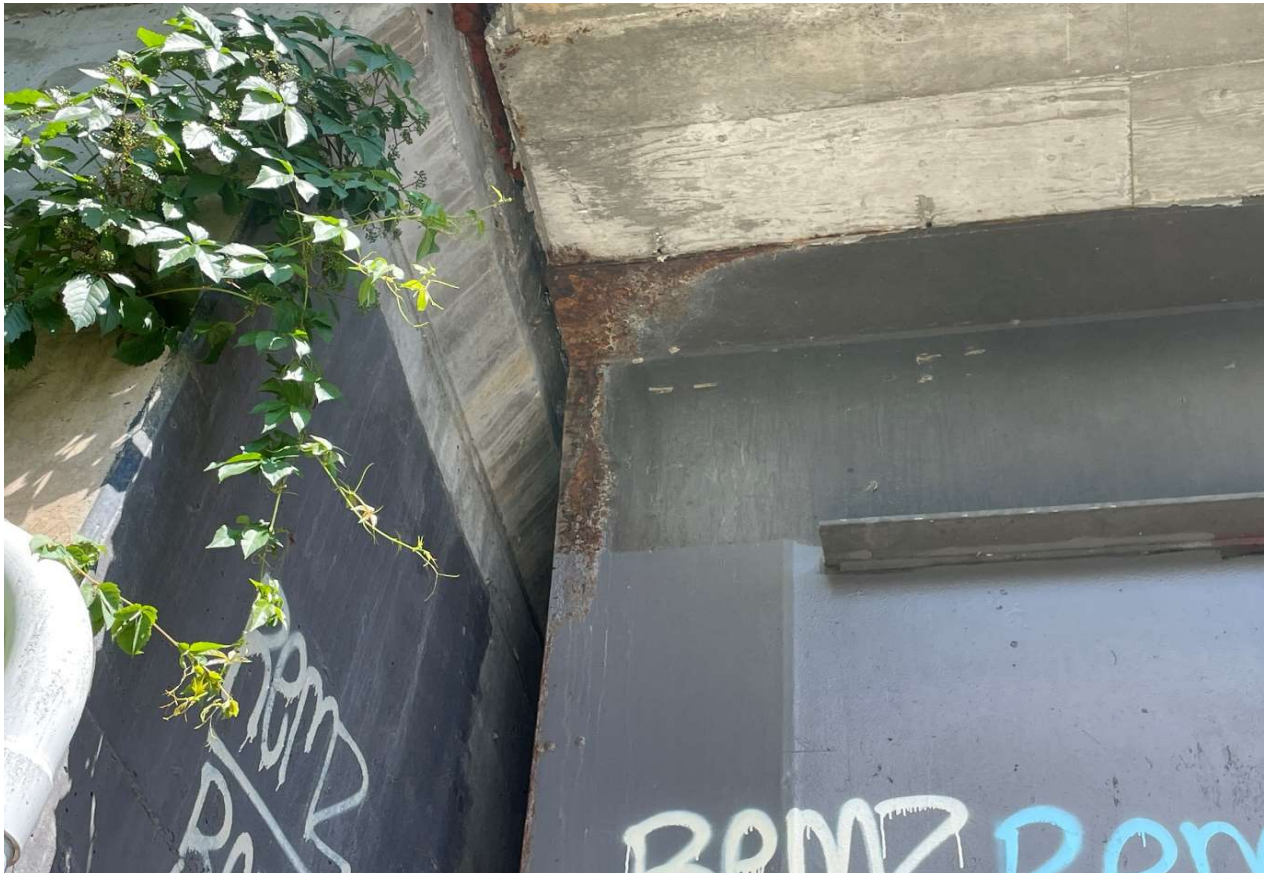
Description of Photo: Girder - Exterior End
