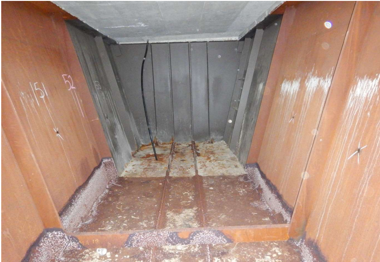
Description of Photo: East Girder End
