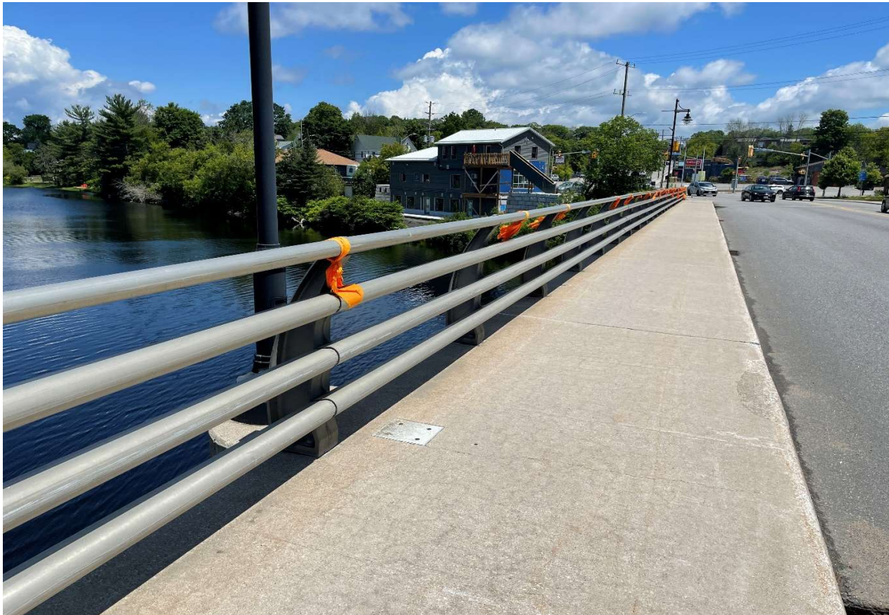
Description of Photo: Railing System
