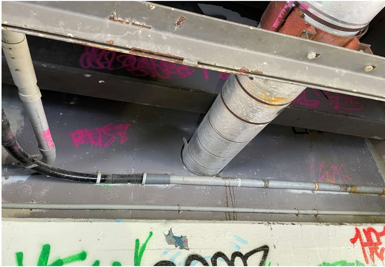
Description of Photo: Ballast Wall
