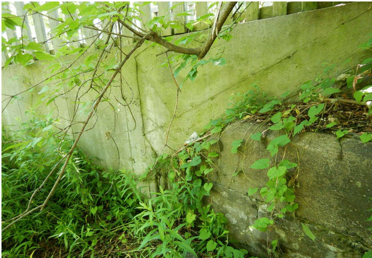
Description of Photo: Wingwall
