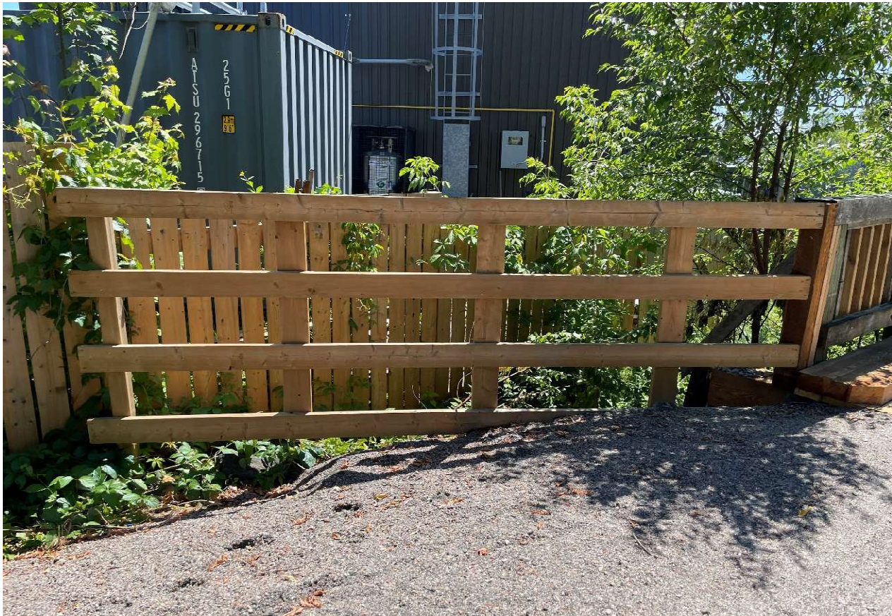
Description of Photo: Approach Barrier
