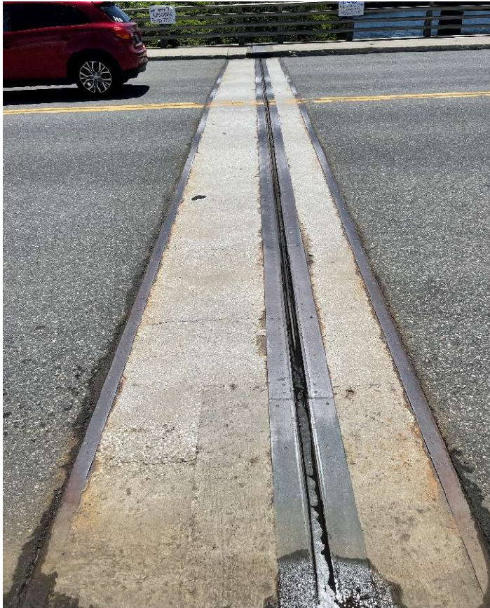
Description of Photo: Joint Concrete End Dam
