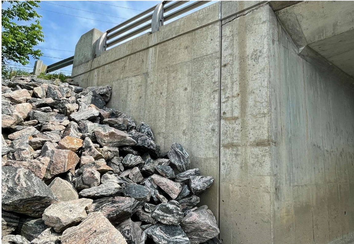
Description of Photo: Northwest wingwall
