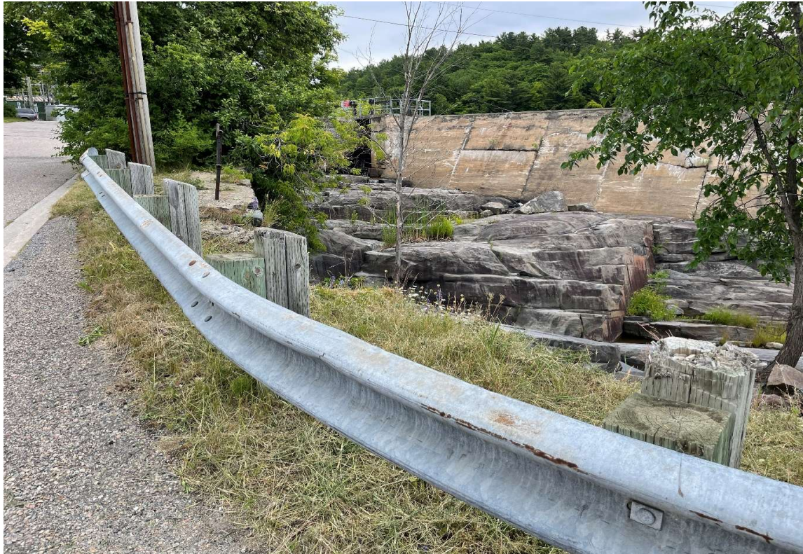
Description of Photo: Northeast approach barrier
