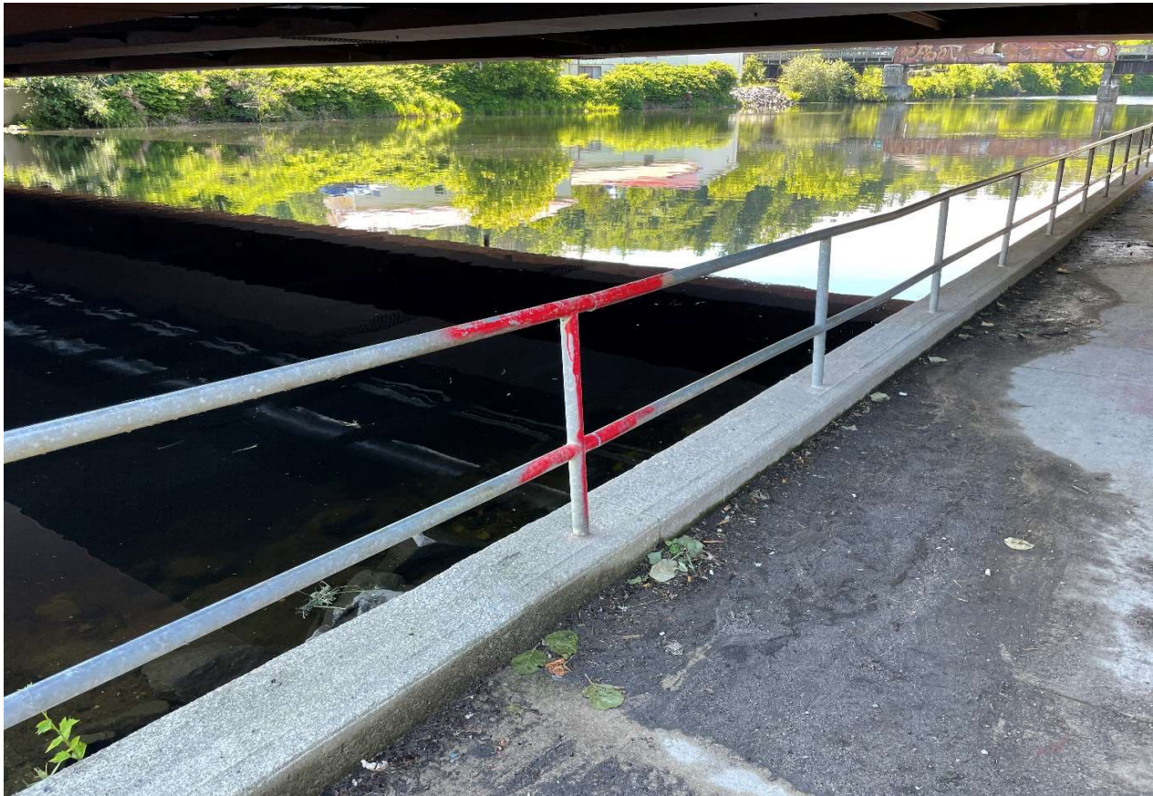
Description of Photo: Retaining Wall Railing
