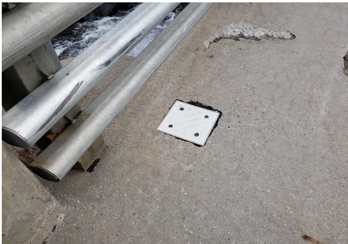
Description of Photo: Photo 24 - Railing
