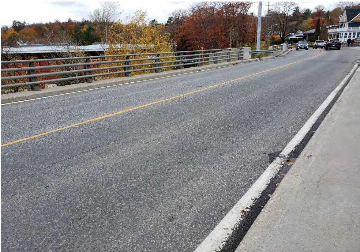
Description of Photo: Photo 16 - Deck Top
