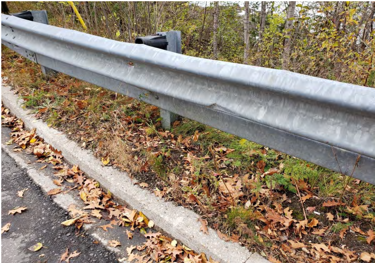
Description of Photo: Photo 6 - Approach Curb
