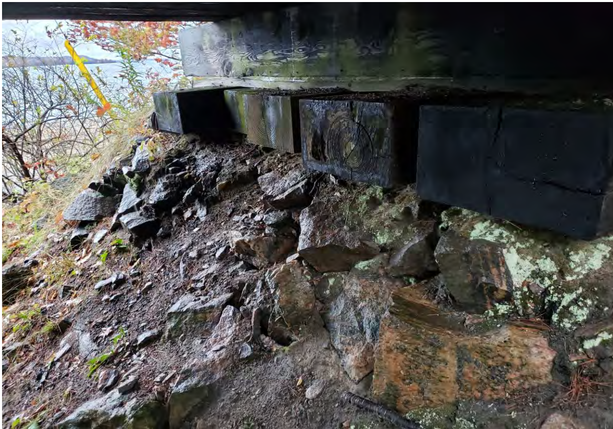
Description of Photo: Photo 34 - Slope Protection.jpg
