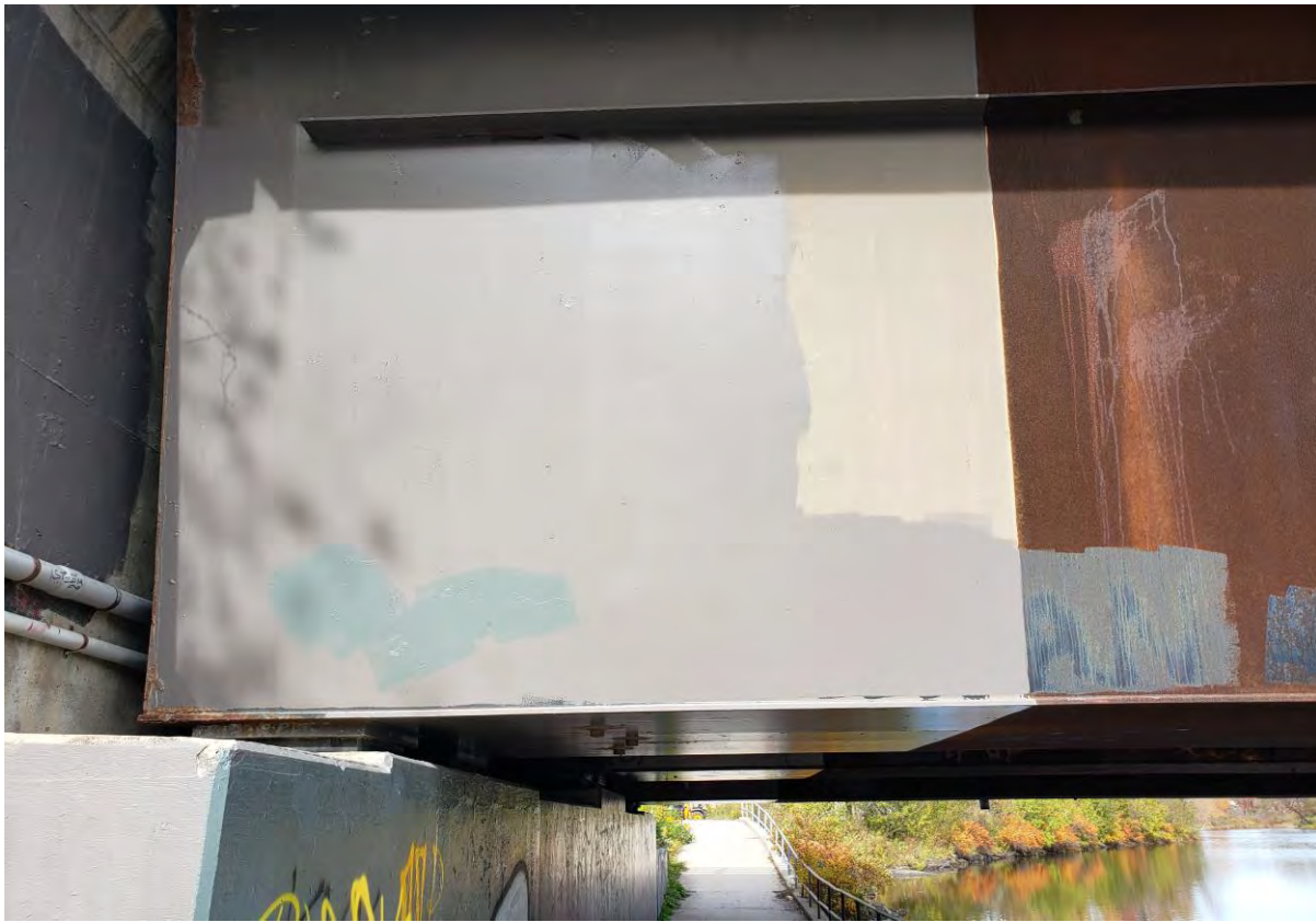
Description of Photo: Photo 34 - Girder Exterior End.jpg
