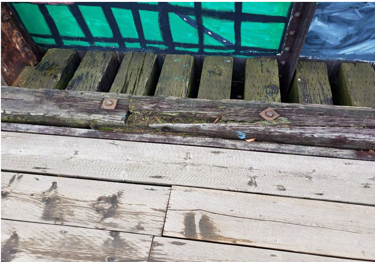
Description of Photo: Photo 7 - Deck Top
