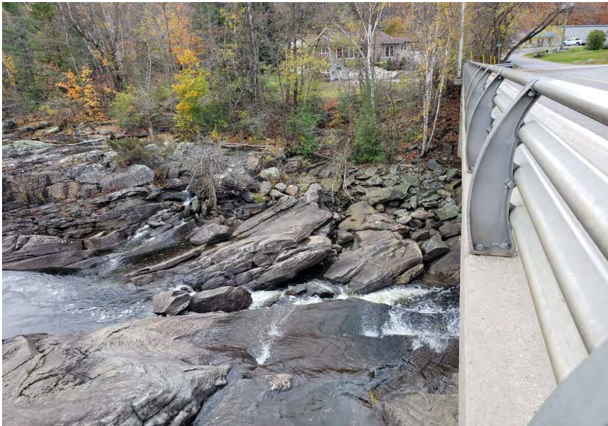
Description of Photo: Photo 36 - Embankment
