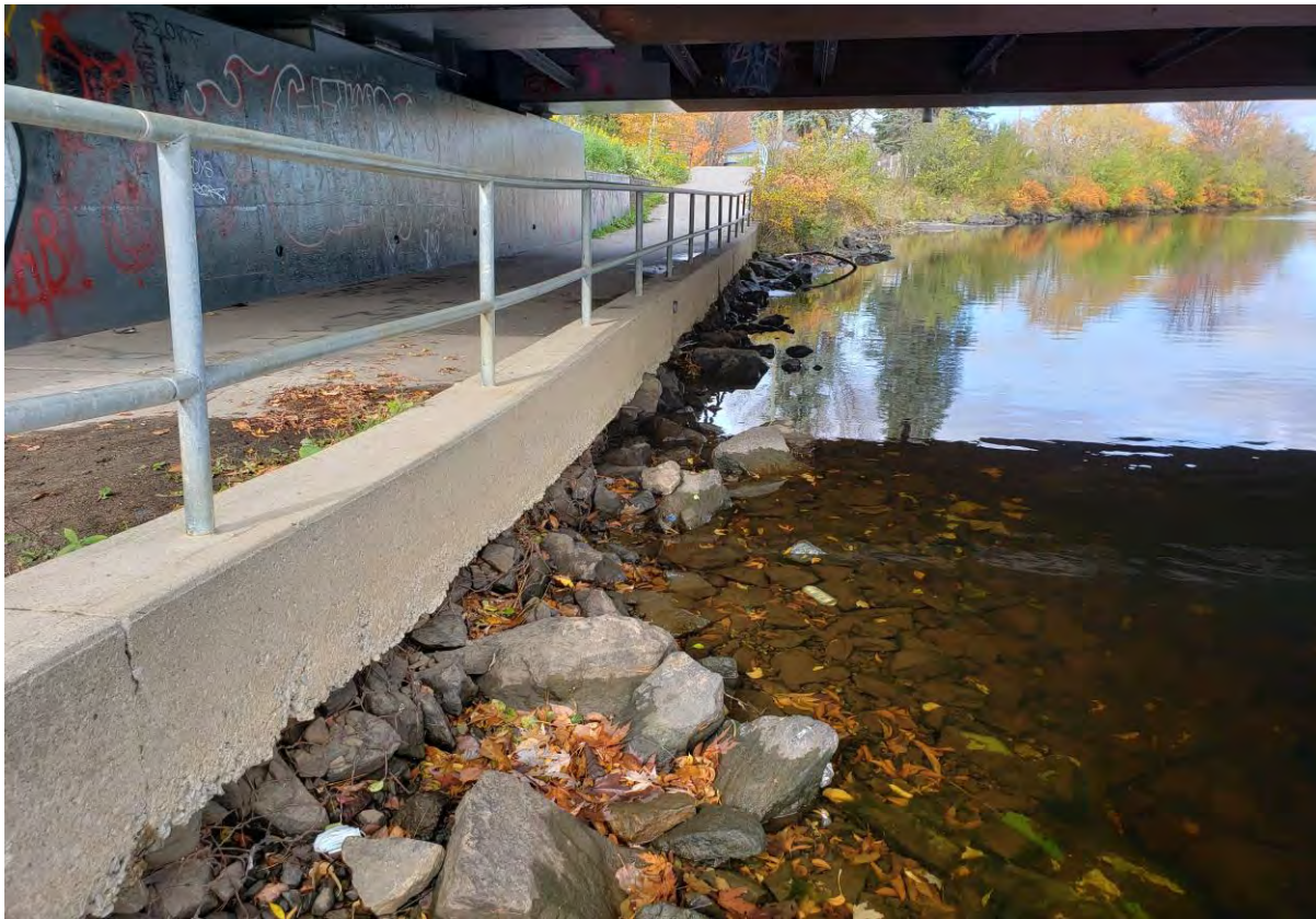
Description of Photo: Photo 66 - Foundation.jpg
