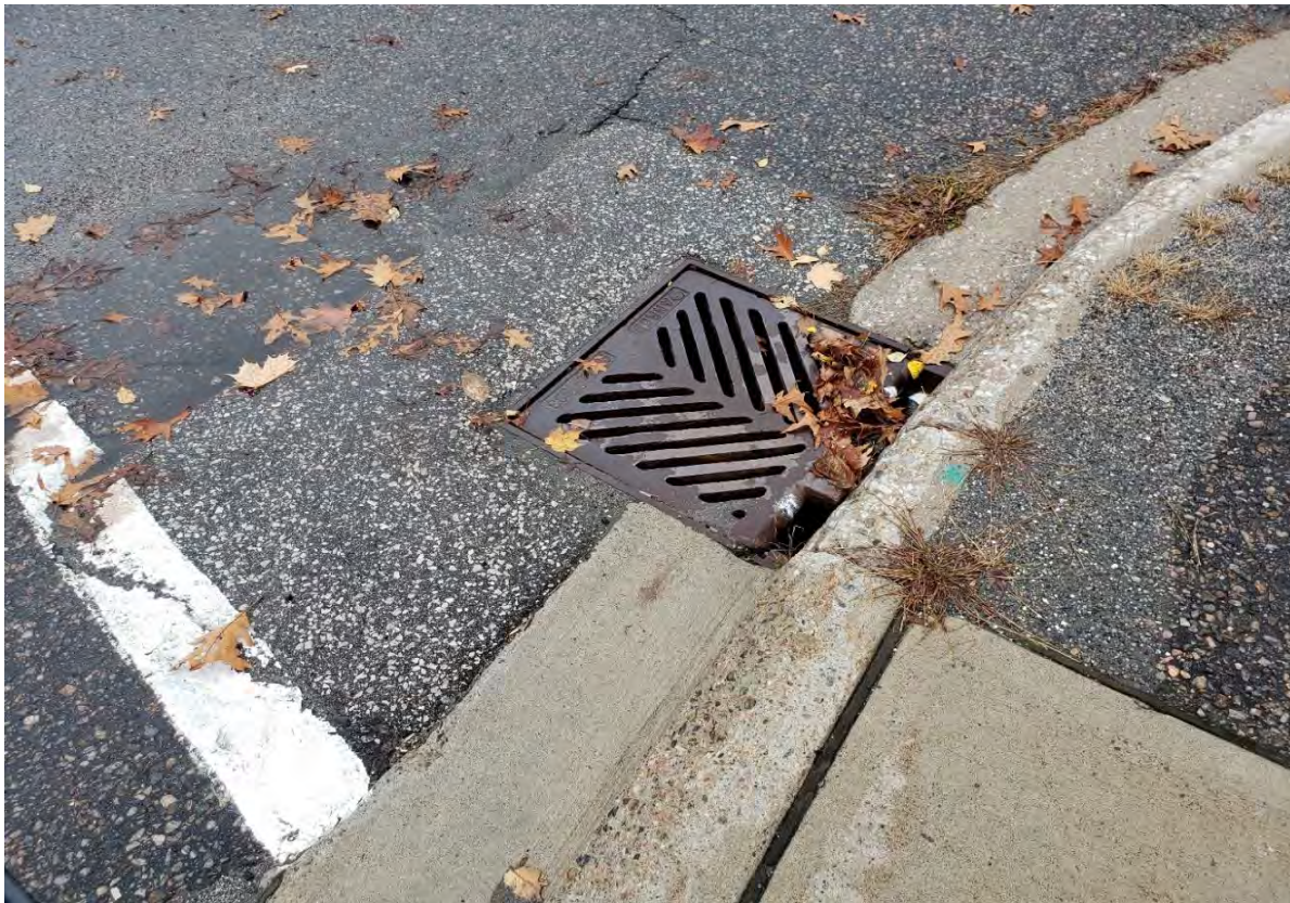
Description of Photo: Photo 6 - Approach Catchbasin
