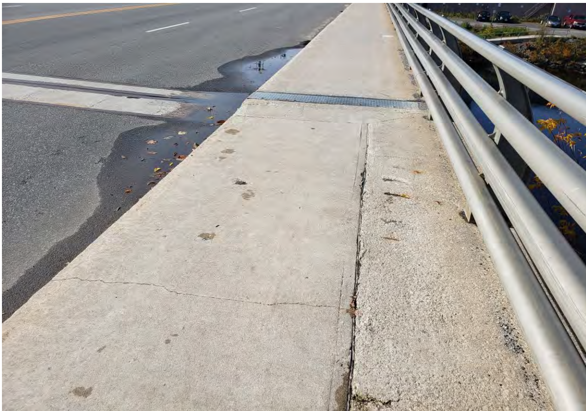
Description of Photo: Photo 19 - Sidewalk.jpg
