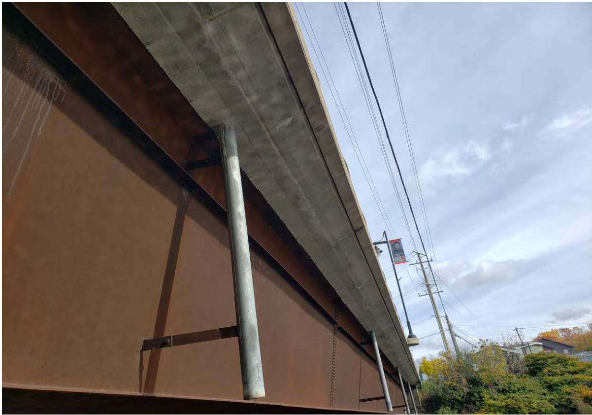
Description of Photo: Photo 60 - Exterior Soffit.jpg
