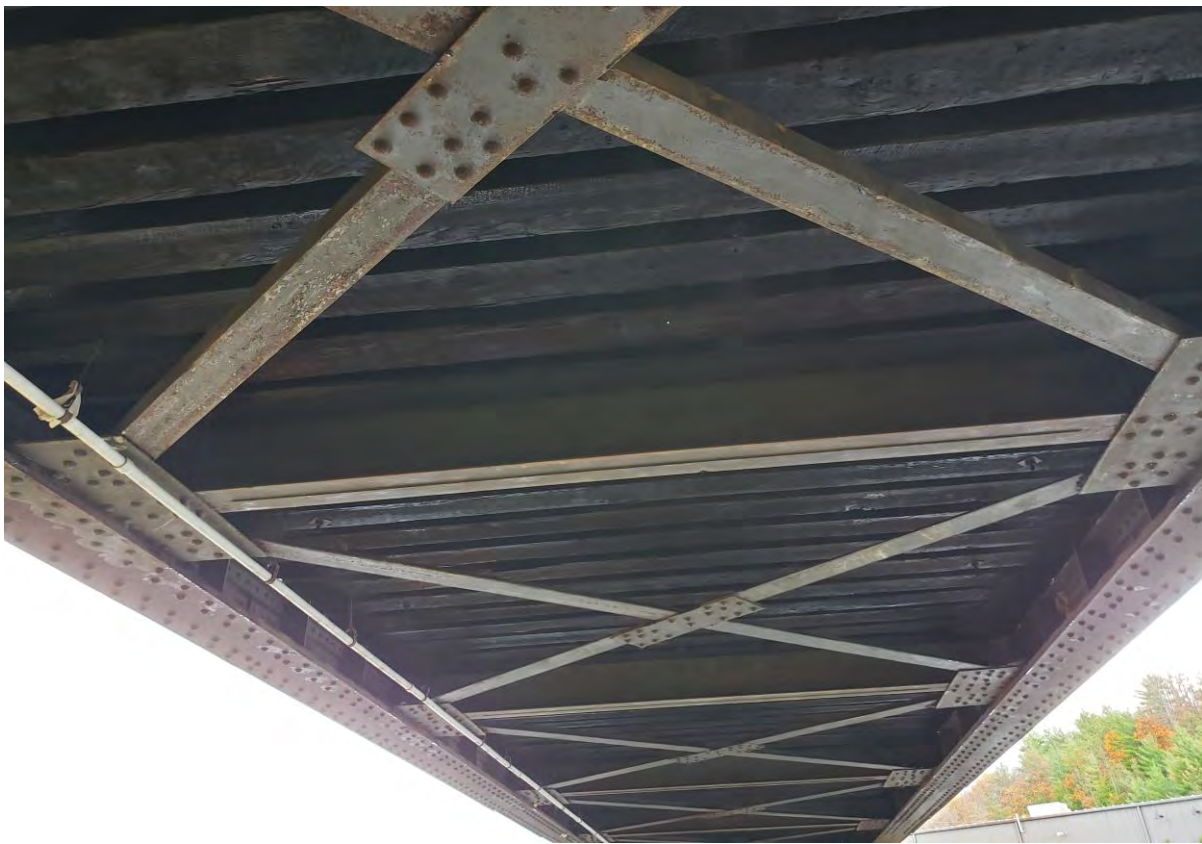
Description of Photo: Photo 53 - Girders.jpg
