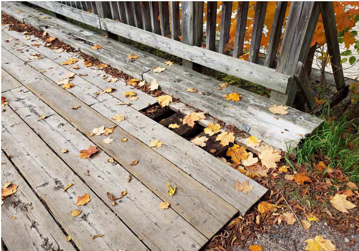
Description of Photo: Photo 4 - Wearing Surface.jpg
