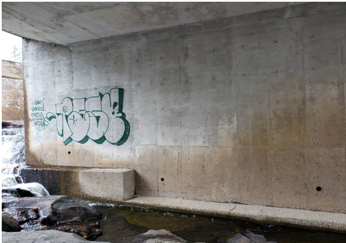
Description of Photo: Photo 26 - Abutment Wall
