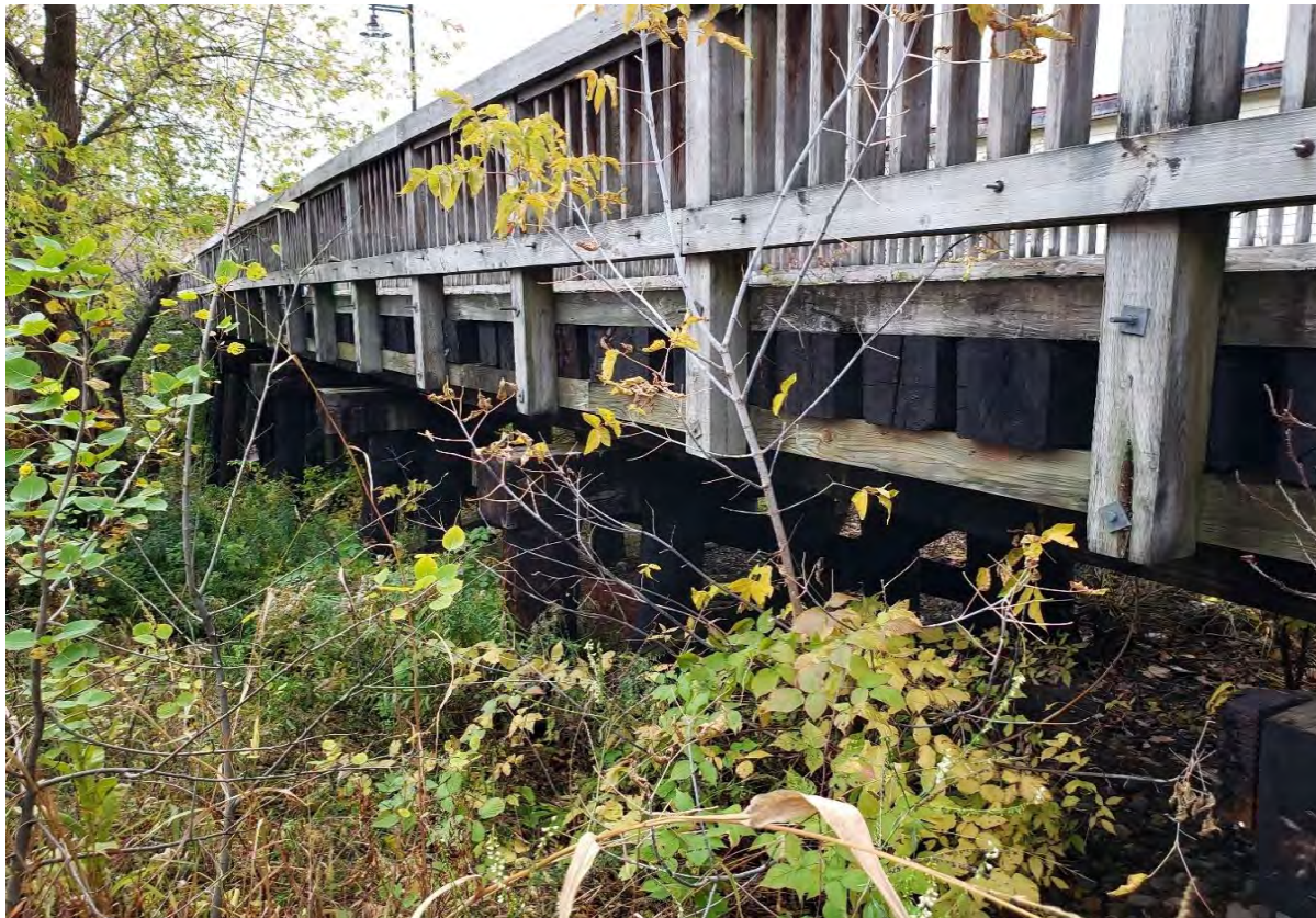
Description of Photo: Photo 36 - Stringers
