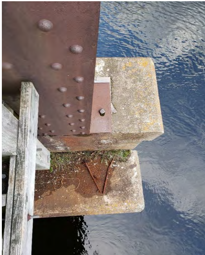
Description of Photo: Photo 44 - Pier Bearings
