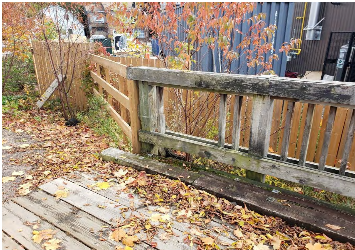
Description of Photo: Photo 12 - Railing
