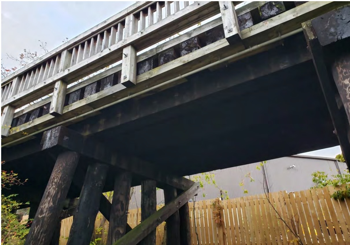
Description of Photo: Photo 35 - Timber Beams
