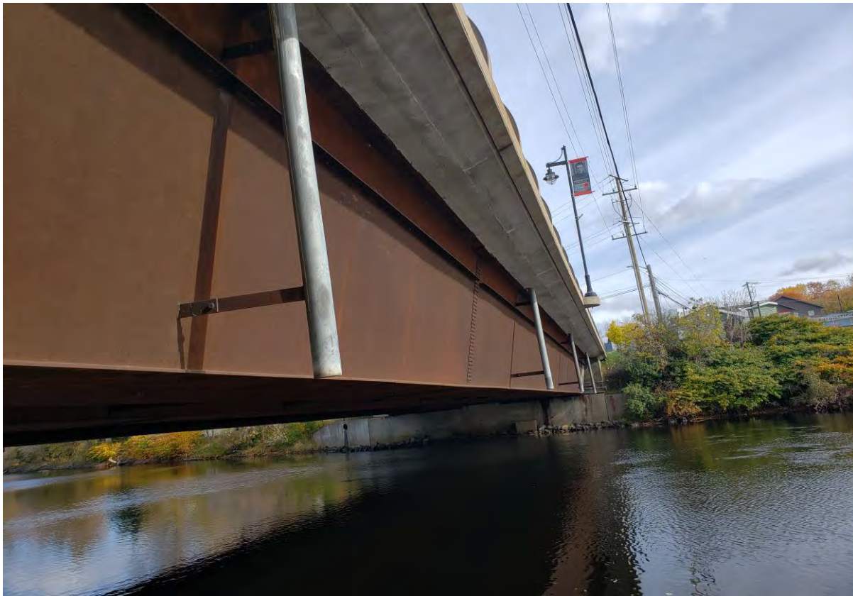
Description of Photo: Photo 36 - Girder Exterior Mid.jpg
