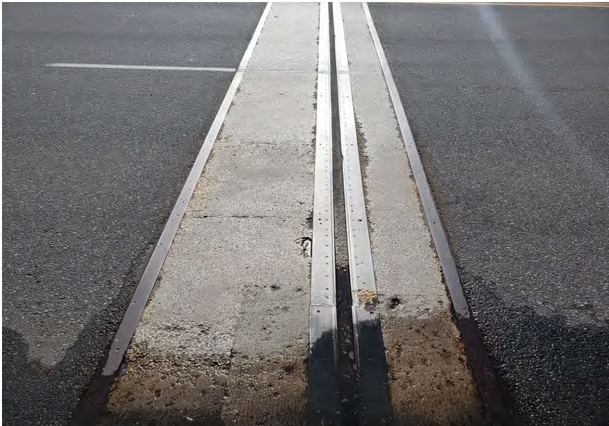
Description of Photo: Photo 16 - Joint End Dam.jpg
