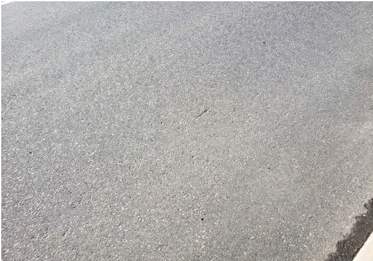
Description of Photo: Photo 14 - Wearing Surface.jpg
