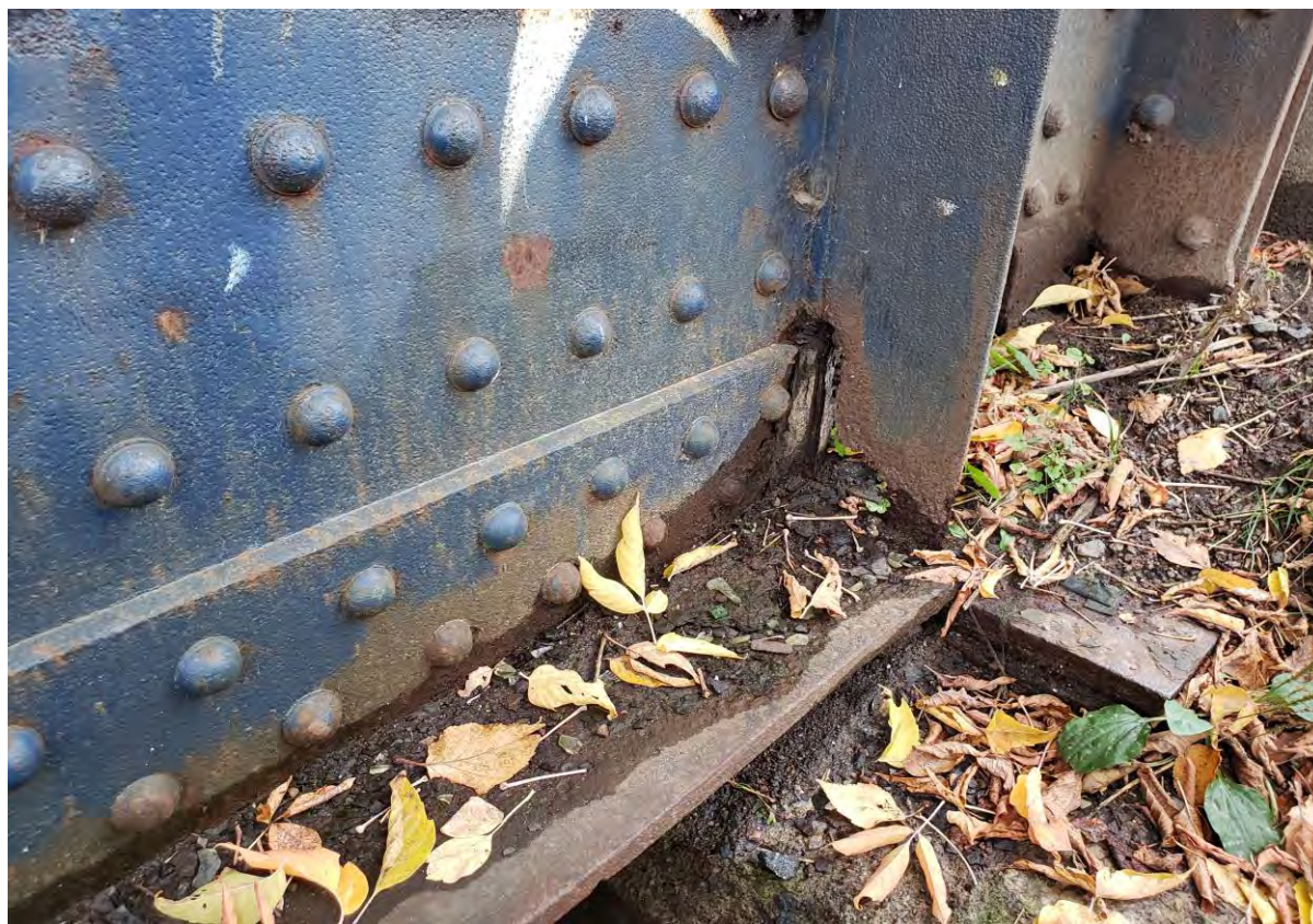
Description of Photo: Photo 18 - Coatings.jpg
