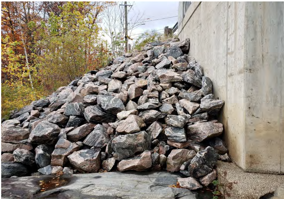
Description of Photo: Photo 35 - Slope Protection
