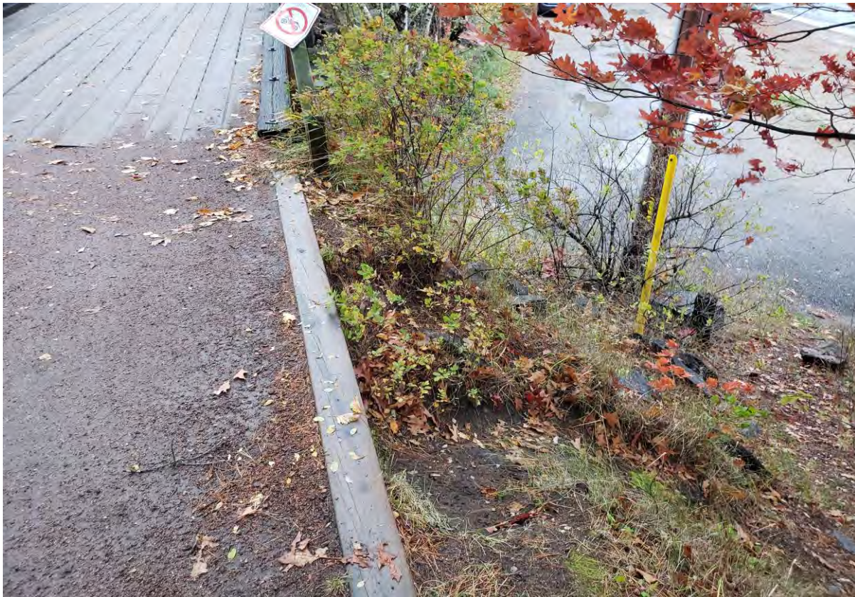
Description of Photo: Photo 31 - Embankment.jpg
