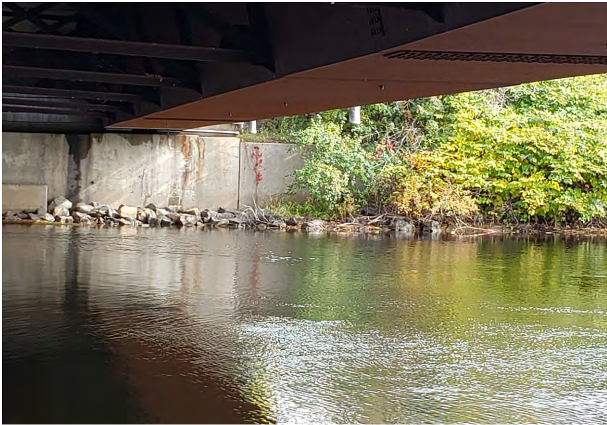
Description of Photo: Photo 68 - Embankment.jpg
