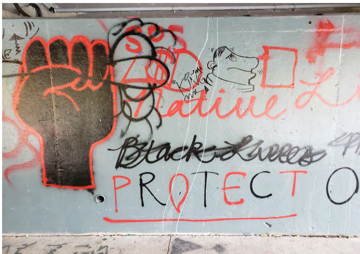
Description of Photo: Photo 48 - Abutment Wall.jpg
