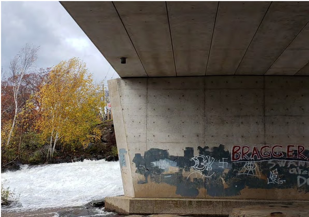
Description of Photo: Photo 42 - Pier Bearings
