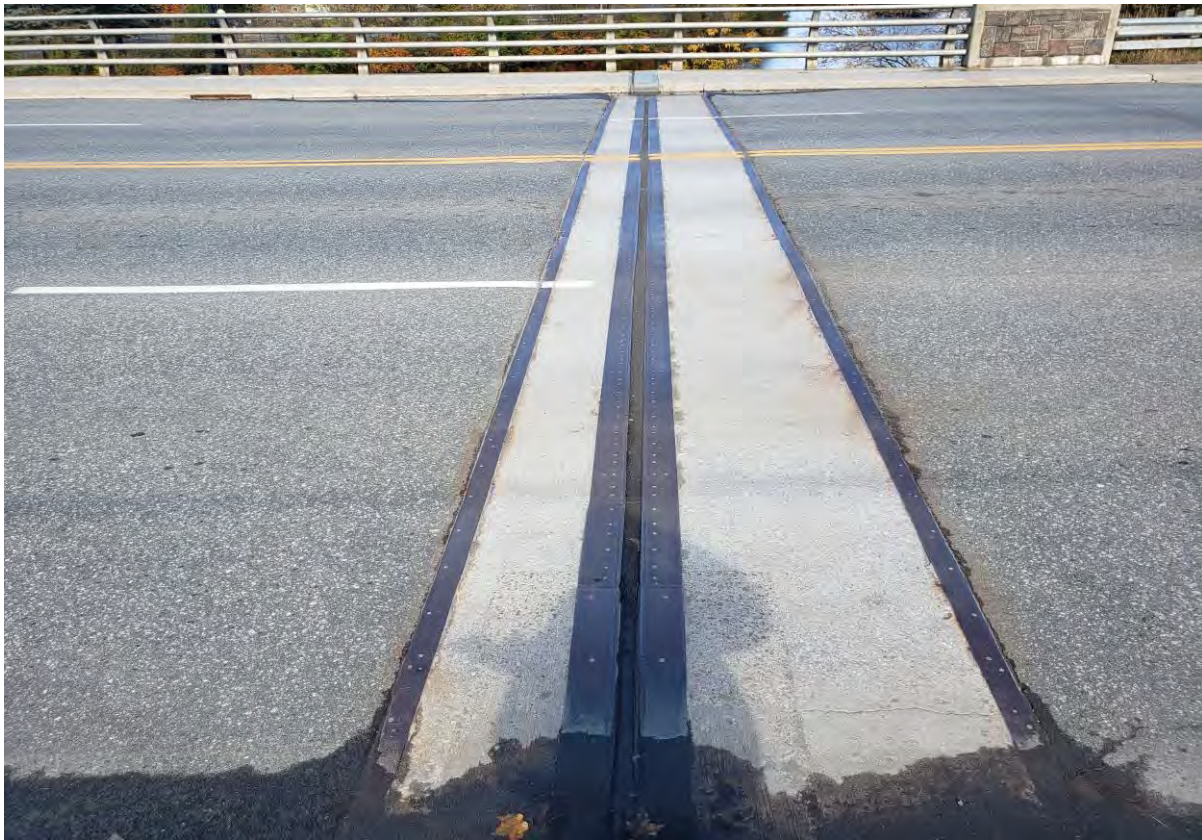
Description of Photo: Photo 15 - Joint End Dam.jpg
