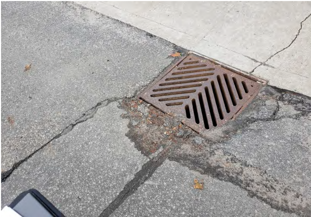
Description of Photo: Photo 3 - Approach Catchbasin
