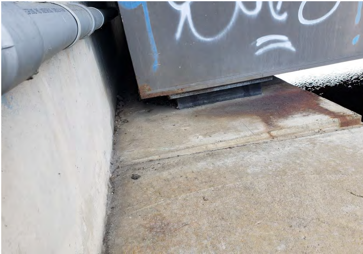
Description of Photo: Photo 61 - Bearings.jpg
