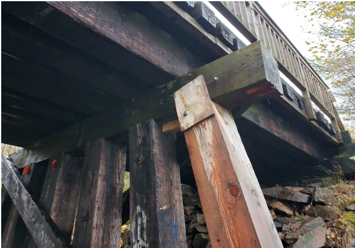
Description of Photo: Photo 28 - Piers.jpg
