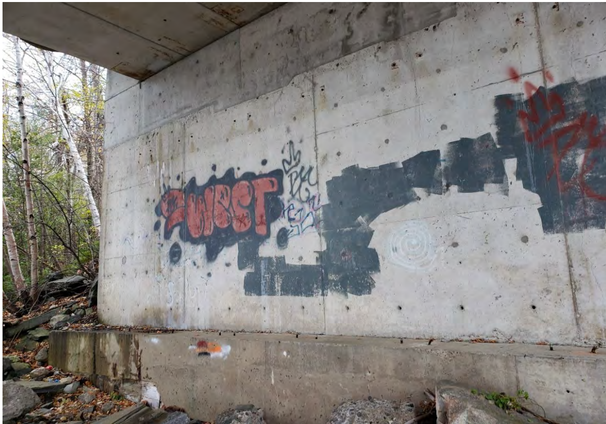
Description of Photo: Photo 28 - Abutment Wall
