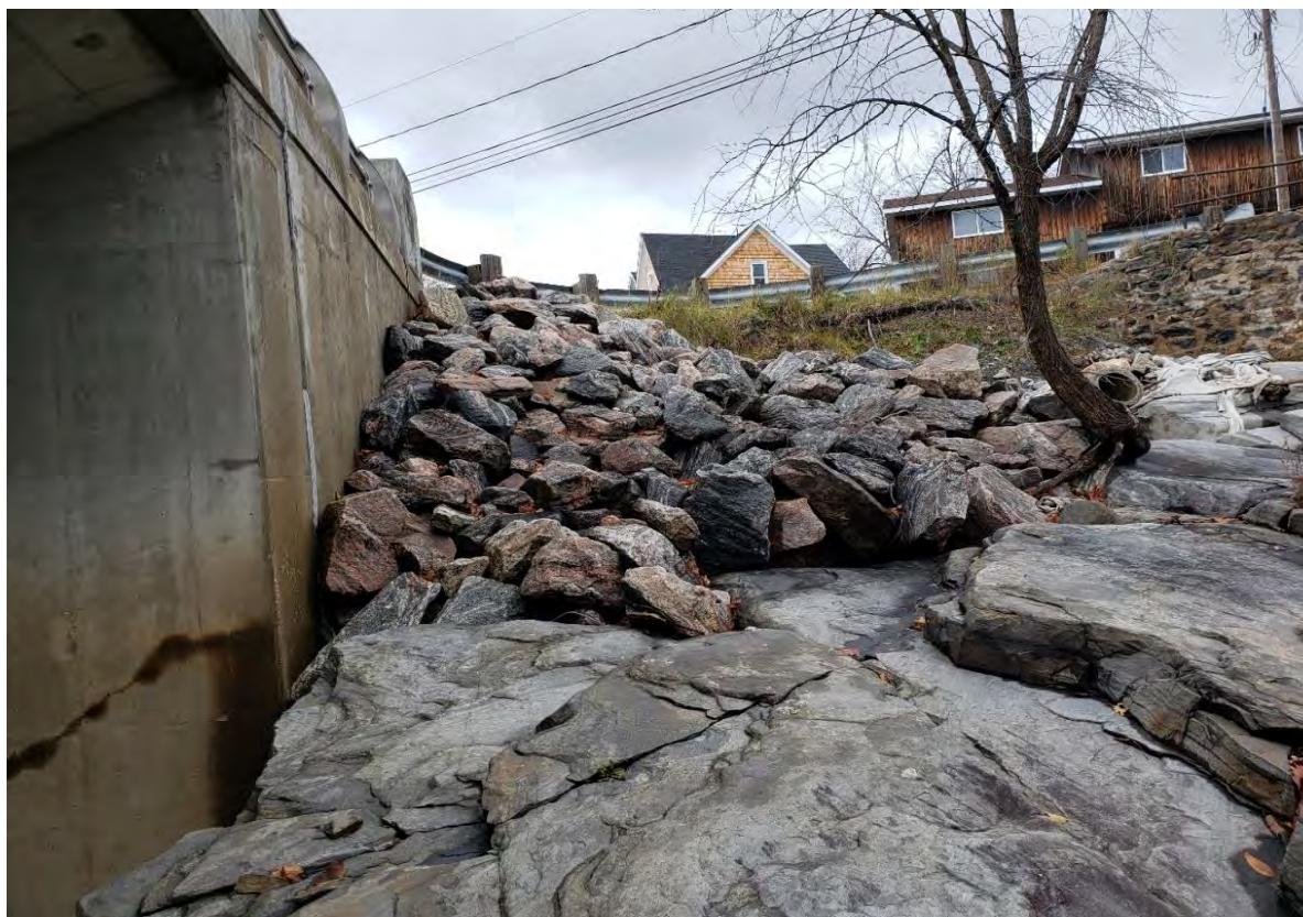
Description of Photo: Photo 29 - Wingwall
