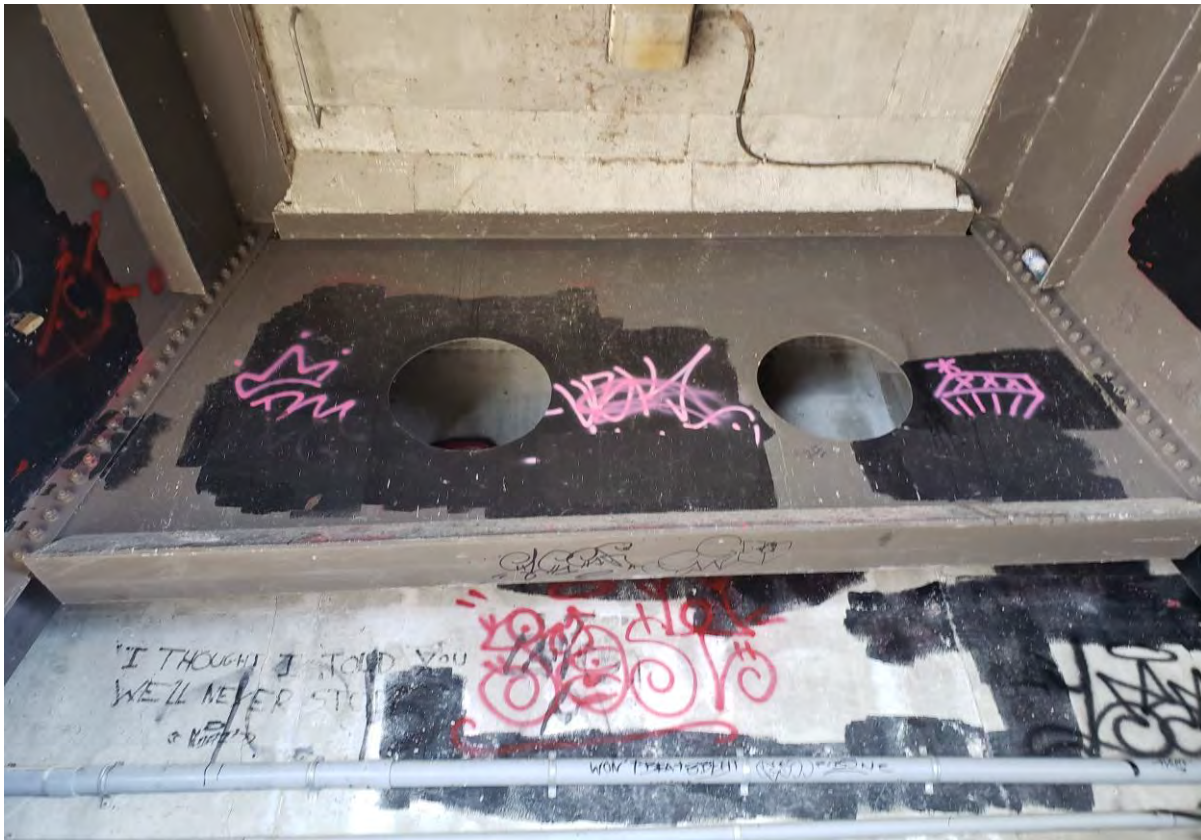
Description of Photo: Photo 32 - Diaphragms.jpg
