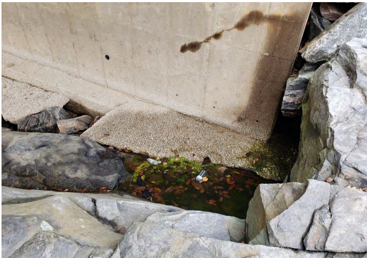
Description of Photo: Photo 32 - Foundation
