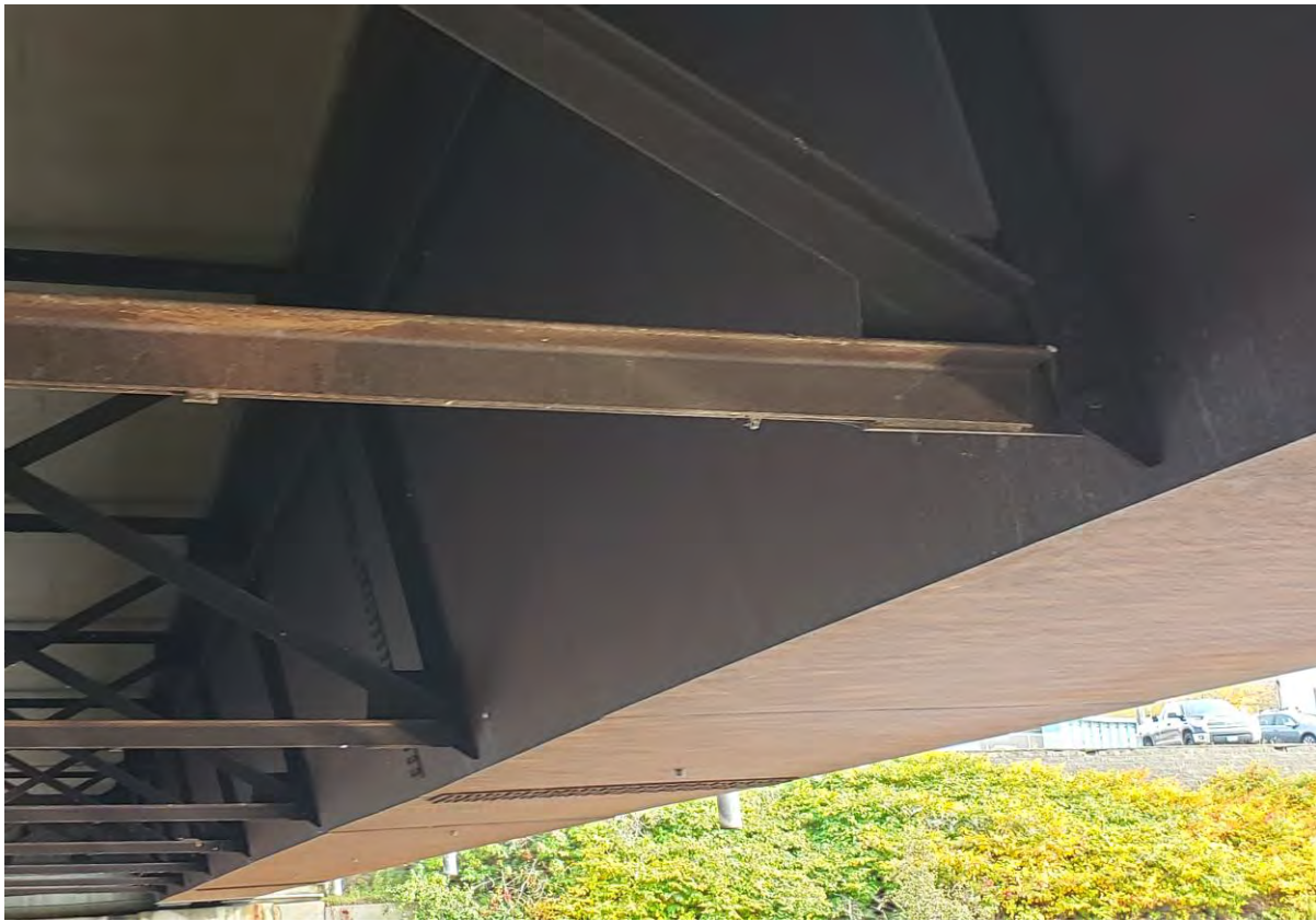
Description of Photo: Photo 33 - Diaphragms.jpg
