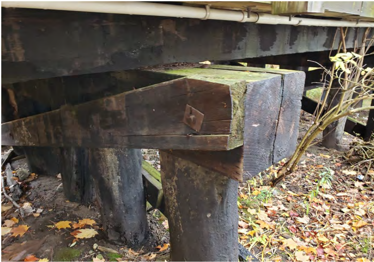
Description of Photo: Photo 38 - Pile Cap.jpg
