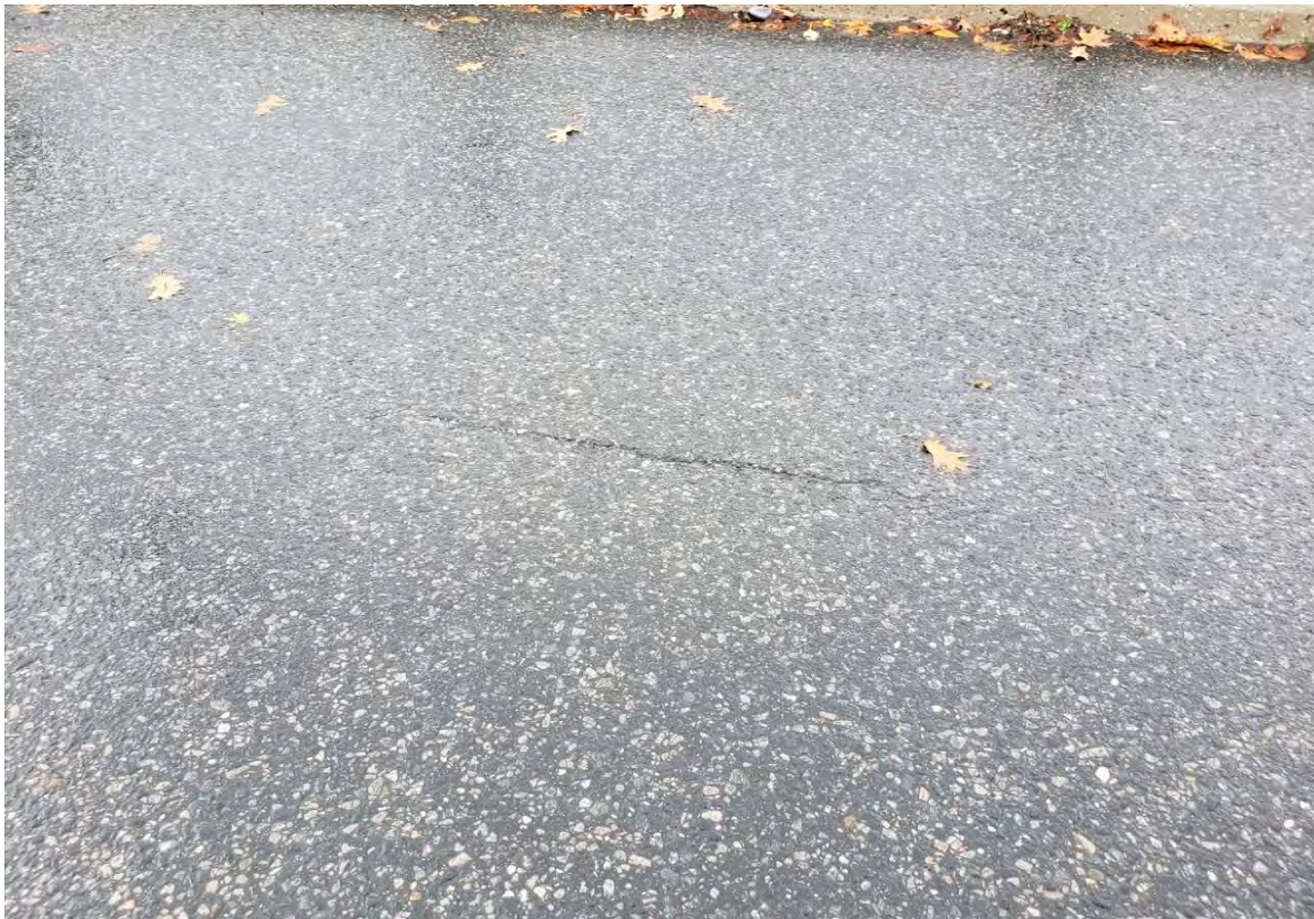
Description of Photo: Photo 13 - Deck Top
