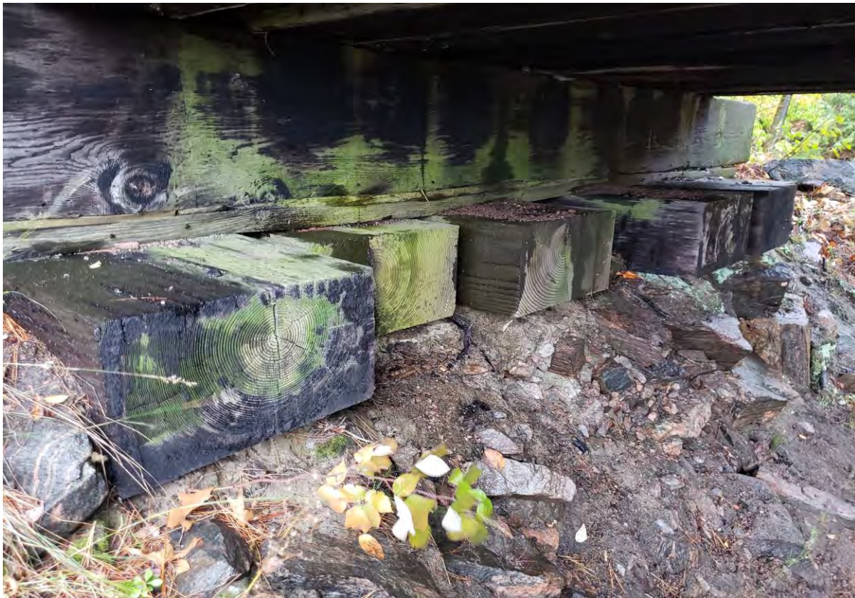
Description of Photo: Photo 25 - Abutment Wall.jpg
