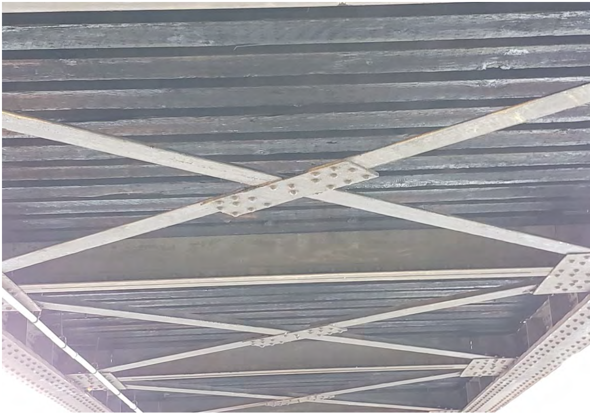
Description of Photo: Photo 56 - Diaphragms.jpg
