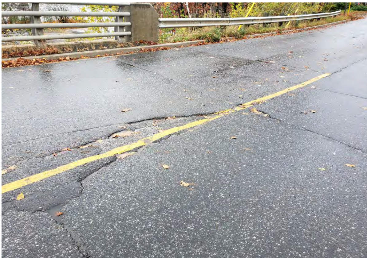
Description of Photo: Photo 10 - Wearing Surface.jpg
