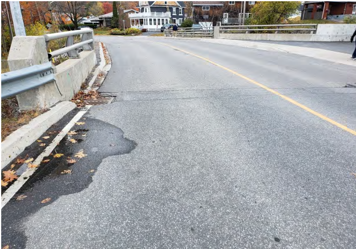
Description of Photo: Photo 2 - Approach Slab
