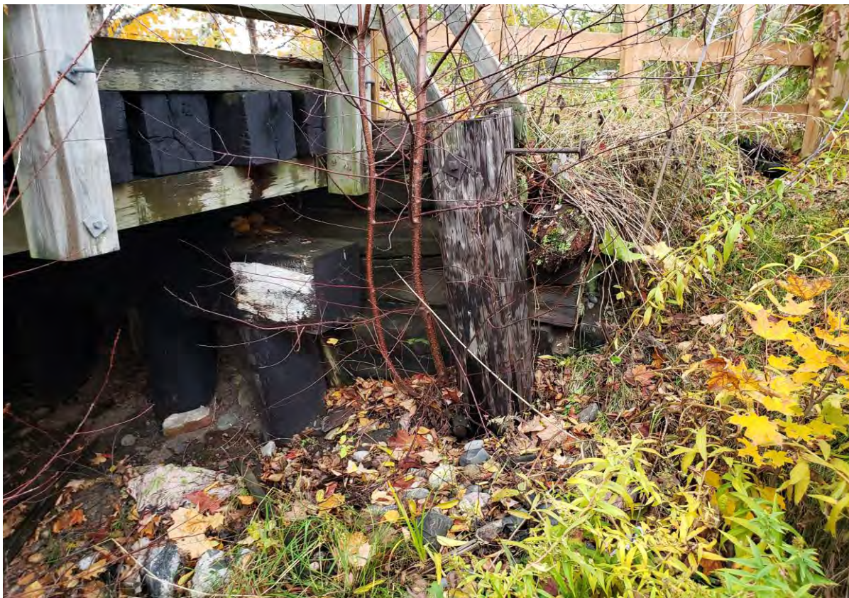
Description of Photo: Photo 30 - Wingwall Piers.jpg
