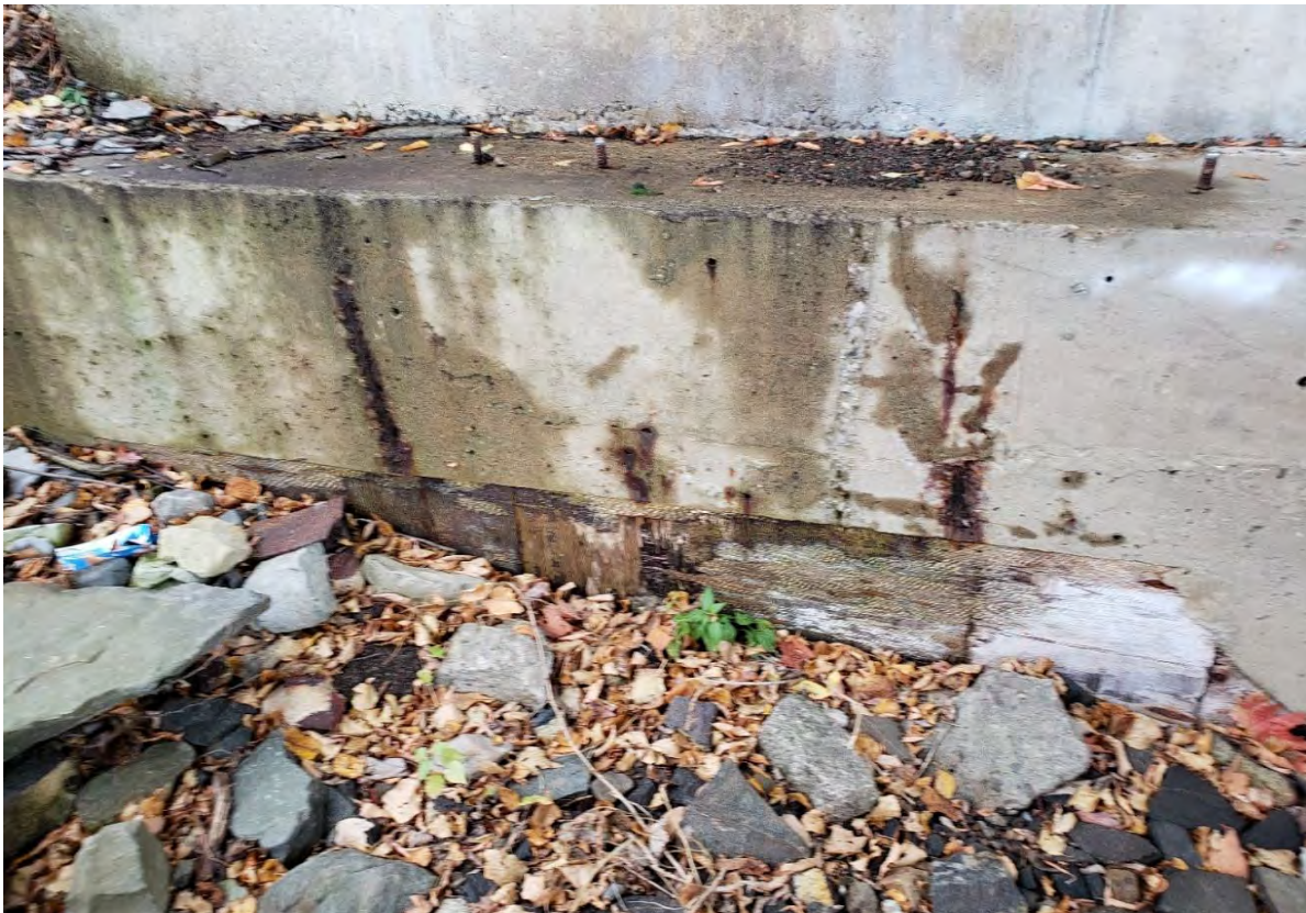
Description of Photo: Photo 33 - Foundation
