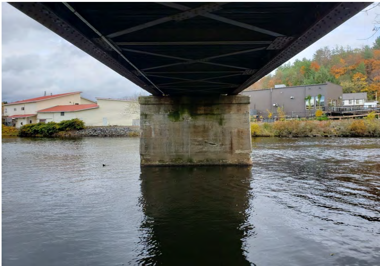
Description of Photo: Photo 57 - Floor Beams
