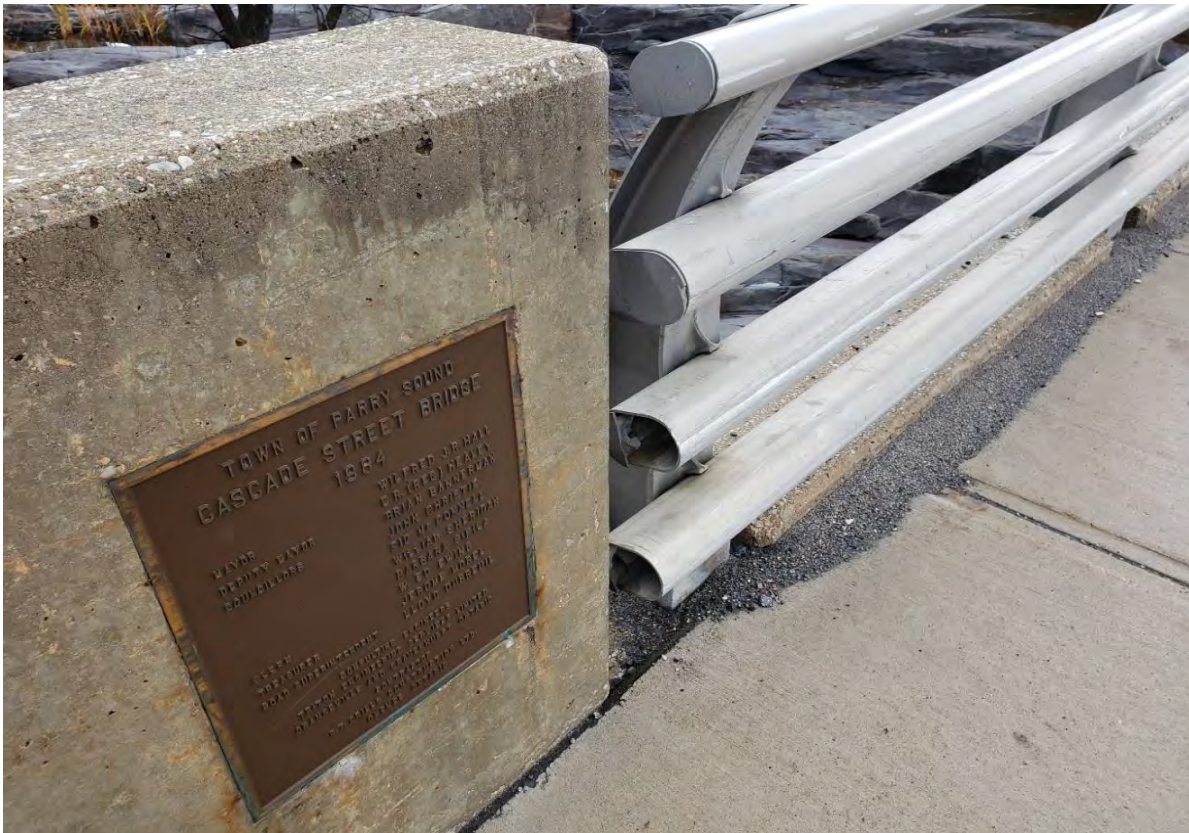
Description of Photo: Photo 21 - Barrier
