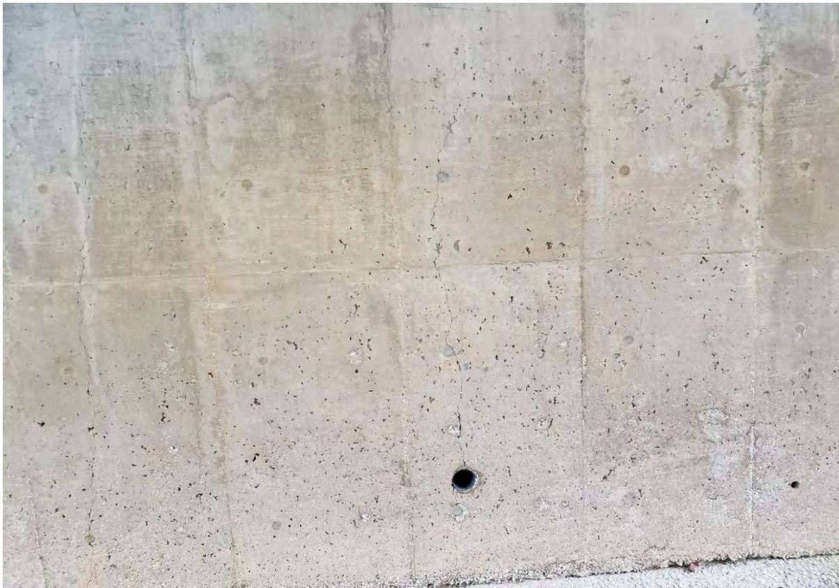
Description of Photo: Photo 17 - Abutment Wall Drain
