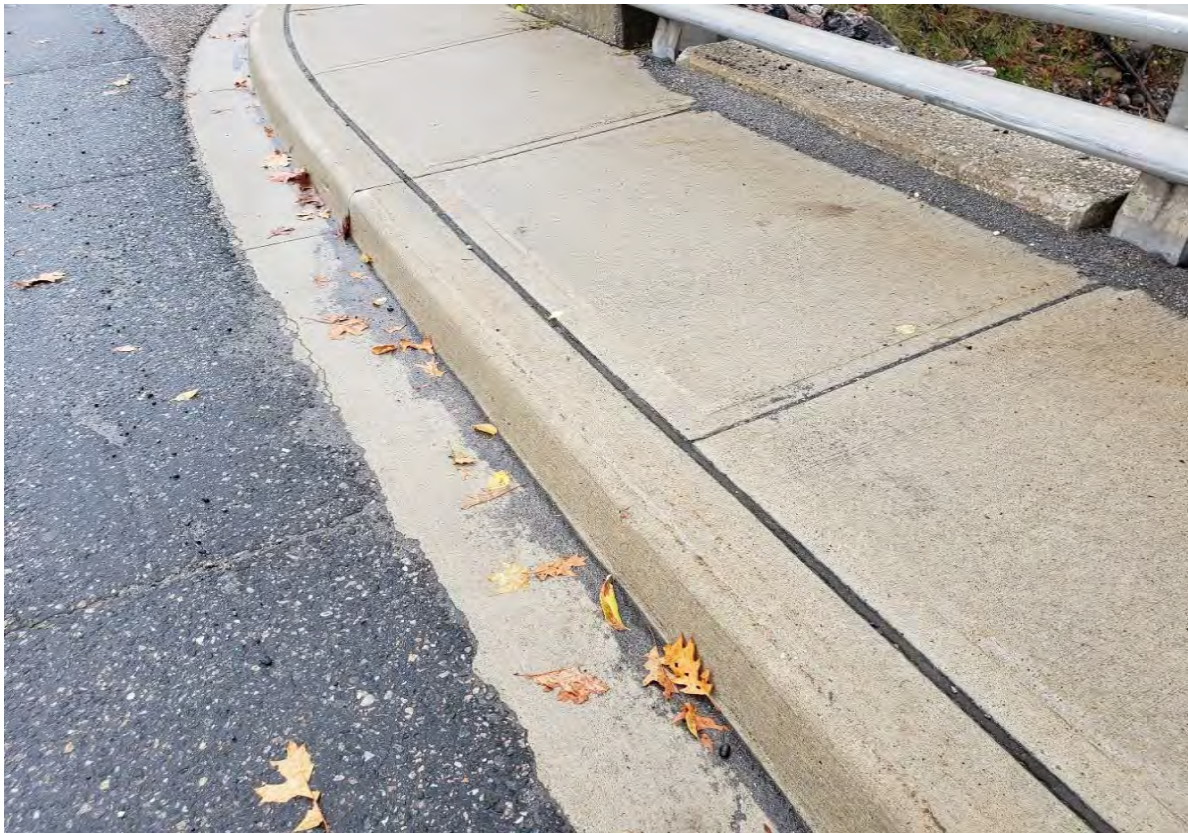
Description of Photo: Photo 4 - Approach Sidewalk
