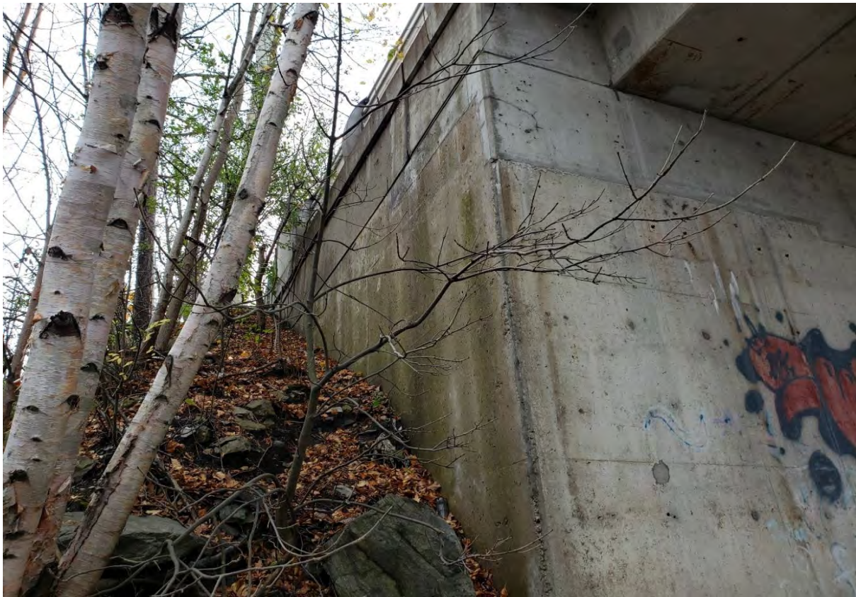
Description of Photo: Photo 31 - Wingwall
