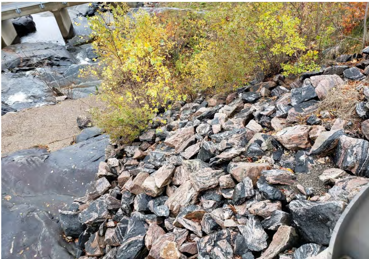
Description of Photo: Photo 34 - Embankment
