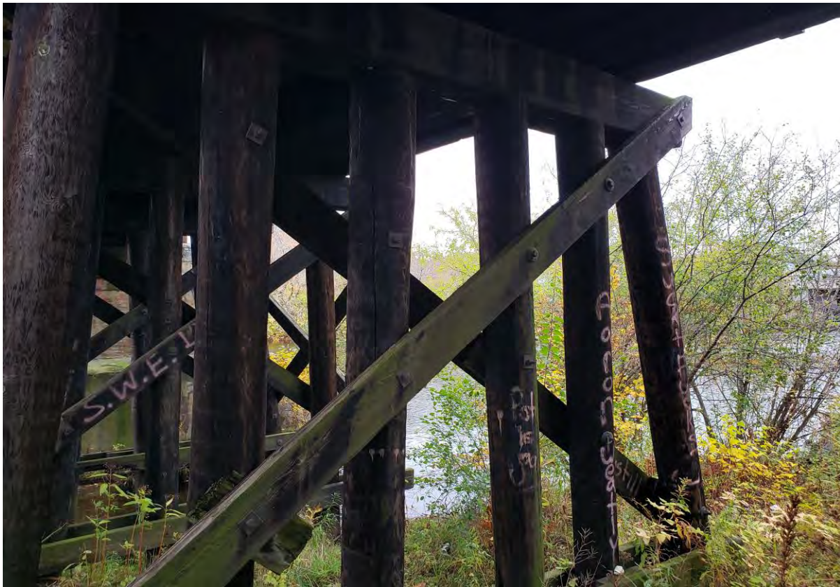
Description of Photo: Photo 43 - Bracing.jpg
