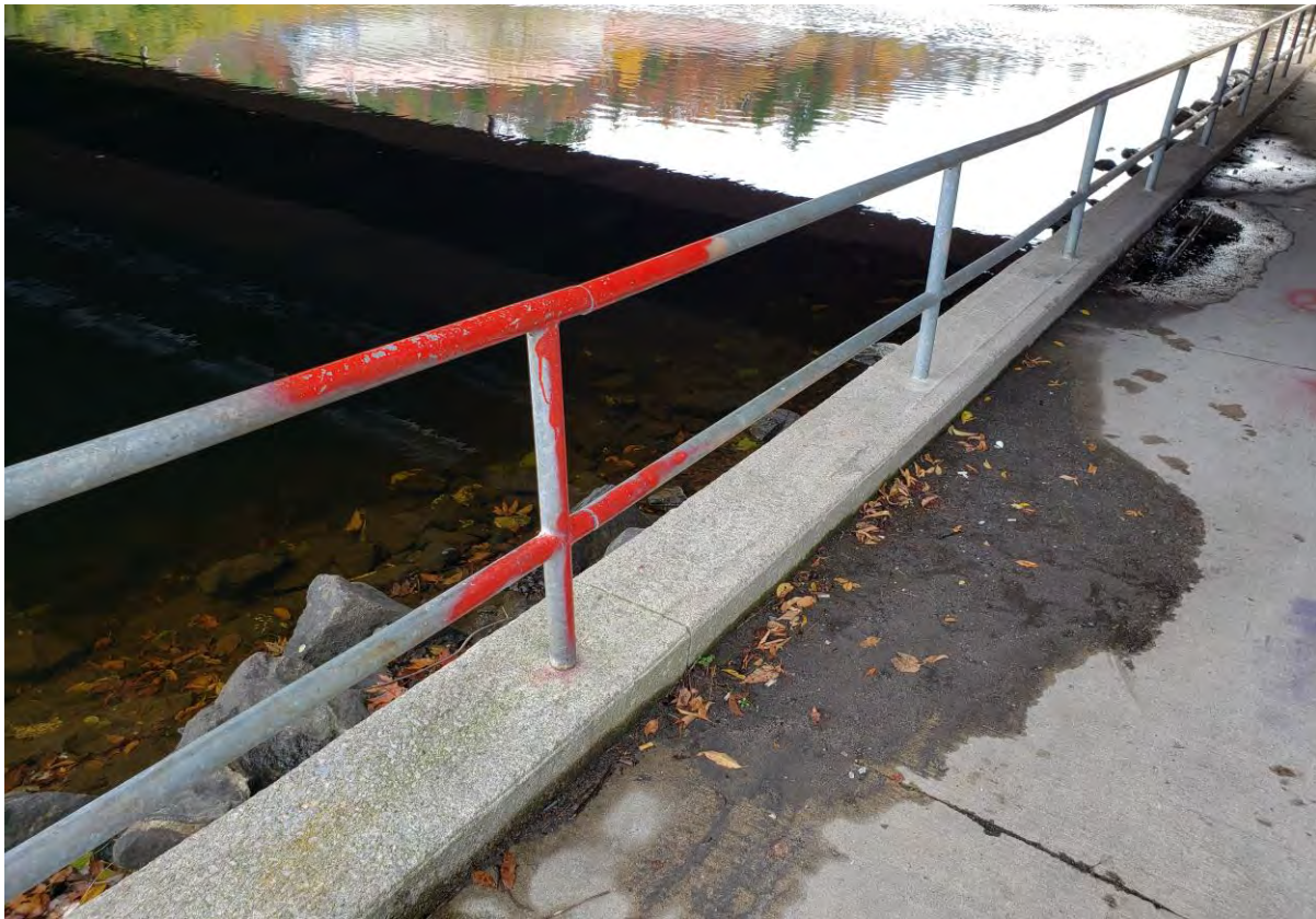
Description of Photo: Photo 25 - Lower Railing.jpg
