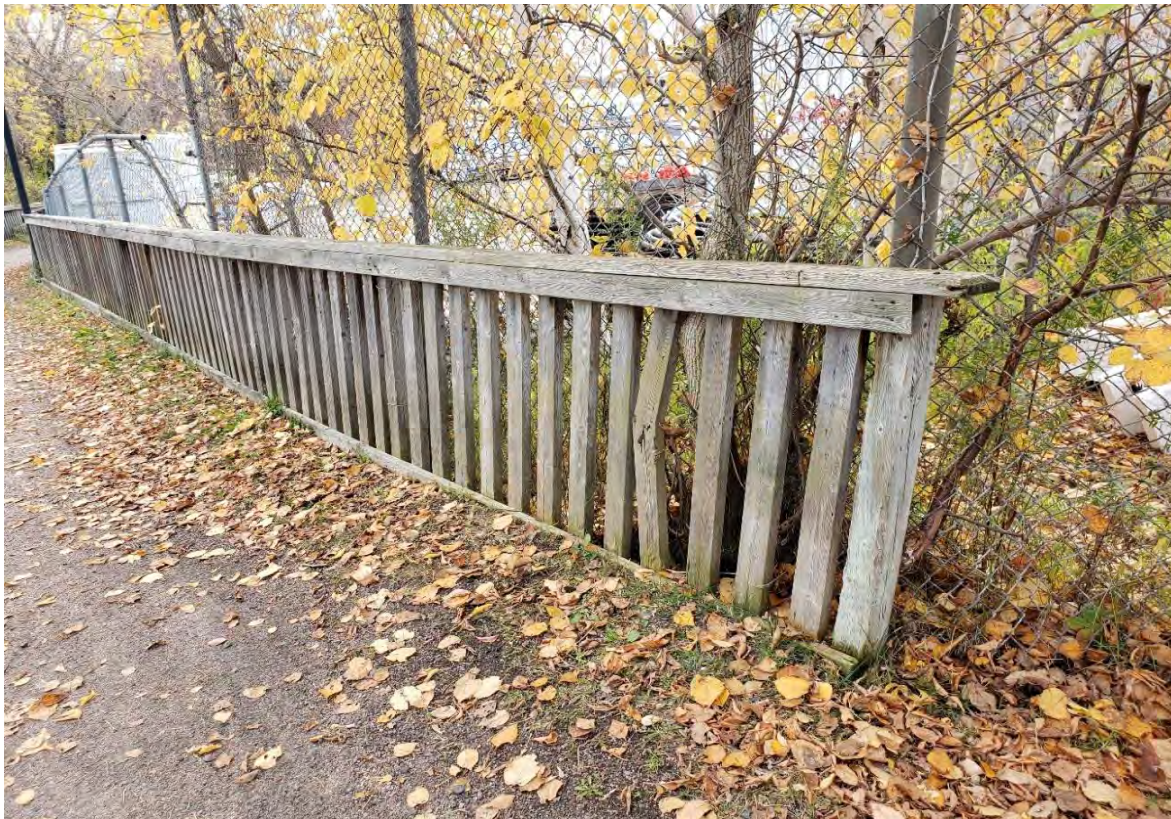
Description of Photo: Photo 32 - Railing
