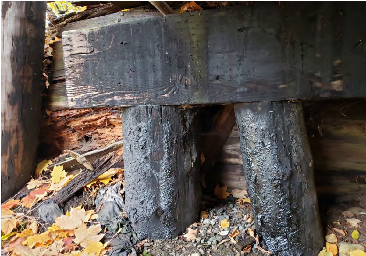
Description of Photo: Photo 22 - Abutment Wall.jpg
