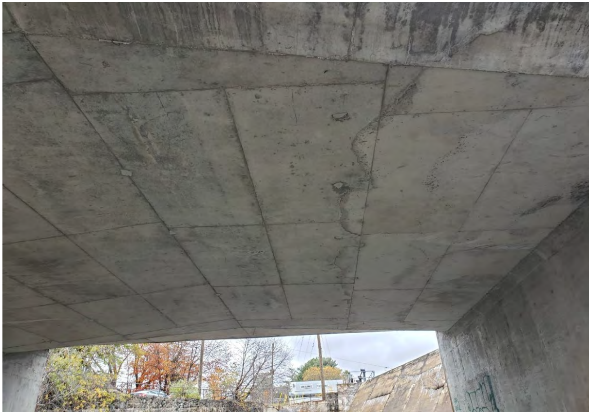
Description of Photo: Photo 14 - Soffit
