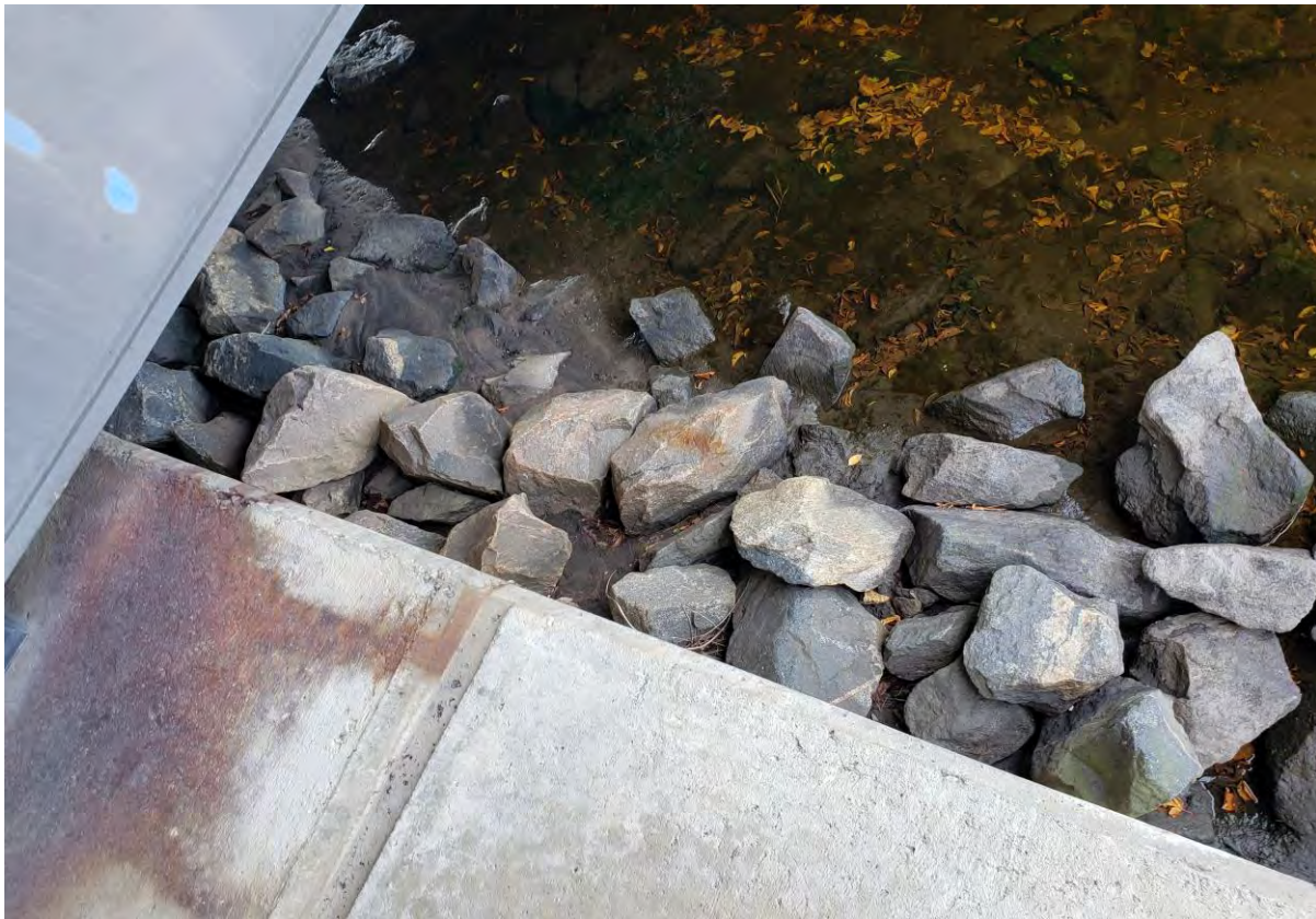
Description of Photo: Photo 71 - Slope Protection.jpg
