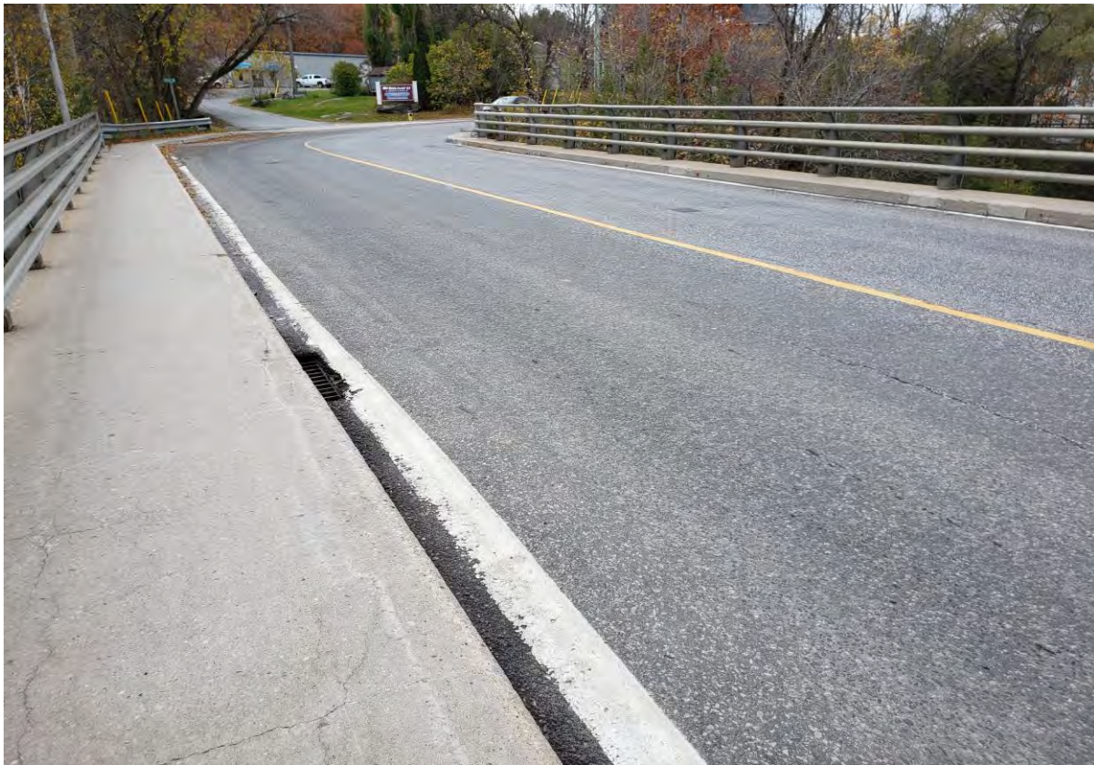
Description of Photo: Photo 13 - Wearing Surface.jpg
