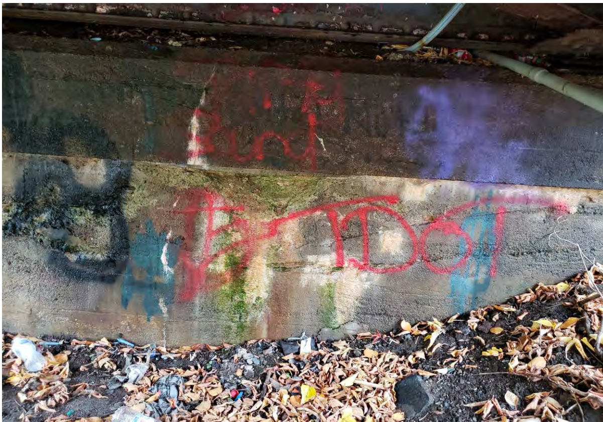
Description of Photo: Photo 19 - Abutment Wall.jpg
