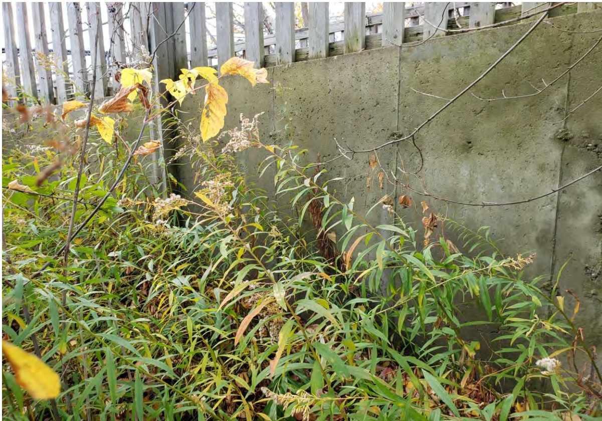
Description of Photo: Photo 31 - Retaining Wall.jpg
