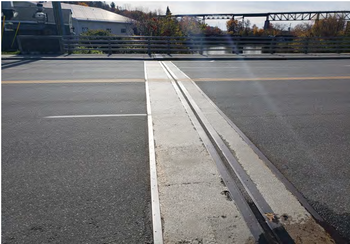
Description of Photo: Photo 18 - Armouring.jpg
