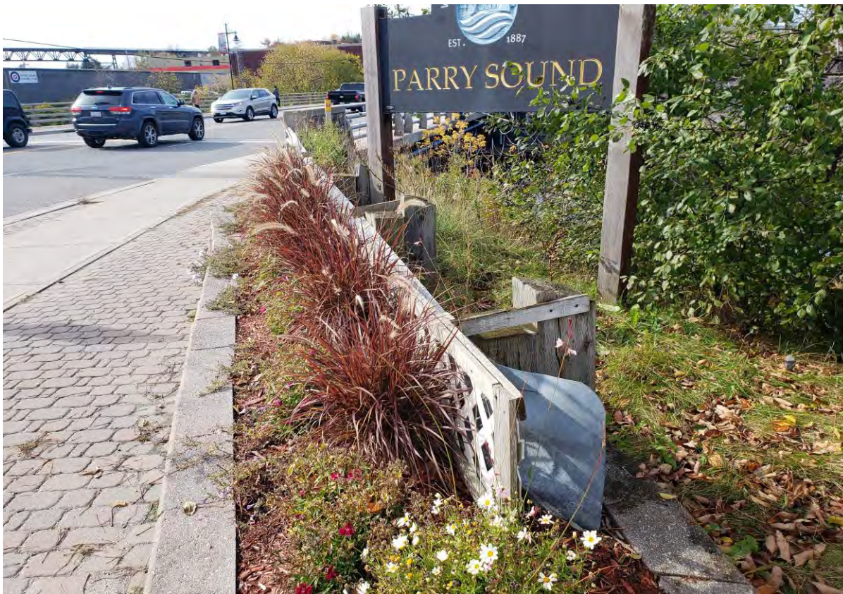
Description of Photo: Photo 9 - Approach Barrier.jpg
