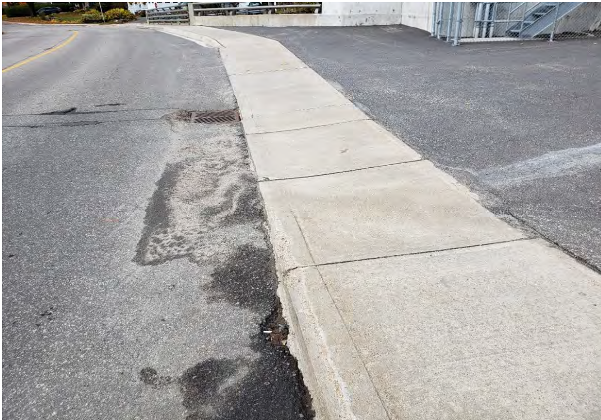
Description of Photo: Photo 9 - Approach Sidewalk
