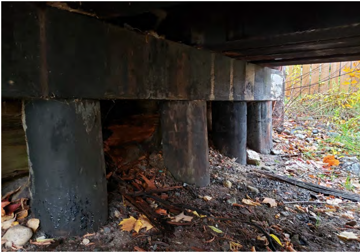
Description of Photo: Photo 25 - Abutment Piles.jpg
