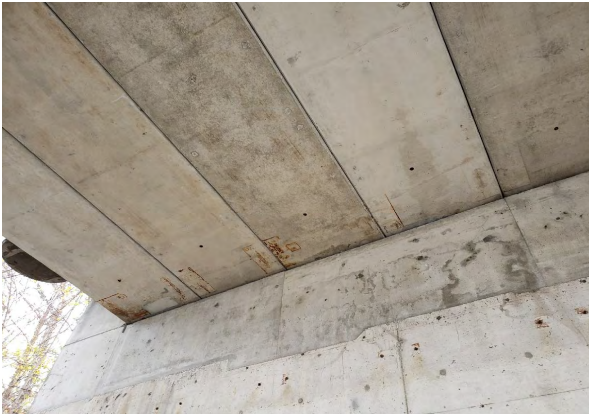
Description of Photo: Photo 39 - Girders
