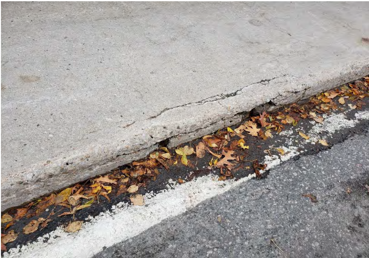
Description of Photo: Photo 21 - Curb
