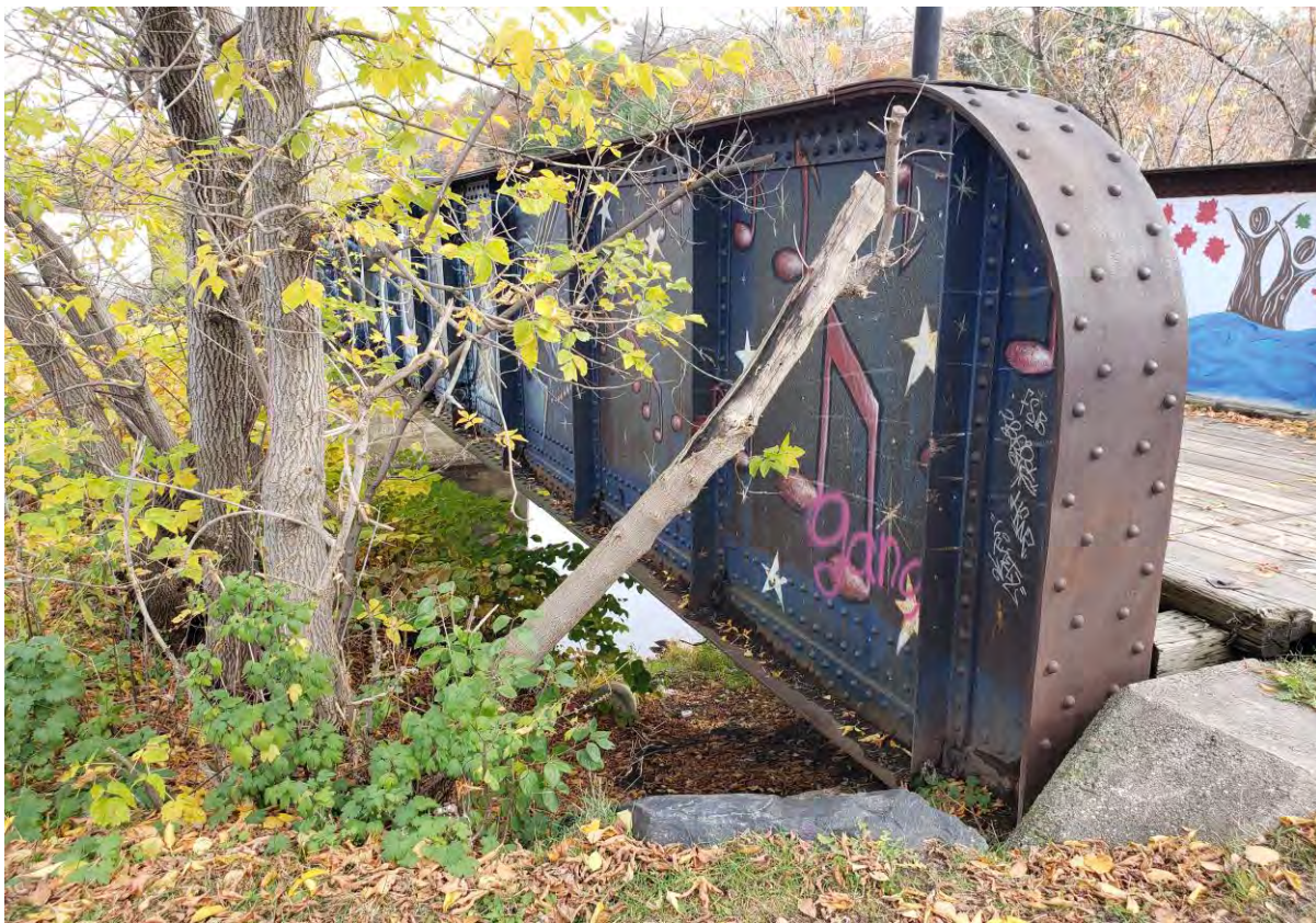
Description of Photo: Photo 55 - Girders.jpg
