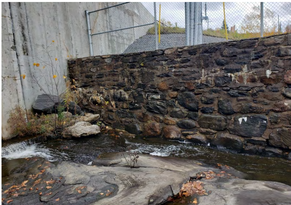
Description of Photo: Photo 36 - Retaining Wall
