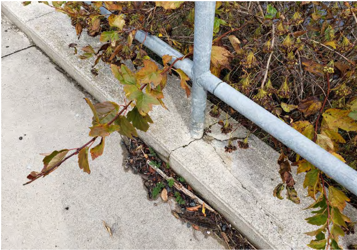
Description of Photo: Photo 63 - Retaining Wall.jpg
