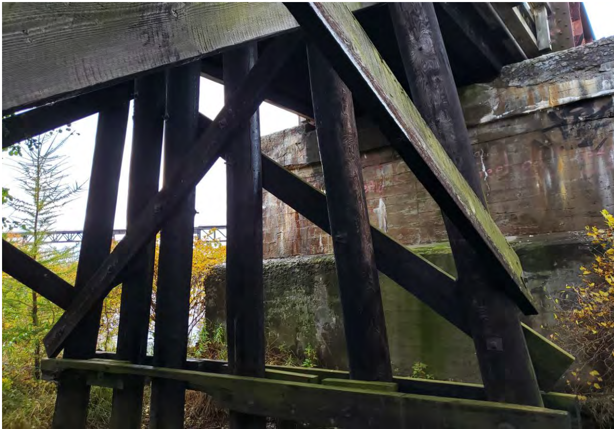
Description of Photo: Photo 40 - Piles.jpg
