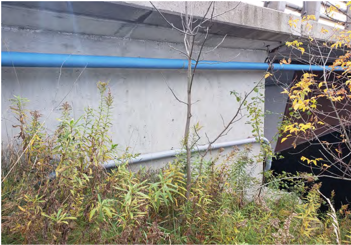
Description of Photo: Photo 53 - Wingwall.jpg
