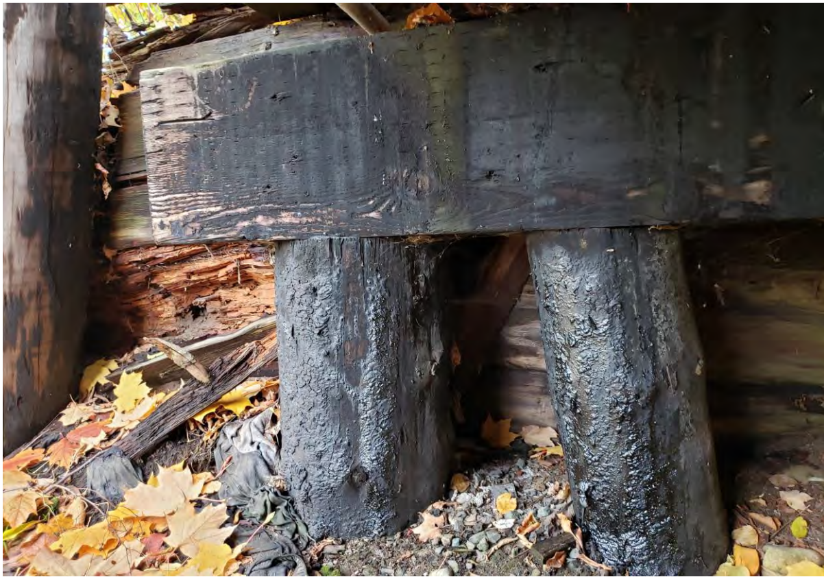
Description of Photo: Photo 26 - Abutment Pile Cap.jpg
