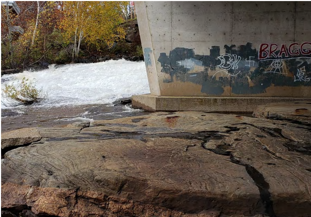
Description of Photo: Photo 43 - Pier
