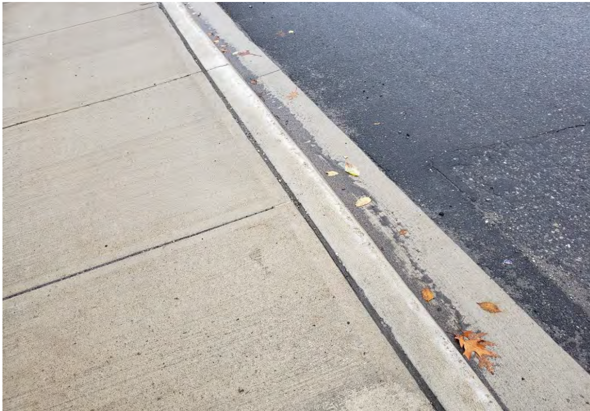
Description of Photo: Photo 5 - Approach Curb
