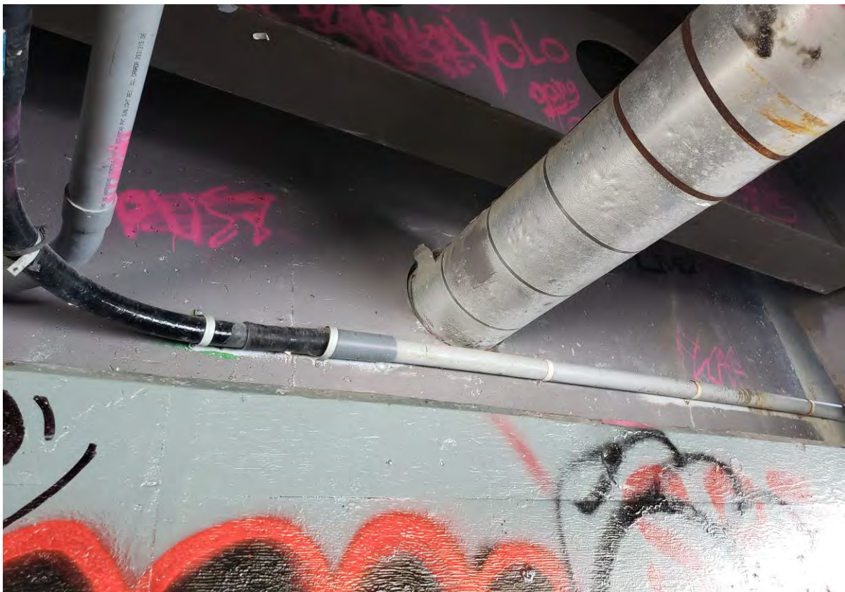
Description of Photo: Photo 51 - Ballast Wall.jpg
