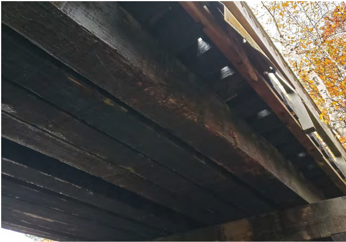
Description of Photo: Photo 19 - Beams.jpg
