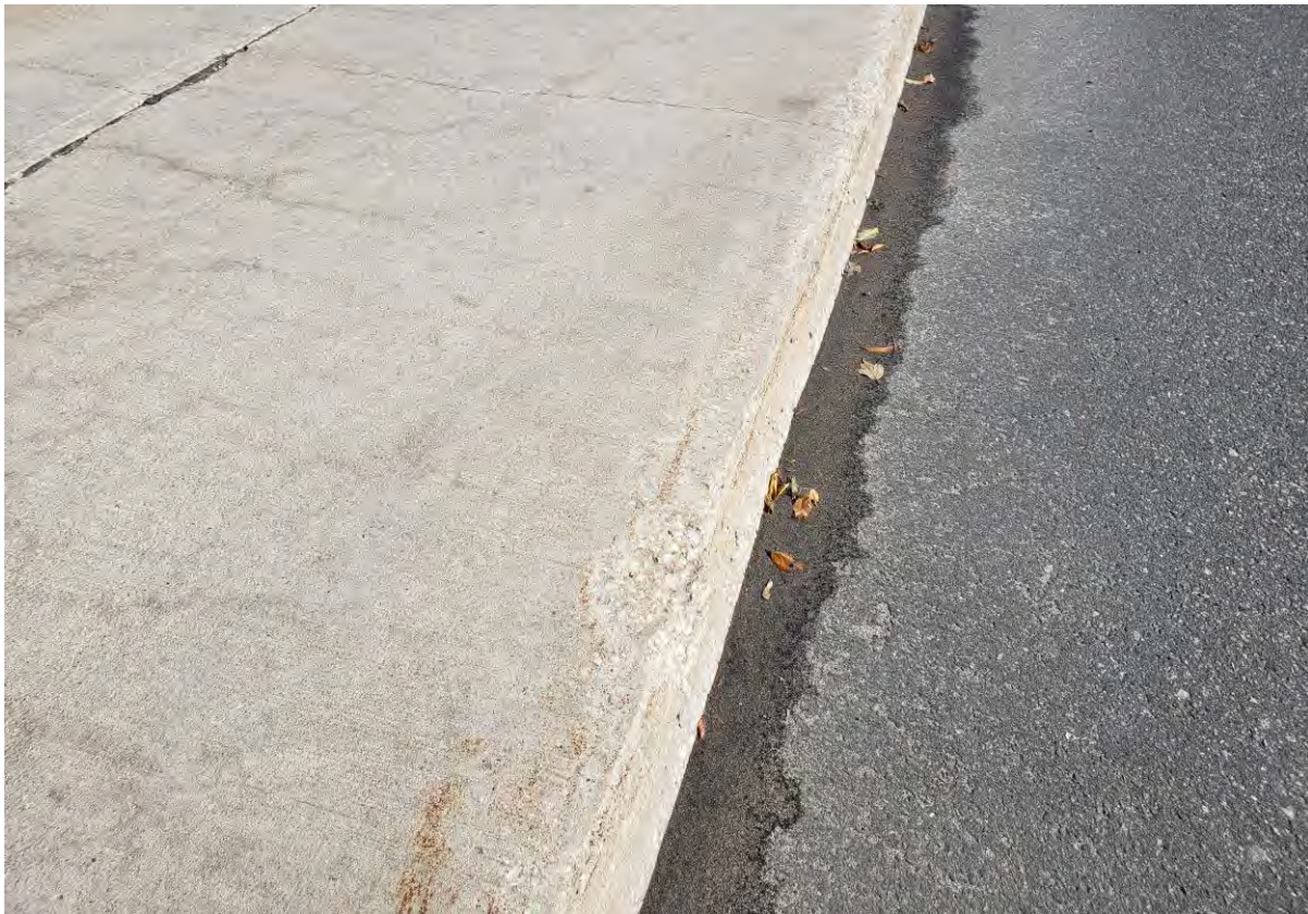
Description of Photo: Photo 6 - Approach Curb.jpg
