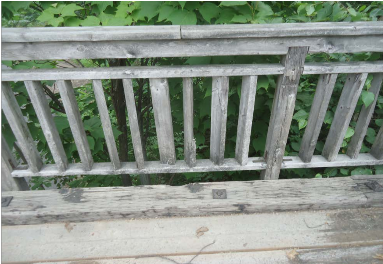
Description of Photo: Photo 7 - Railing
