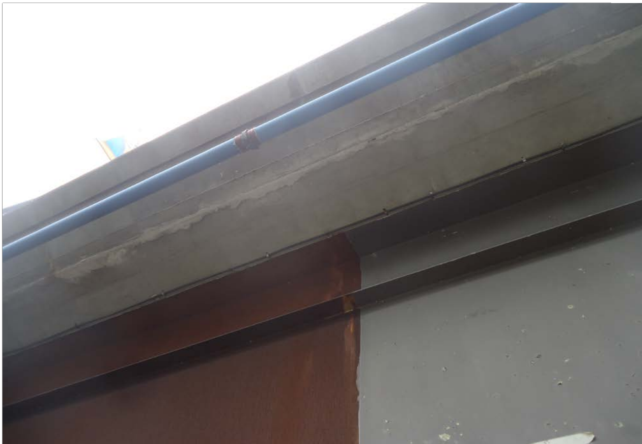
Description of Photo: Photo 10 - Soffit Exterior
