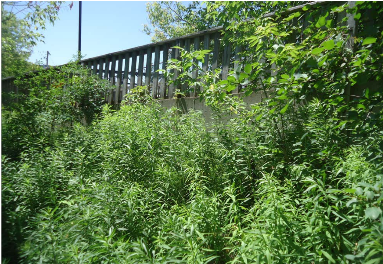
Description of Photo: Photo 24 - Southwest Retaining Wall
