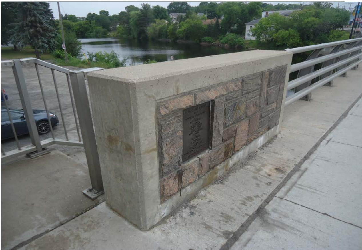
Description of Photo: Photo 85 - Approach - no barrier
