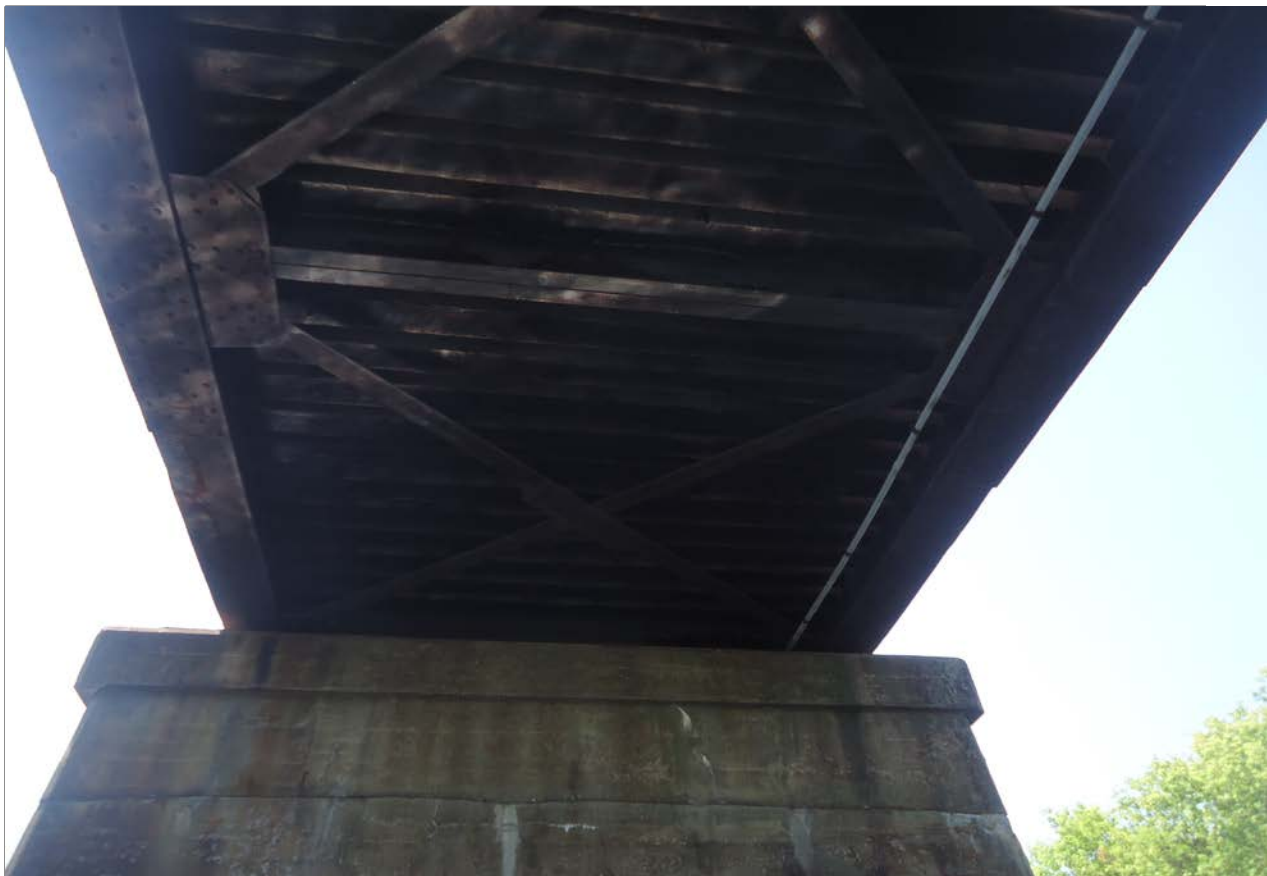
Description of Photo: Photo 63 - Steel Diaphragm
