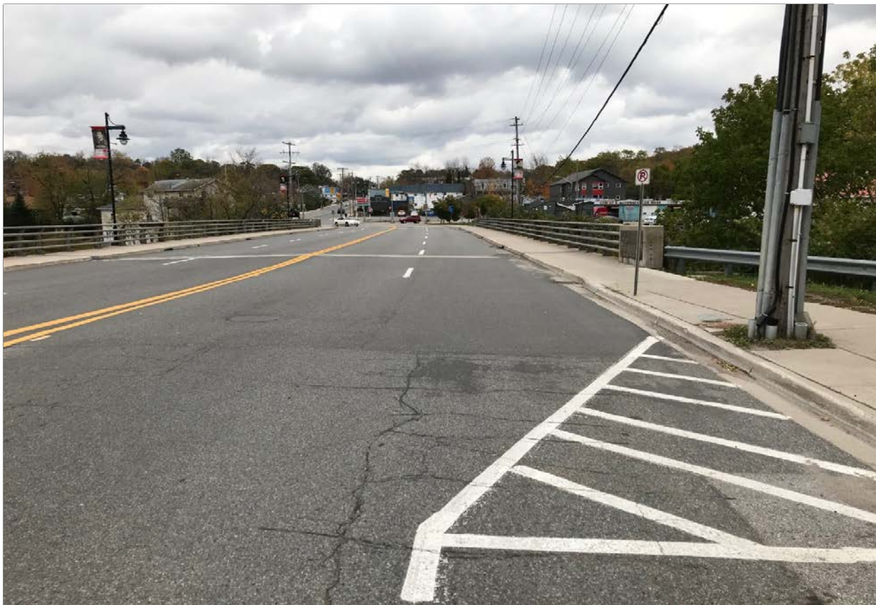
Description of Photo: Photo 75 - West Approach
