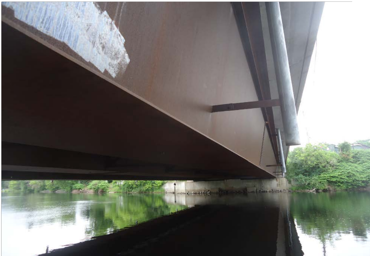
Description of Photo: Photo 34 - Girder Mid
