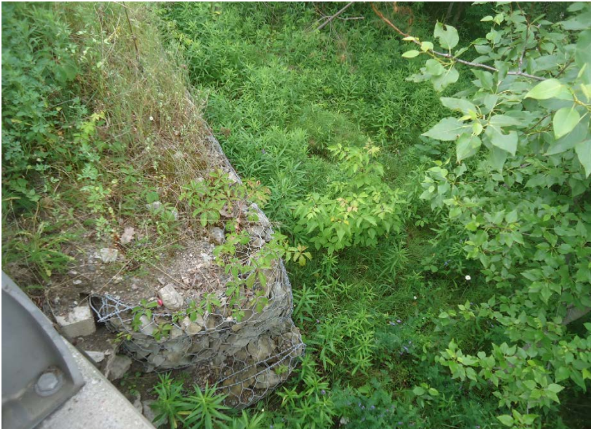
Description of Photo: Photo 47 - Gabion Retaining Wall
