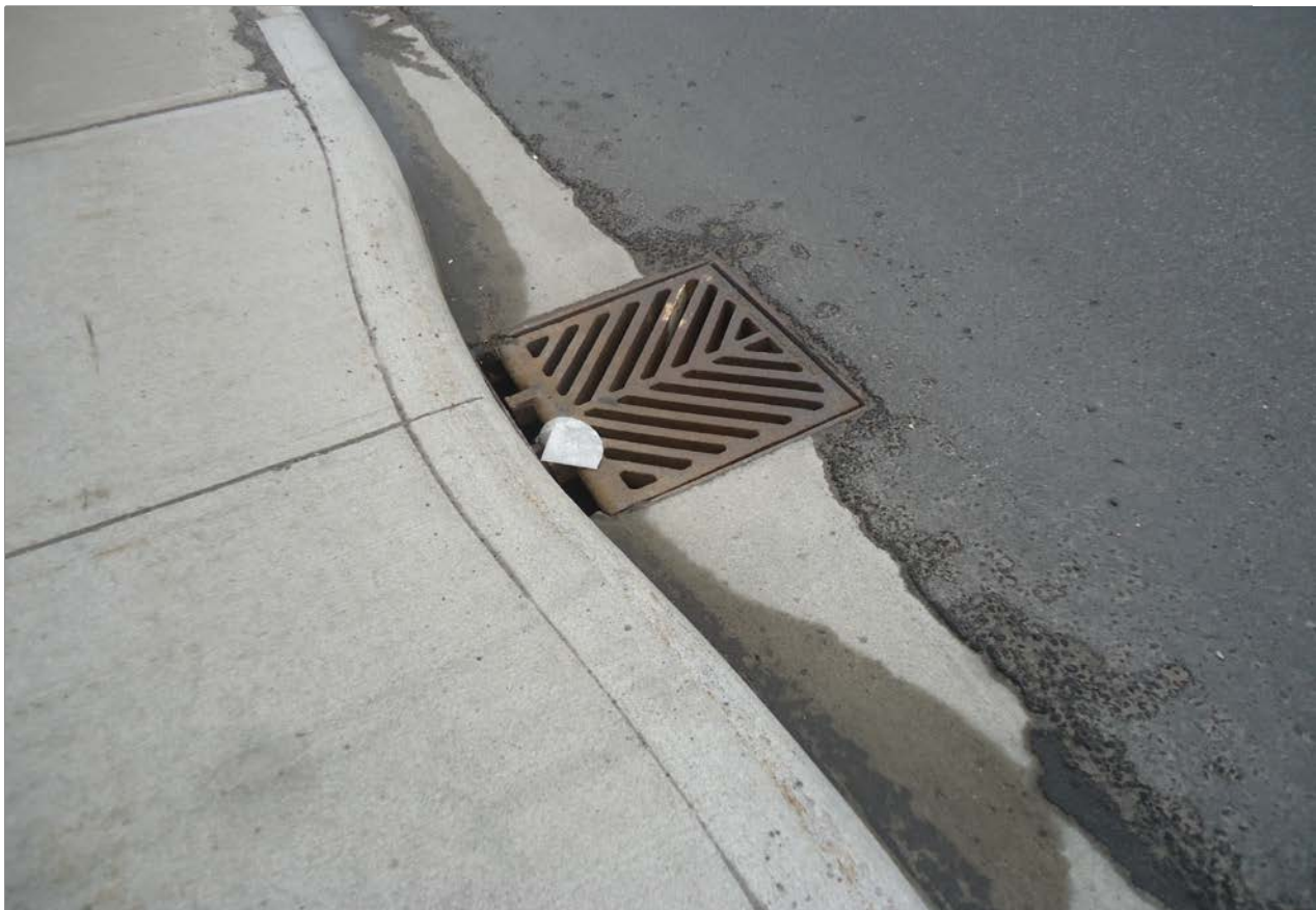
Description of Photo: Photo 79 - Approach Curb
