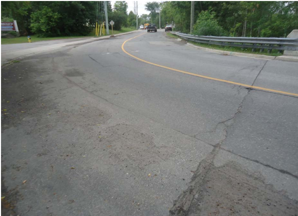
Description of Photo: Photo 41 - Approach Slab
