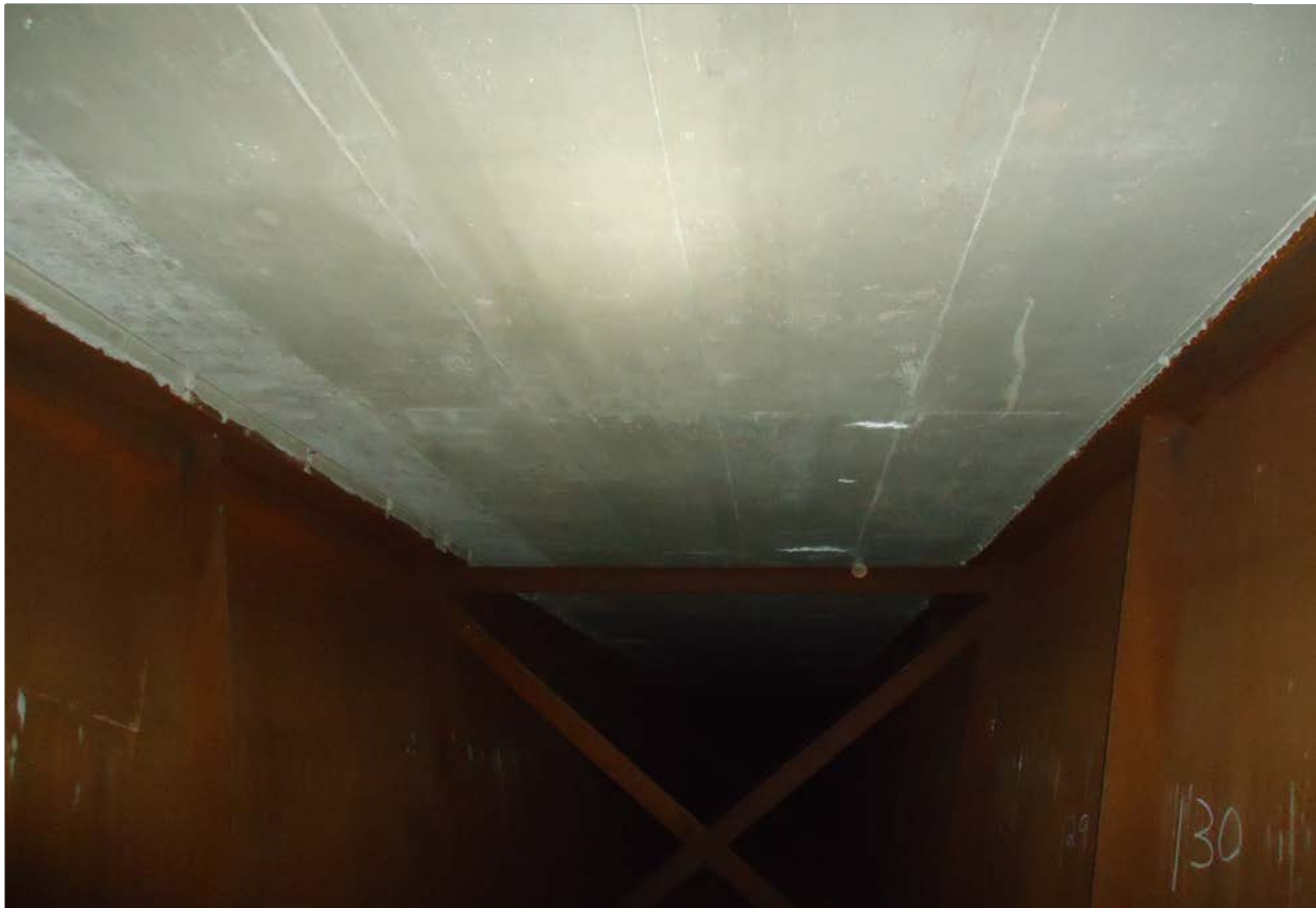
Description of Photo: Photo 4 - Interior Soffit Mid
