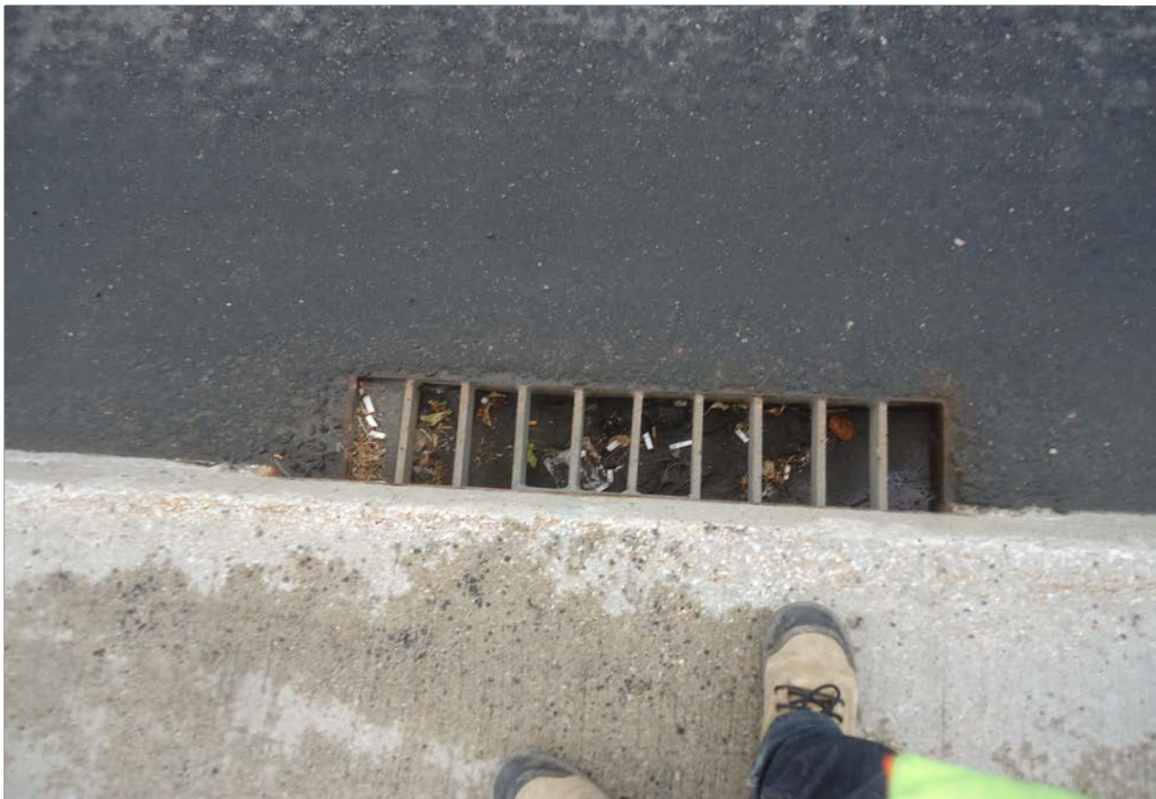
Description of Photo: Photo 5 - Drain
