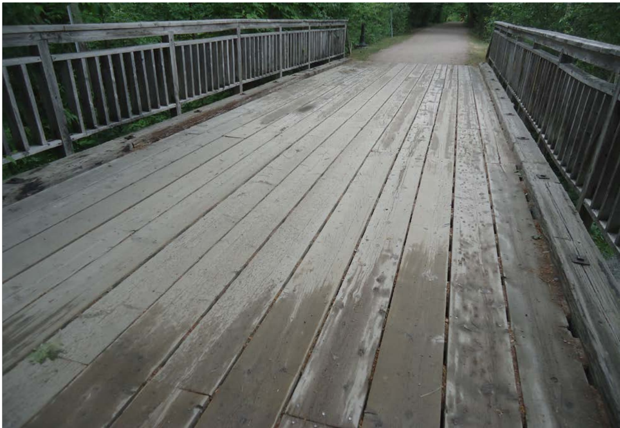
Description of Photo: Photo 1 - Deck Top
