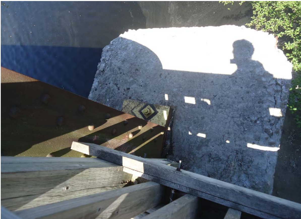
Description of Photo: Photo 46 - Pier Bearing
