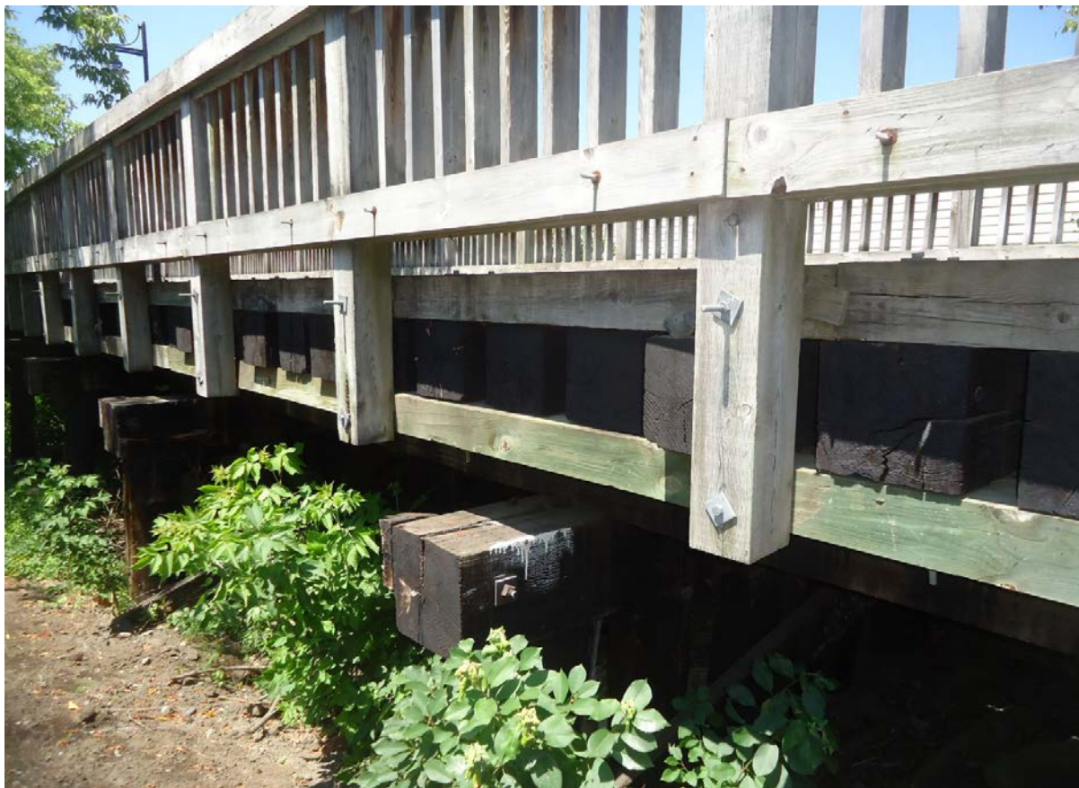
Description of Photo: Photo 39 - Stringer Beams
