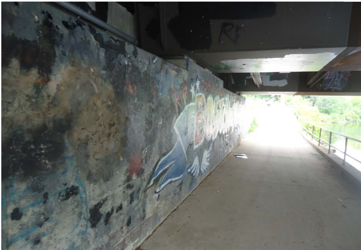
Description of Photo: Photo 50 - Abutment
