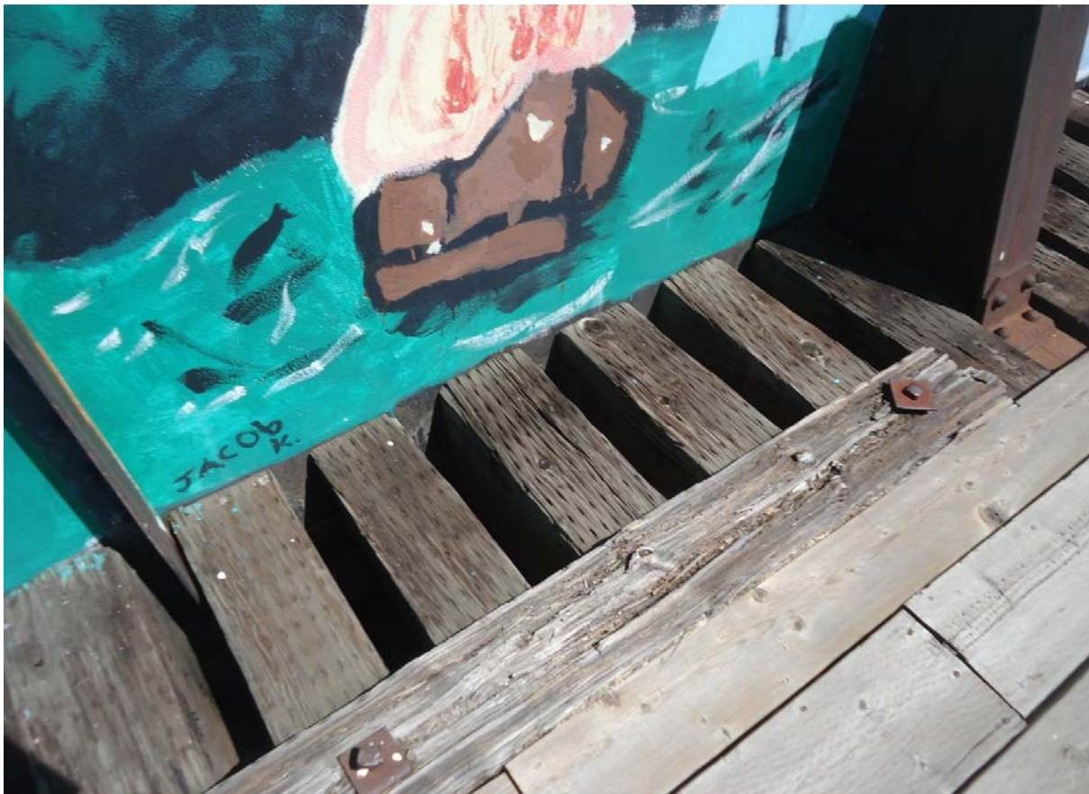
Description of Photo: Photo 4 - Deck Timbers
