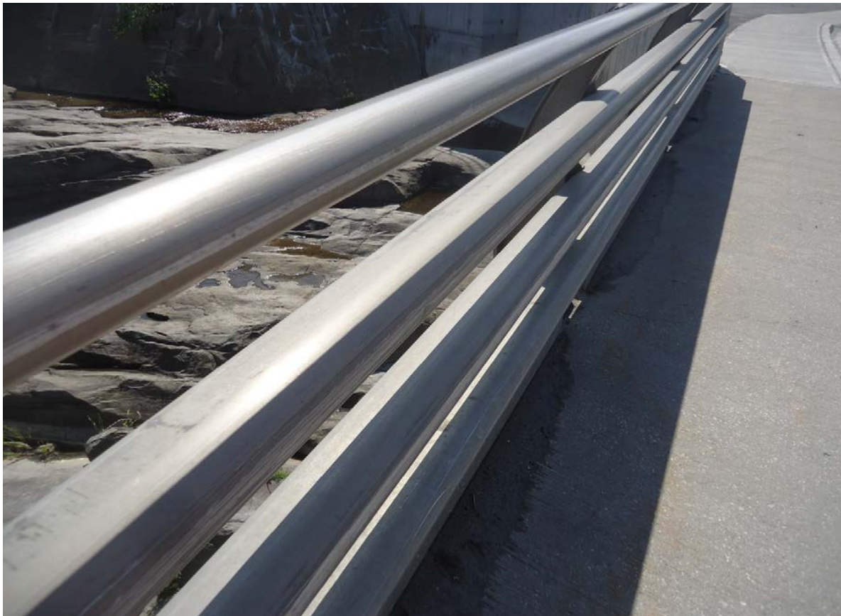
Description of Photo: Photo 12 - Barrier
