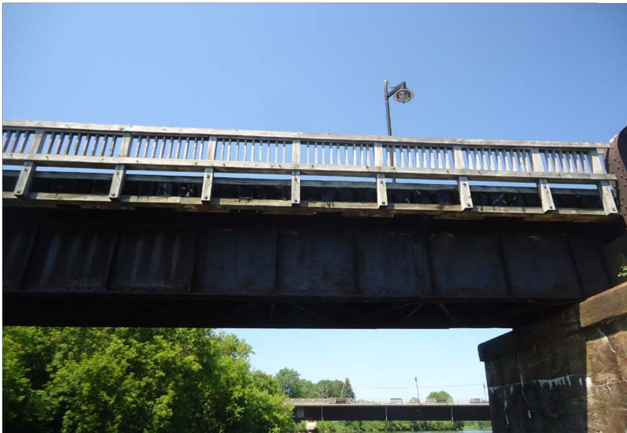
Description of Photo: Photo 57 - Steel Girder
