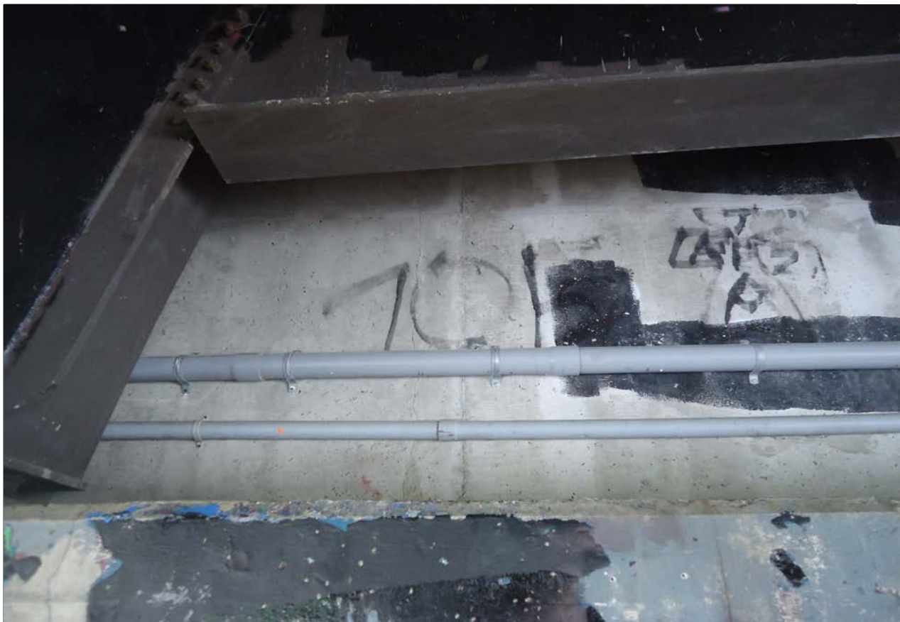
Description of Photo: Photo 53 - Ballast Wall
