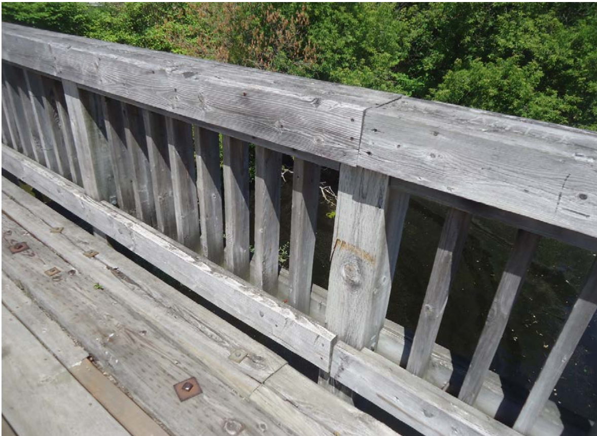
Description of Photo: Photo 10 - Railing
