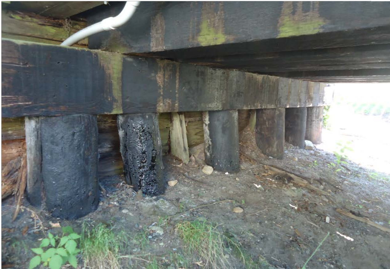
Description of Photo: Photo 16 - East Abutment
