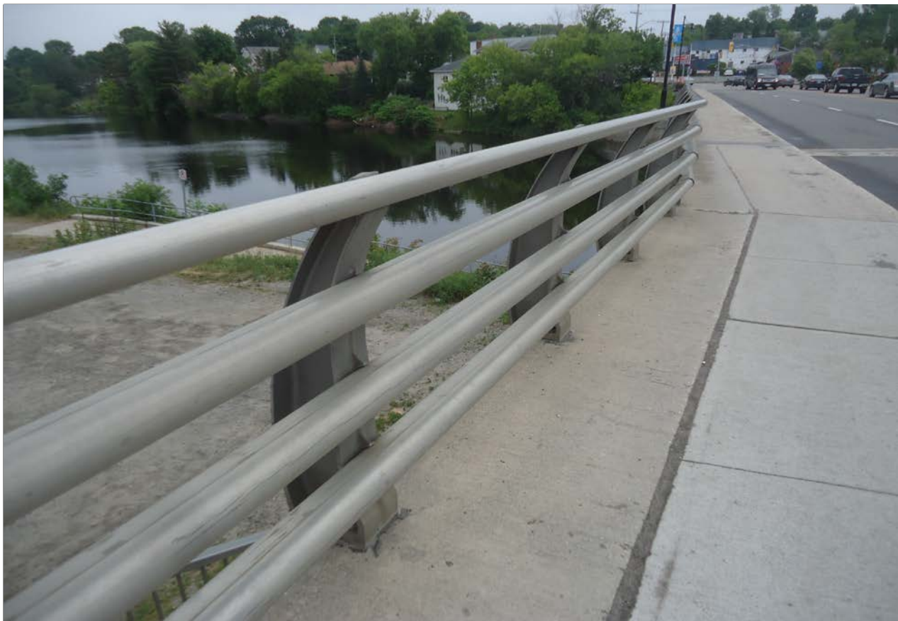
Description of Photo: Photo 65 - Northwest Railing
