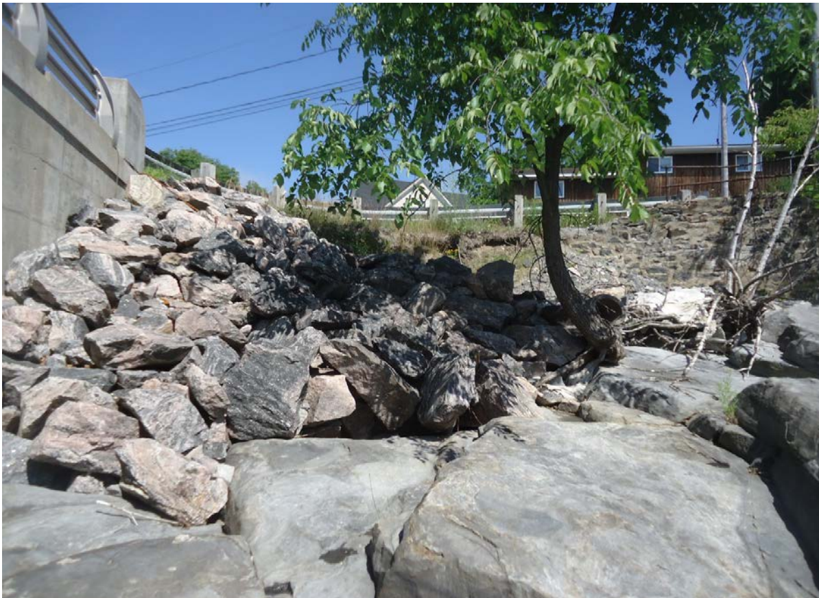
Description of Photo: Photo 24 - Northeast Slope Protection
