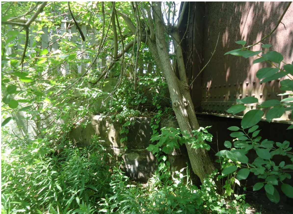
Description of Photo: Photo 21 - Southwest Wingwall
