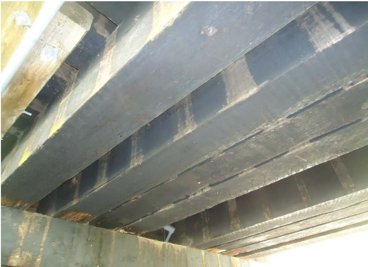
Description of Photo: Photo 37 - Timber Beams
