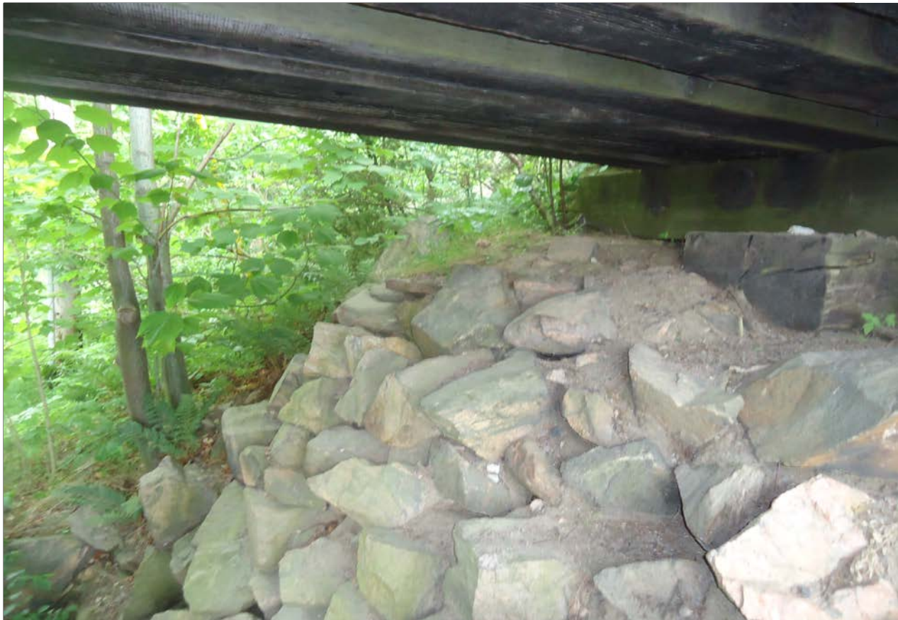
Description of Photo: Photo 28 - Slope Protection
