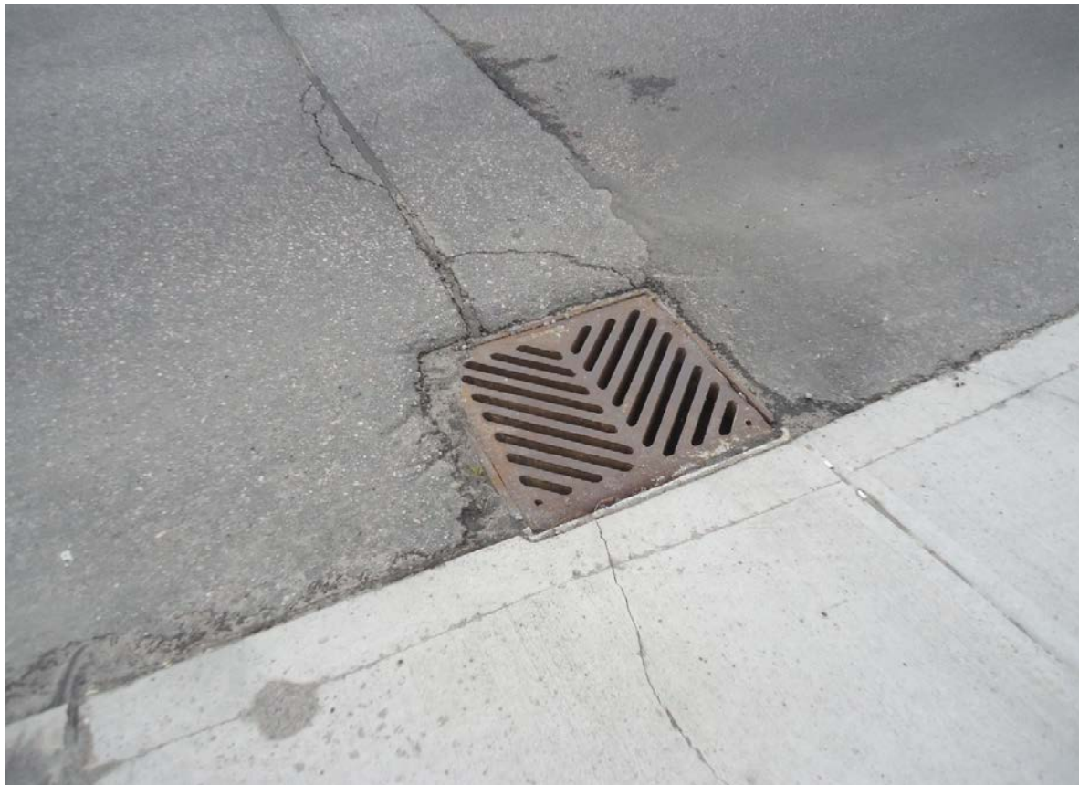
Description of Photo: Photo 31 - Catchbasin
