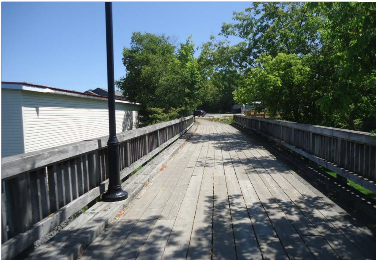
Description of Photo: Photo 1 - Wearing Surface
