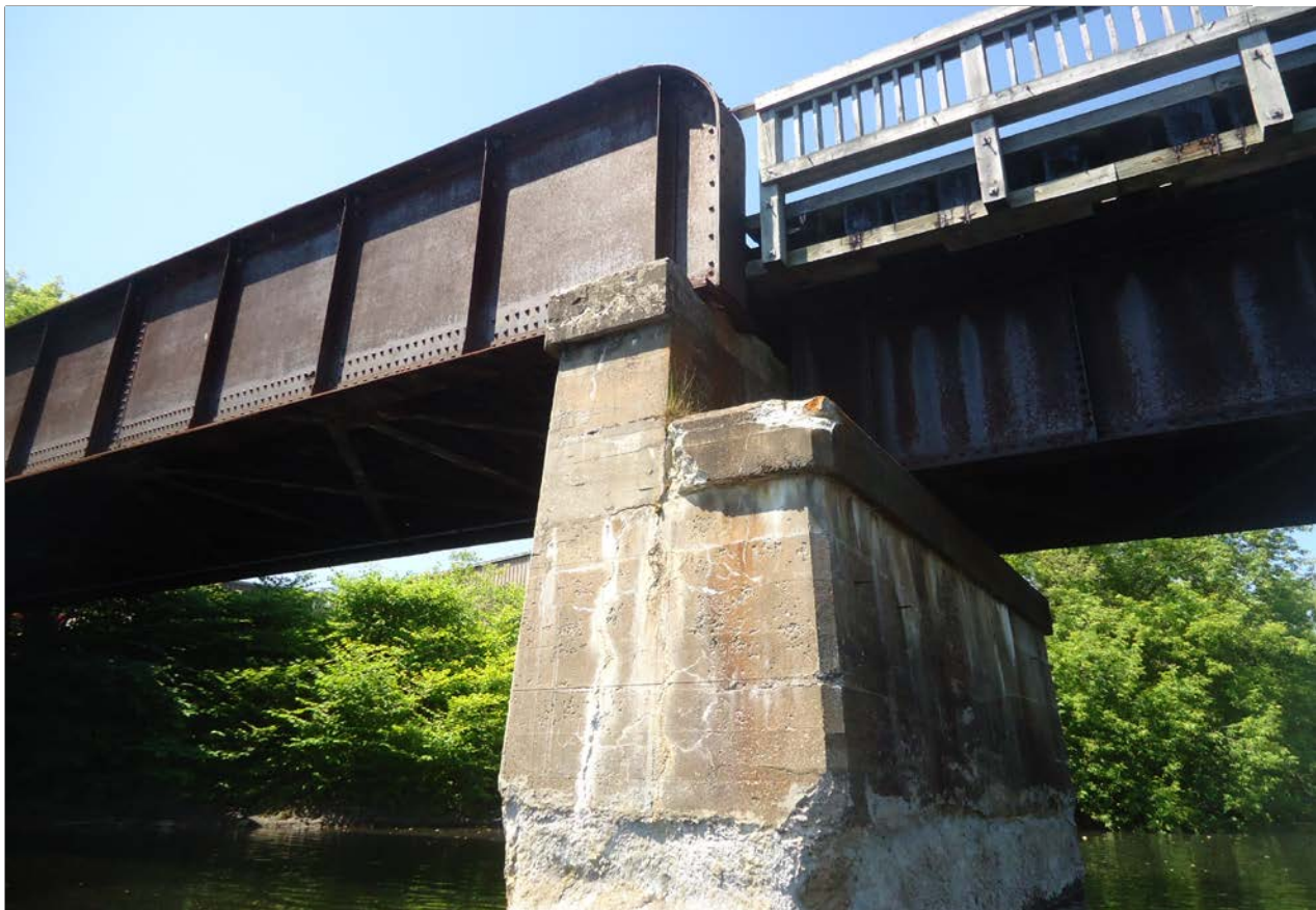
Description of Photo: Photo 60 - Steel through girder
