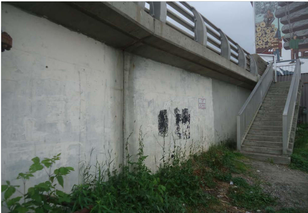
Description of Photo: Photo 59 - Northwest Wingwall
