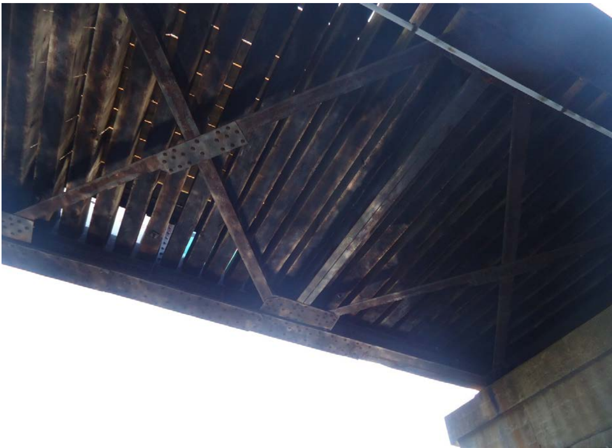
Description of Photo: Photo 65 - Steel Floor Beams
