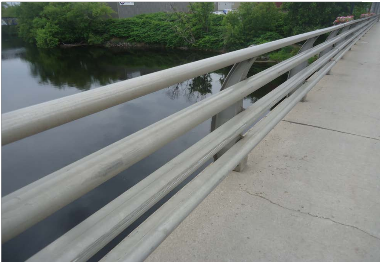
Description of Photo: Photo 24 - Railing
