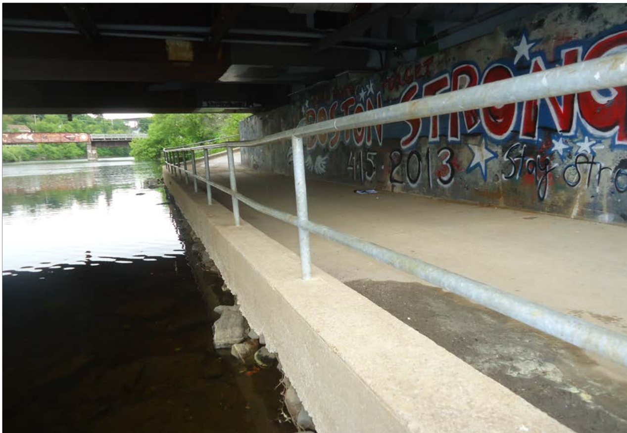
Description of Photo: Photo 69 - West Foundation
