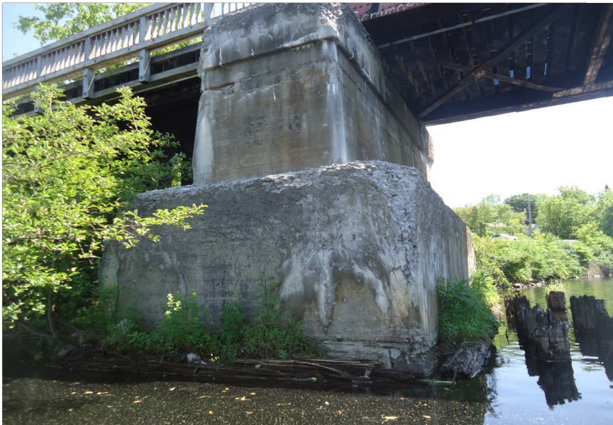
Description of Photo: Photo 54 - Pier Foundation
