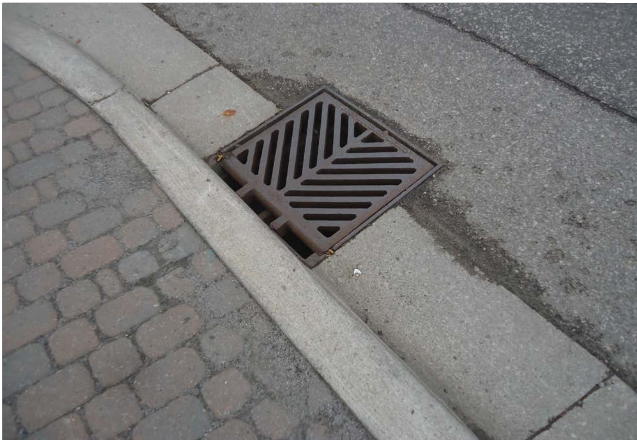
Description of Photo: Photo 78 - Approach Drainage
