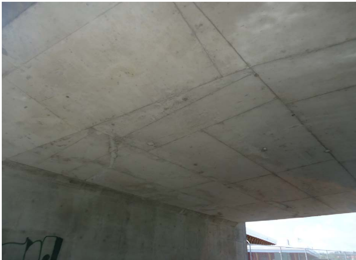
Description of Photo: Photo 5 - Soffit
