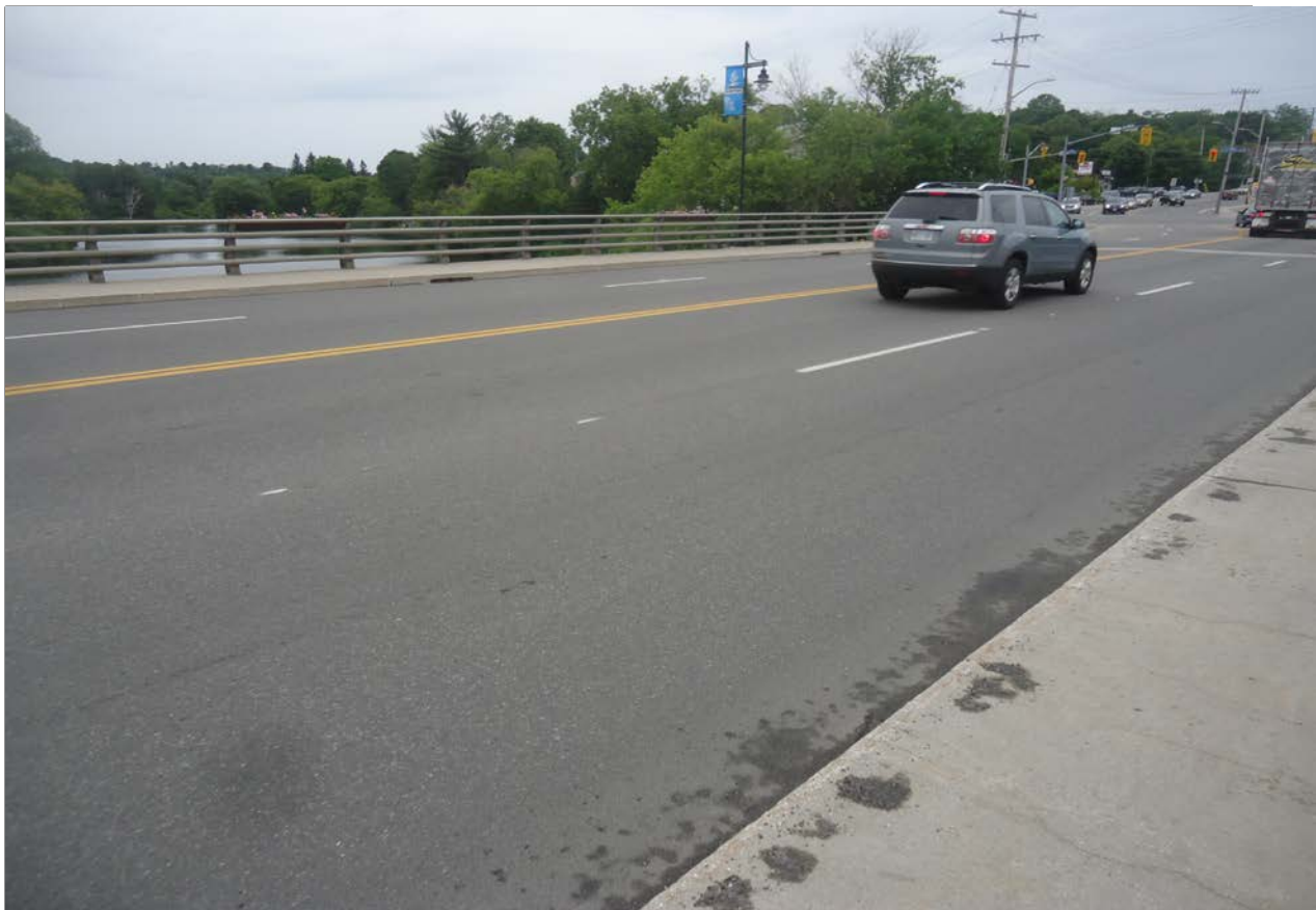
Description of Photo: Photo 1 - Wearing Surface
