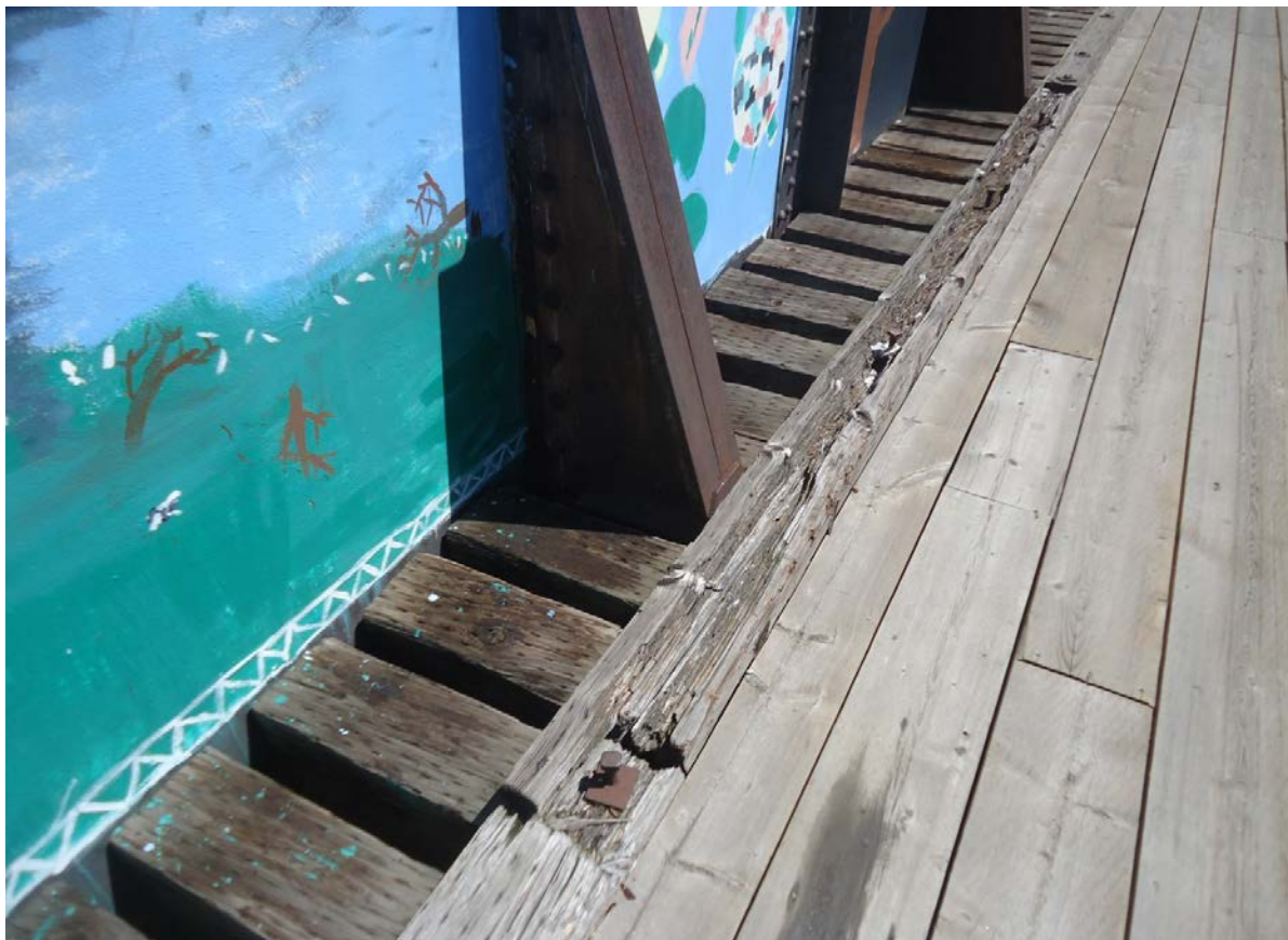
Description of Photo: Photo 7 - Timber Curb
