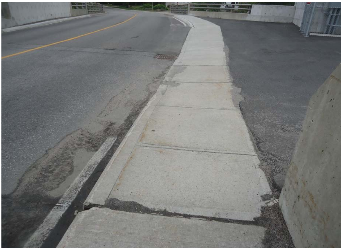
Description of Photo: Photo 35 - Northeast Approach Sidewalk
