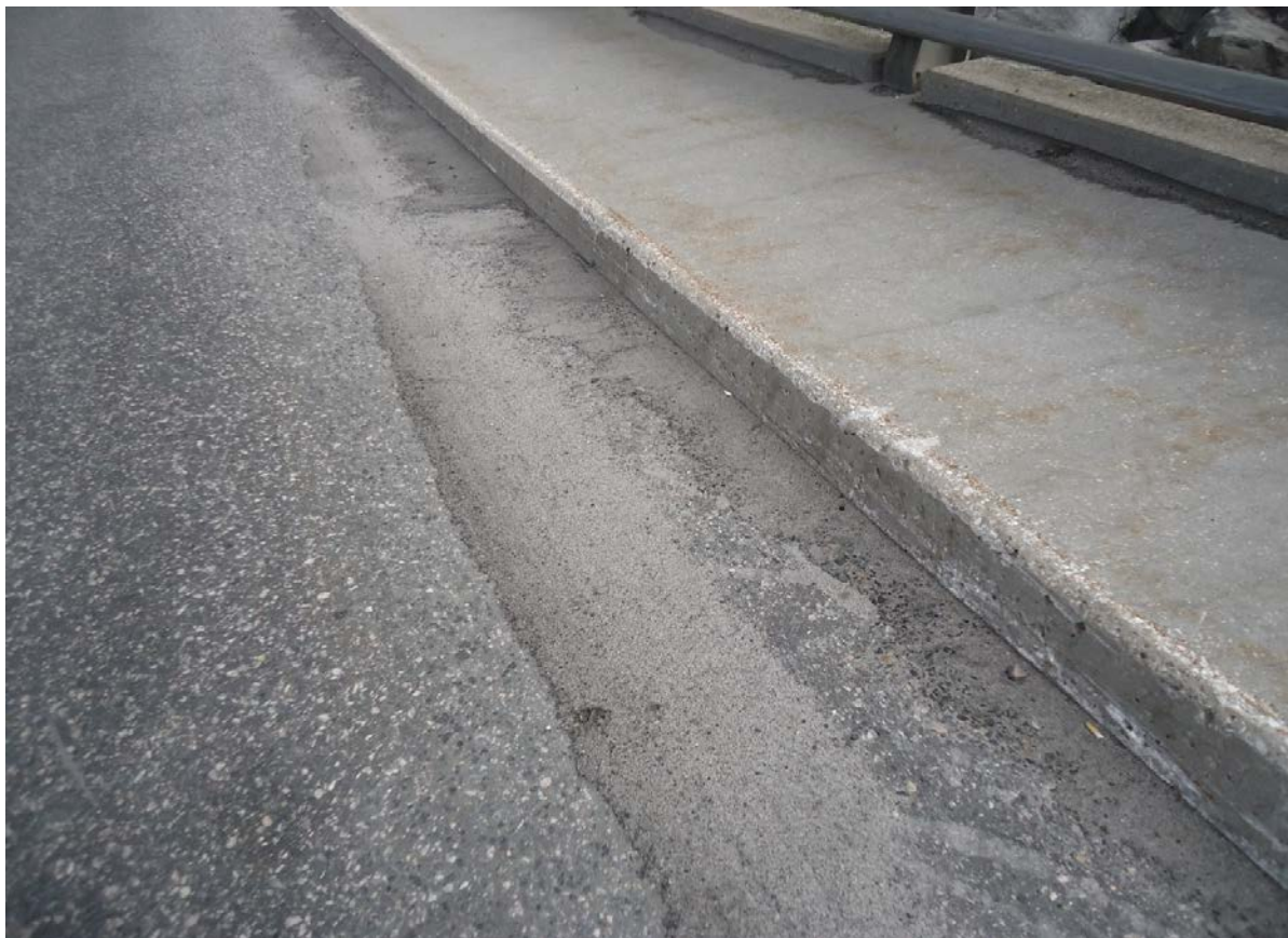
Description of Photo: Photo 8 - Sand Buildup
