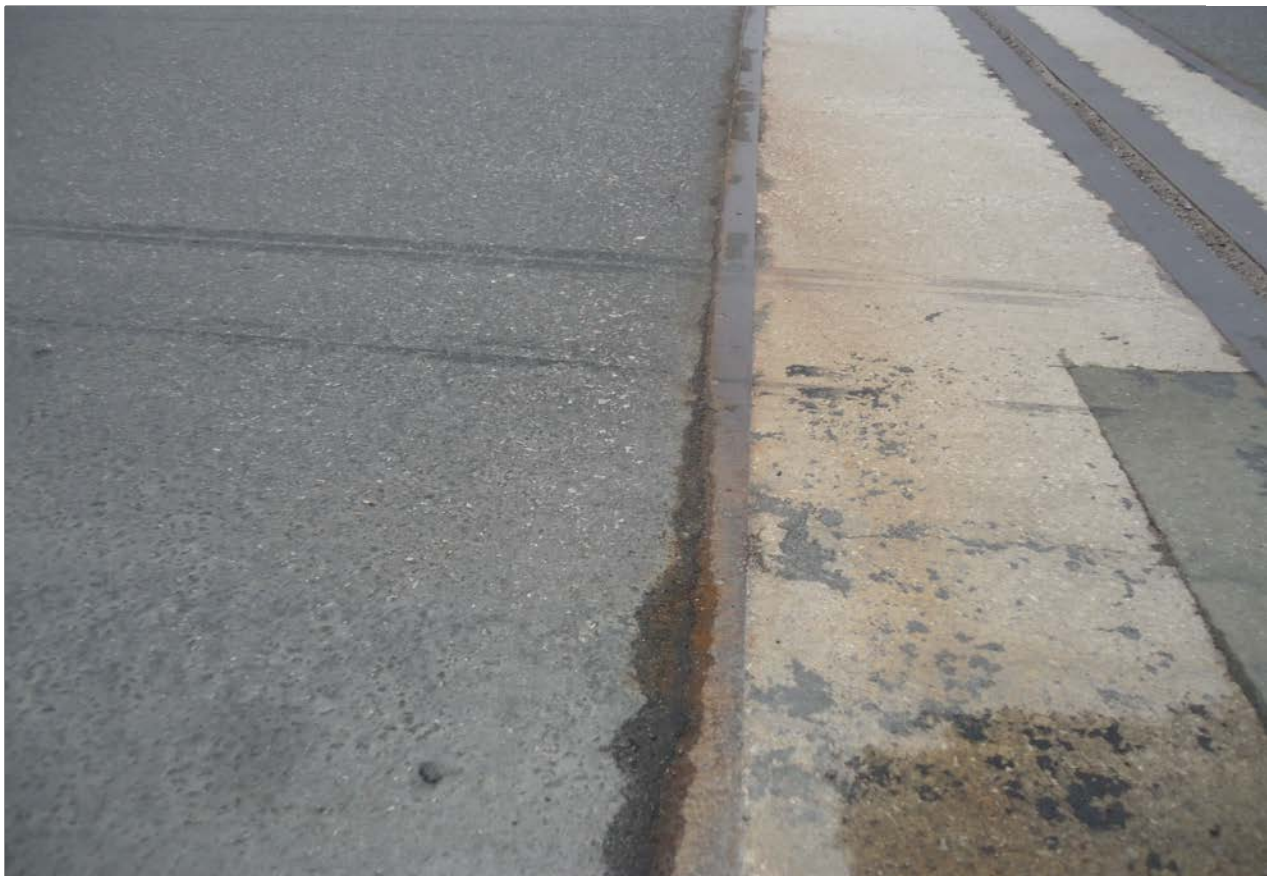
Description of Photo: Photo 18 - End Dam
