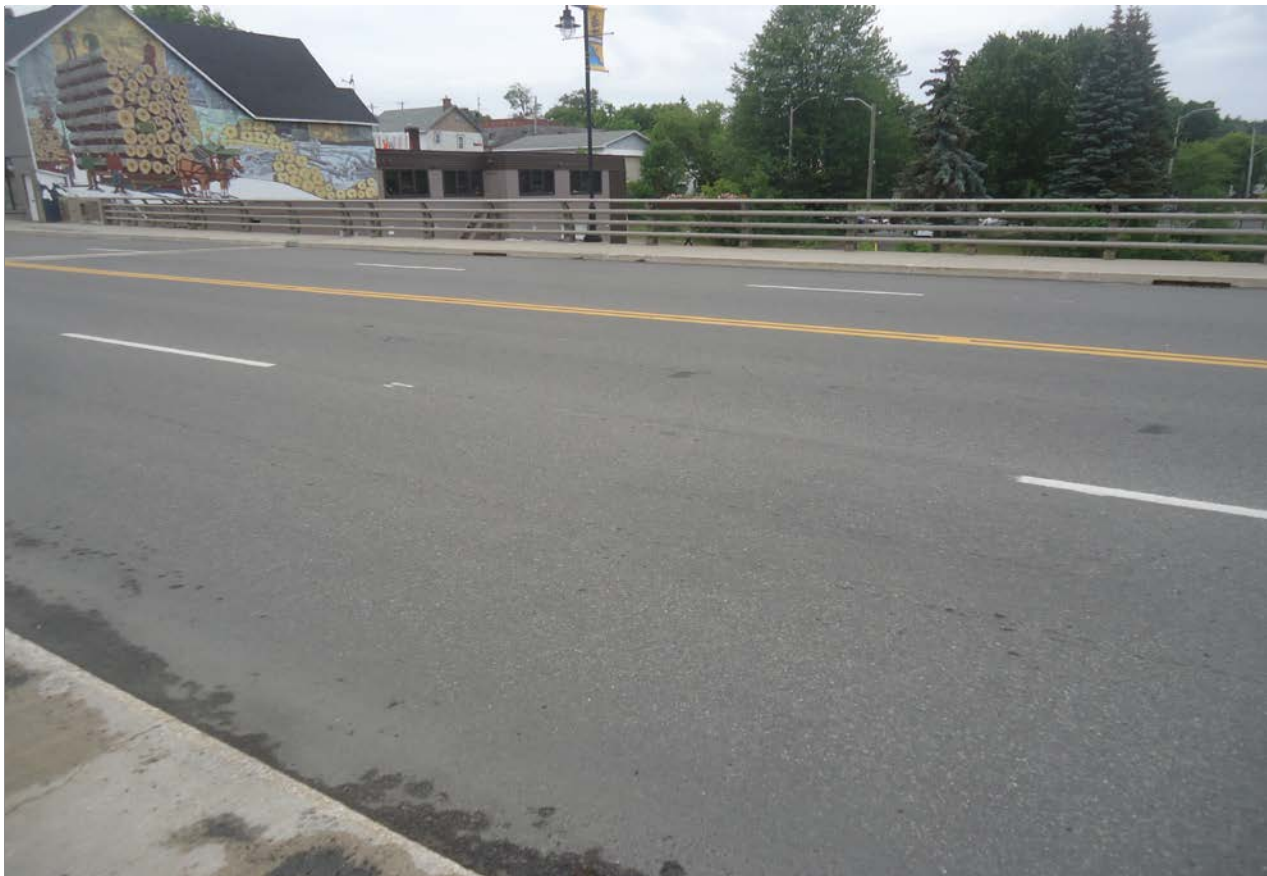
Description of Photo: Photo 2 - Deck Top
