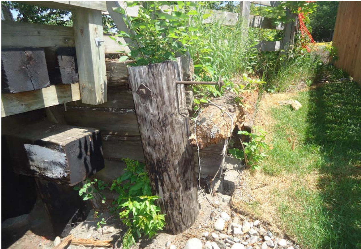
Description of Photo: Photo 22 - Southeast Wingwall
