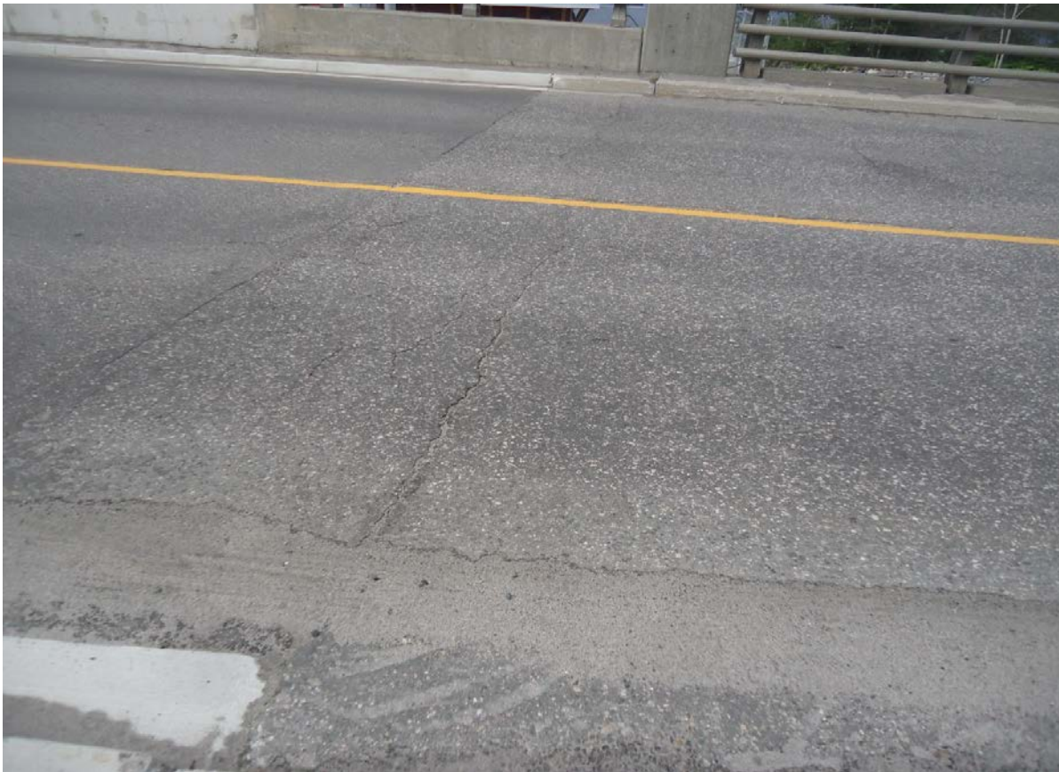
Description of Photo: Photo 4 - Deck Top
