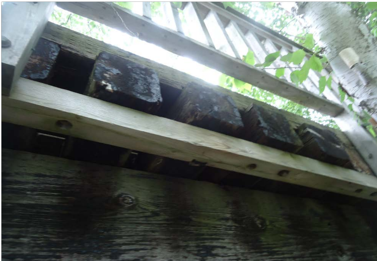
Description of Photo: Photo 16 - Stringers
