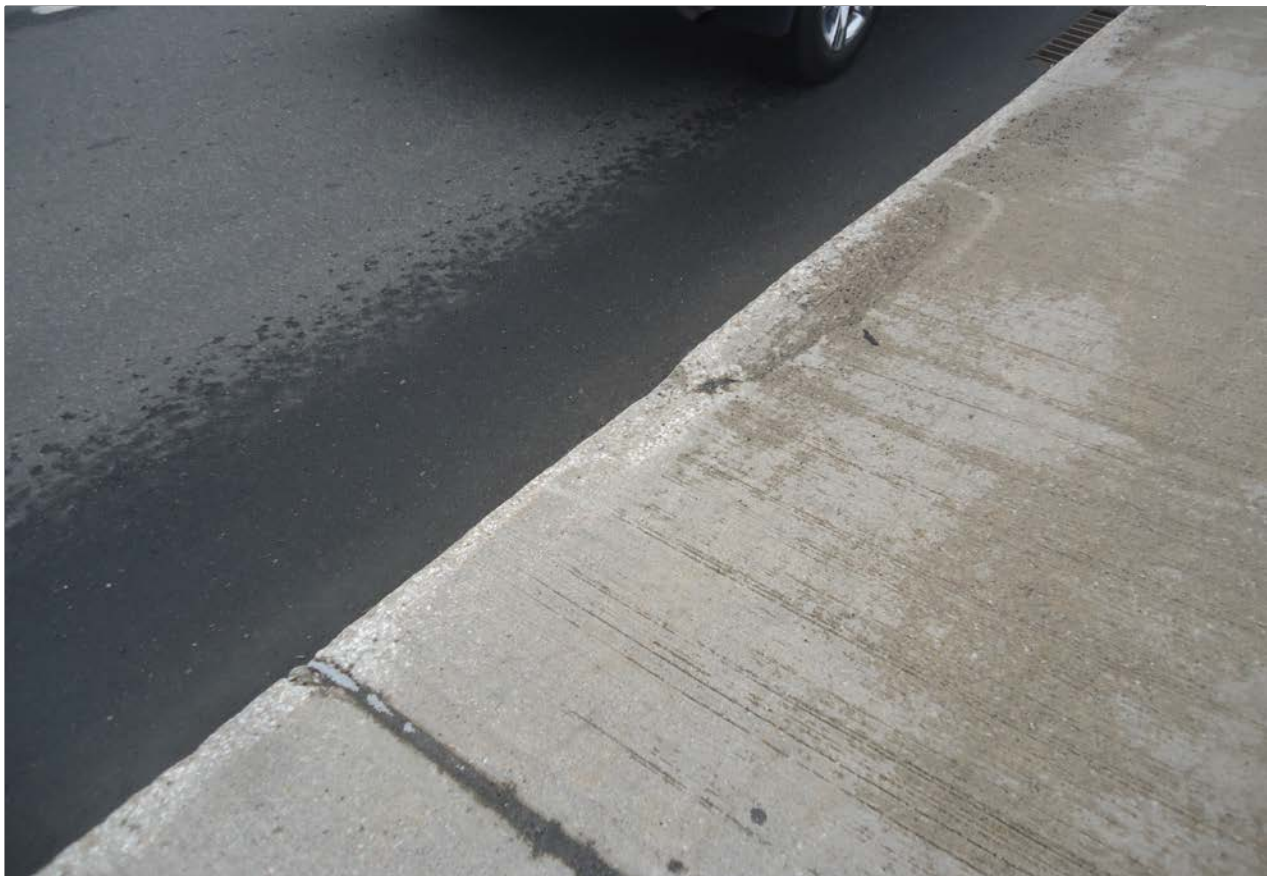
Description of Photo: Photo 80 - Approach Sidewalk
