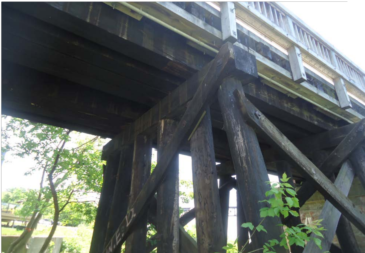
Description of Photo: Photo 41 - Pile Cap
