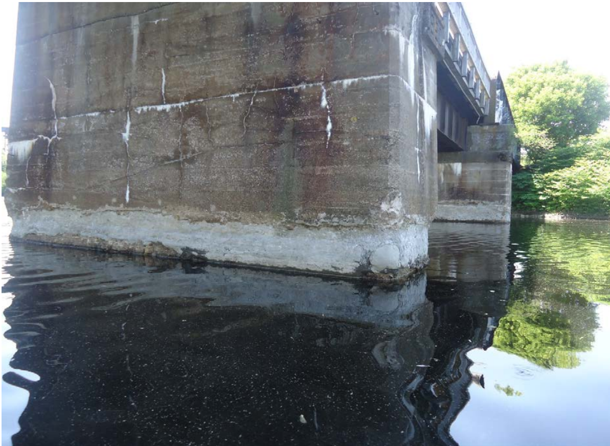
Description of Photo: Photo 49 - Pier
