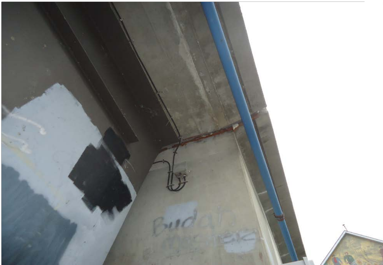
Description of Photo: Photo 8 - Soffit End
