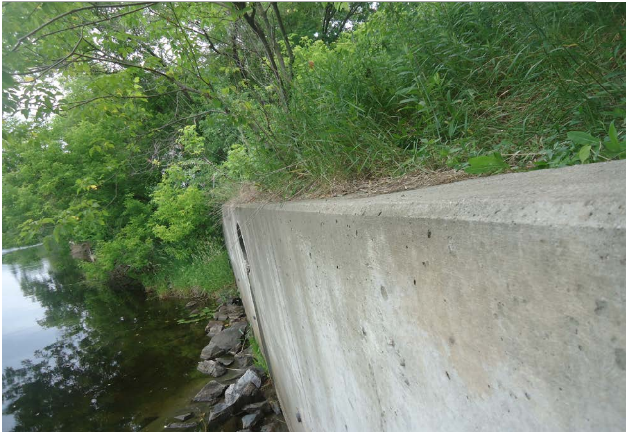
Description of Photo: Photo 72 - Embankment
