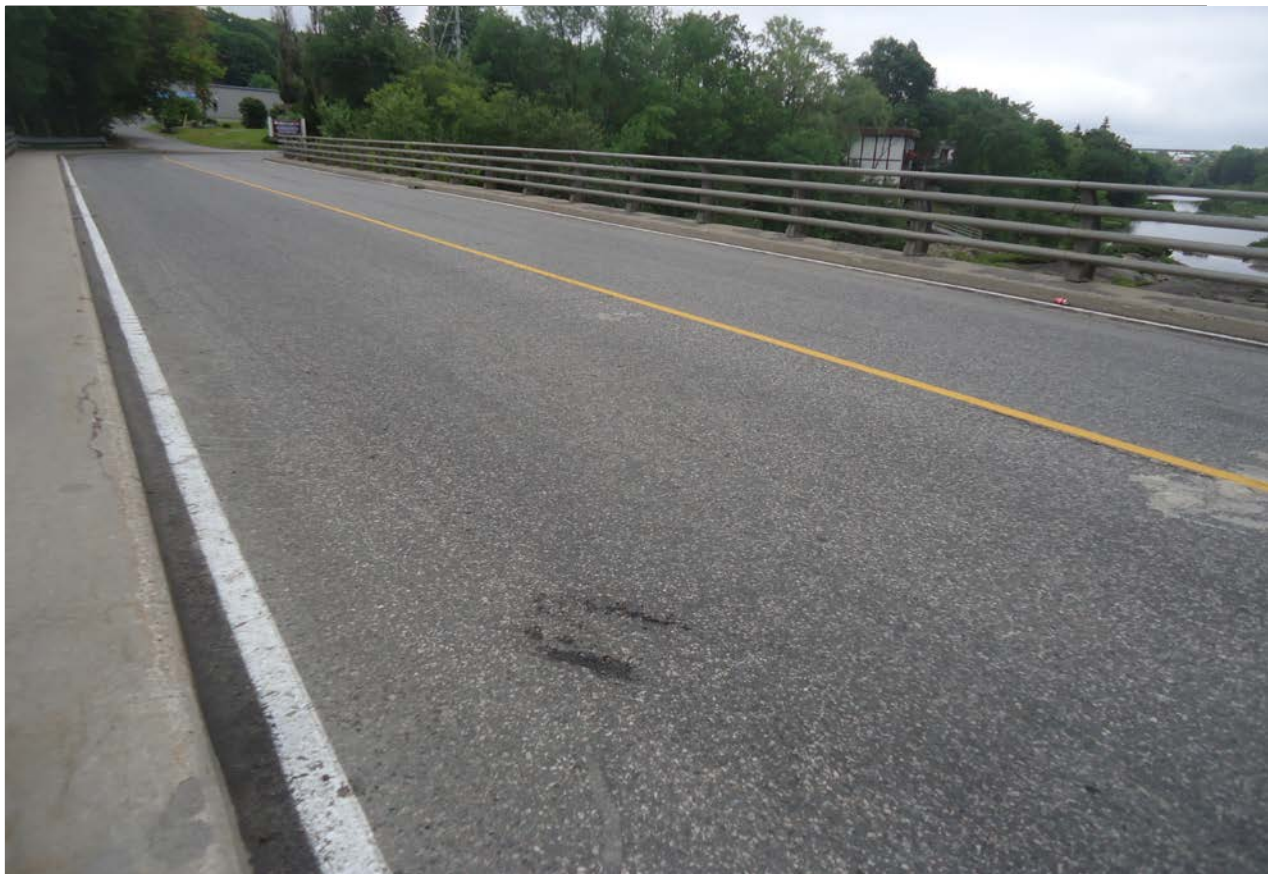
Description of Photo: Photo 1 - Wearing Surface
