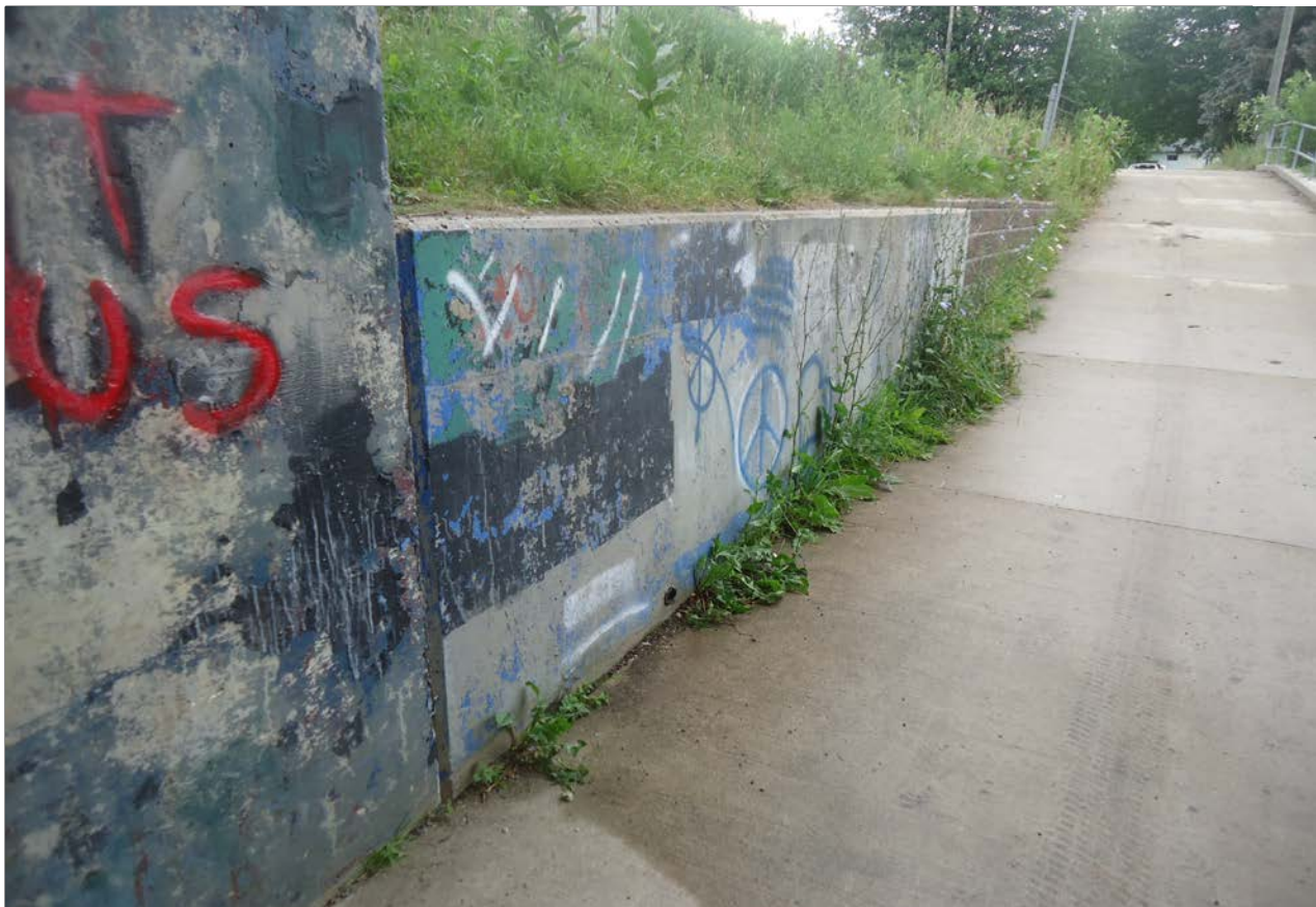
Description of Photo: Photo 62 - Retaining Wall
