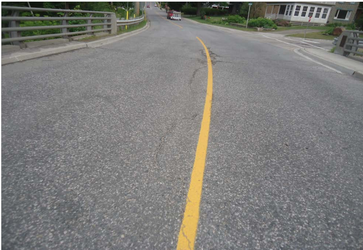
Description of Photo: Photo 1 - Wearing Surface
