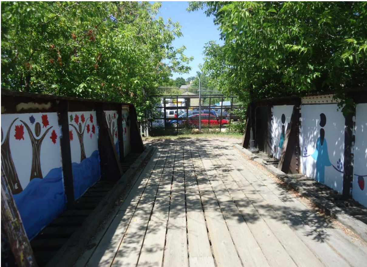
Description of Photo: Photo 29 - West Approach
