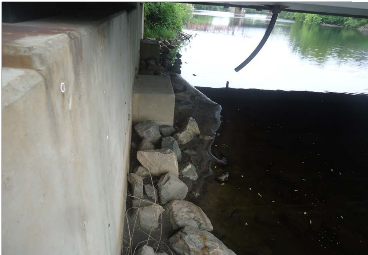
Description of Photo: Photo 70 - East Foundation
