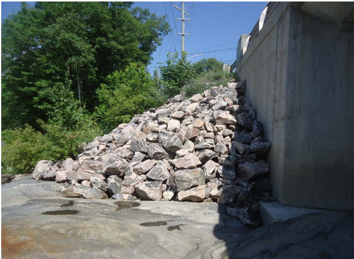
Description of Photo: Photo 23 - Northwest Embankment
