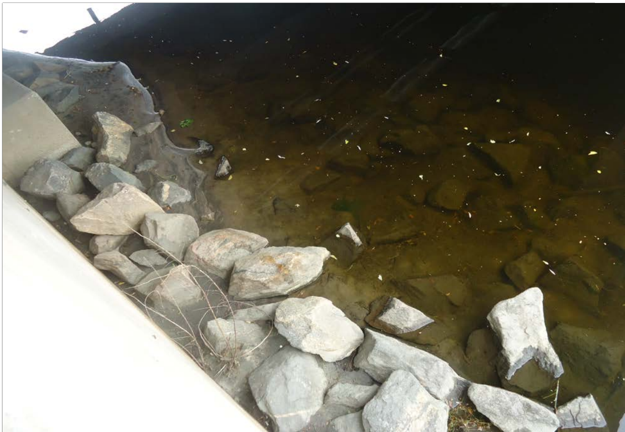
Description of Photo: Photo 74 - Slope Protection
