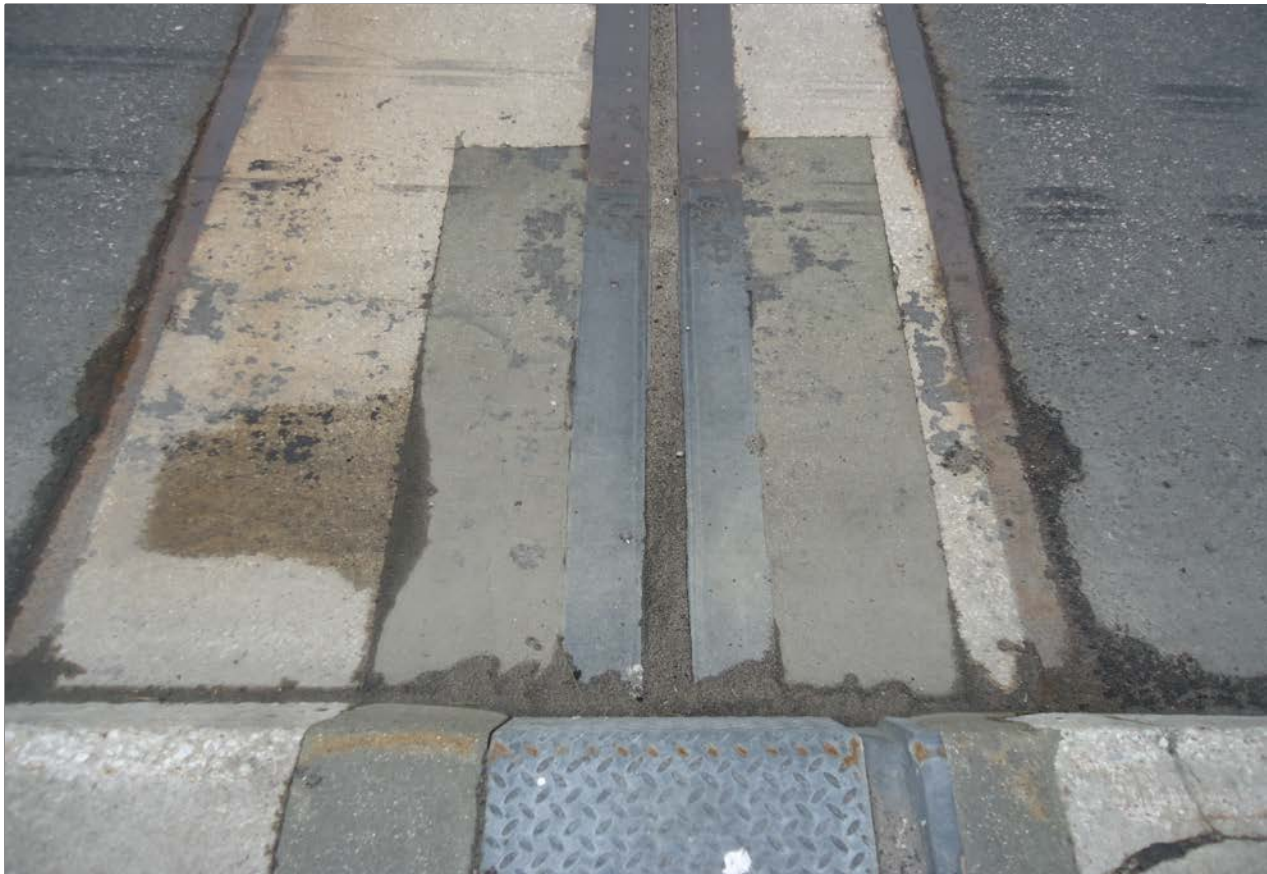
Description of Photo: Photo 16 - Expansion Joint
