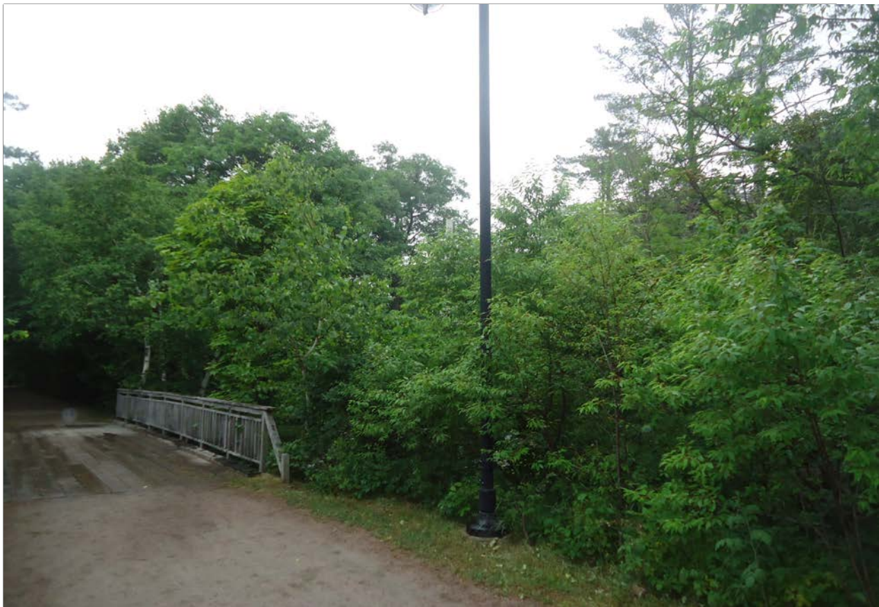
Description of Photo: Photo 26 - Embankment
