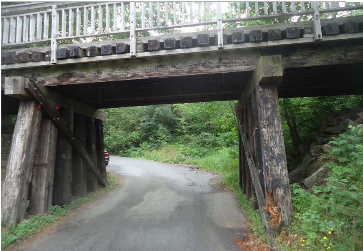
Description of Photo: Photo 13 - Floor Beams
