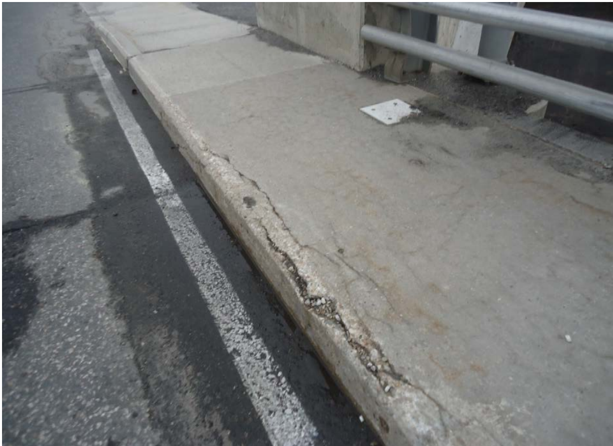
Description of Photo: Photo 7 - East Sidewalk
