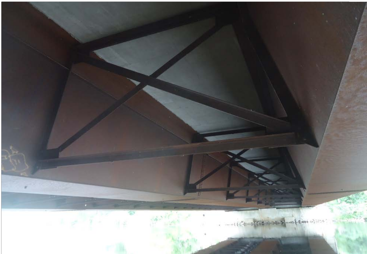
Description of Photo: Photo 13 - Soffit Interior
