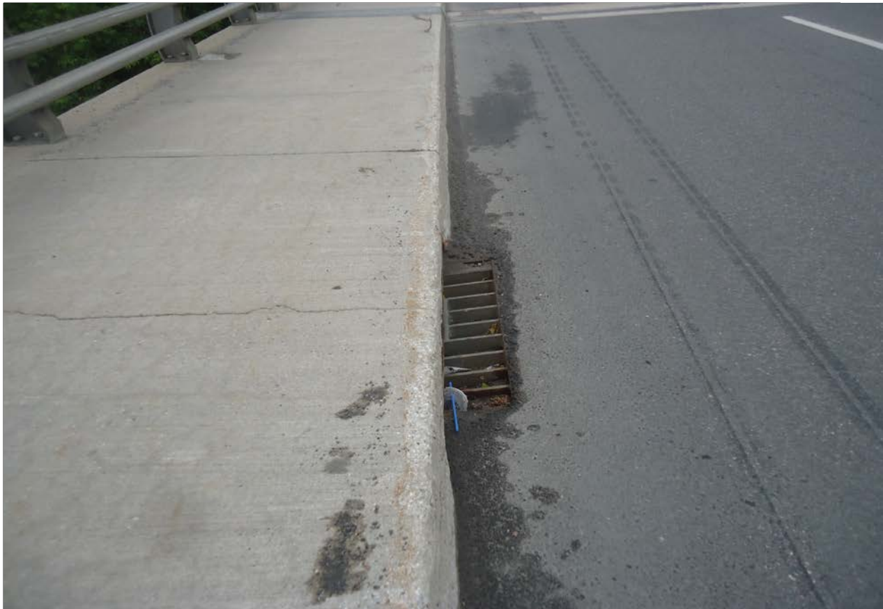
Description of Photo: Photo 77 - Approach Slabs
