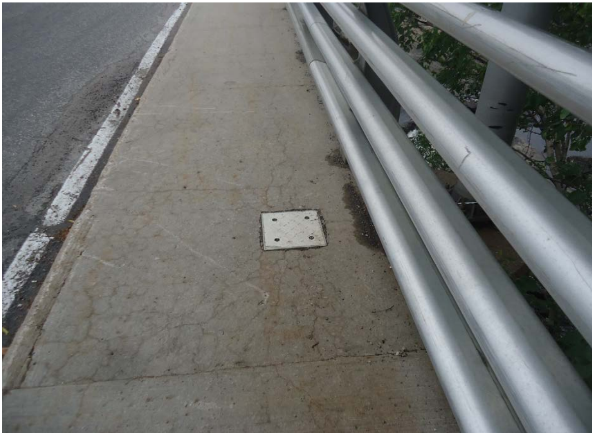
Description of Photo: Photo 37 - Utility Cover
