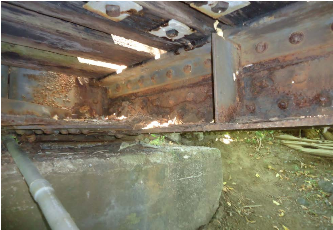
Description of Photo: Photo 13 - Steel Coating
