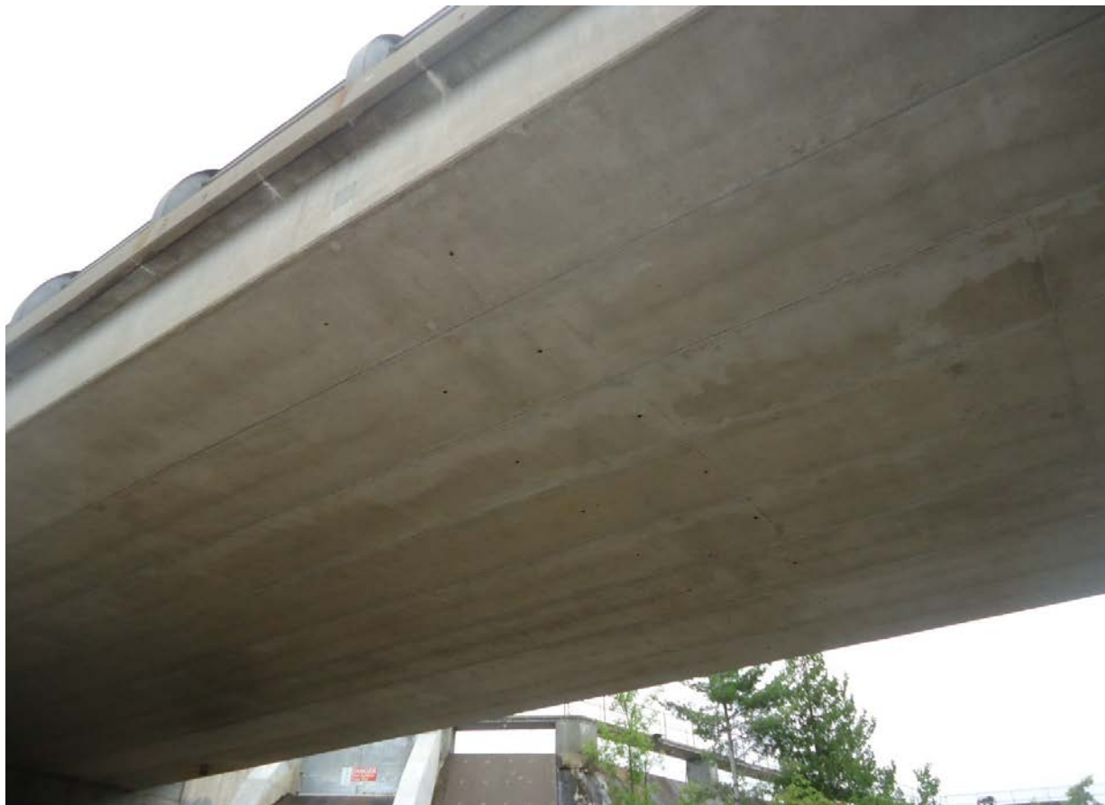
Description of Photo: Photo 42 - Underside of Girders
