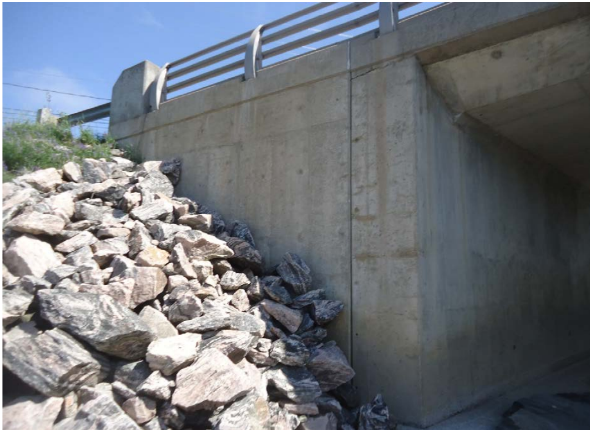
Description of Photo: Photo 17 - Northwest Wingwall
