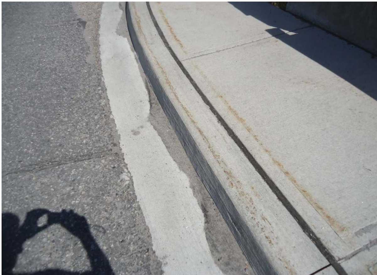
Description of Photo: Photo 32 - Approach Curb
