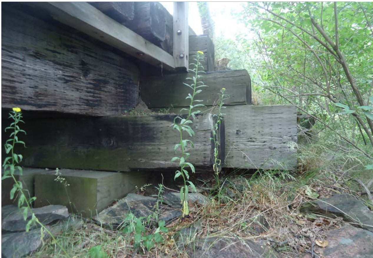
Description of Photo: Photo 18 - Abutment
