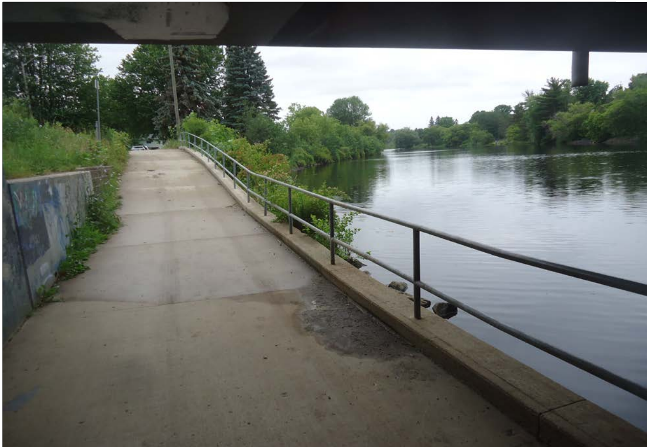
Description of Photo: Photo 66 - Steel Handrail
