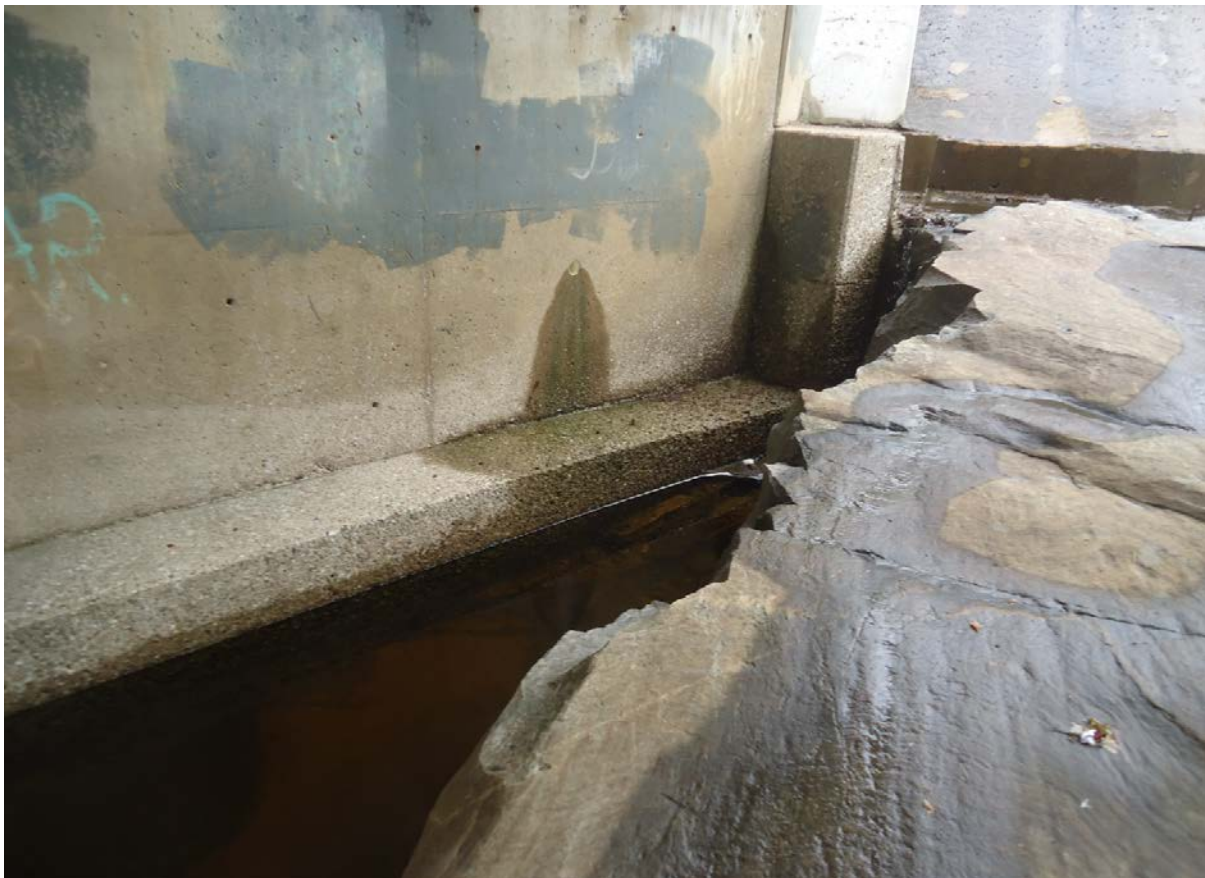
Description of Photo: Photo 22 - North Foundation
