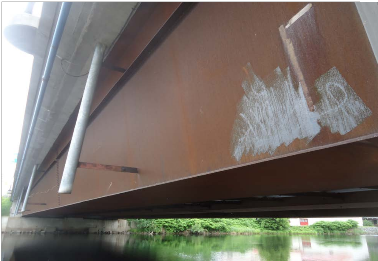
Description of Photo: Photo 31 - Girder End
