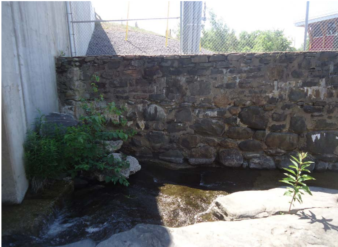
Description of Photo: Photo 25 - Southwest Retaining Wall
