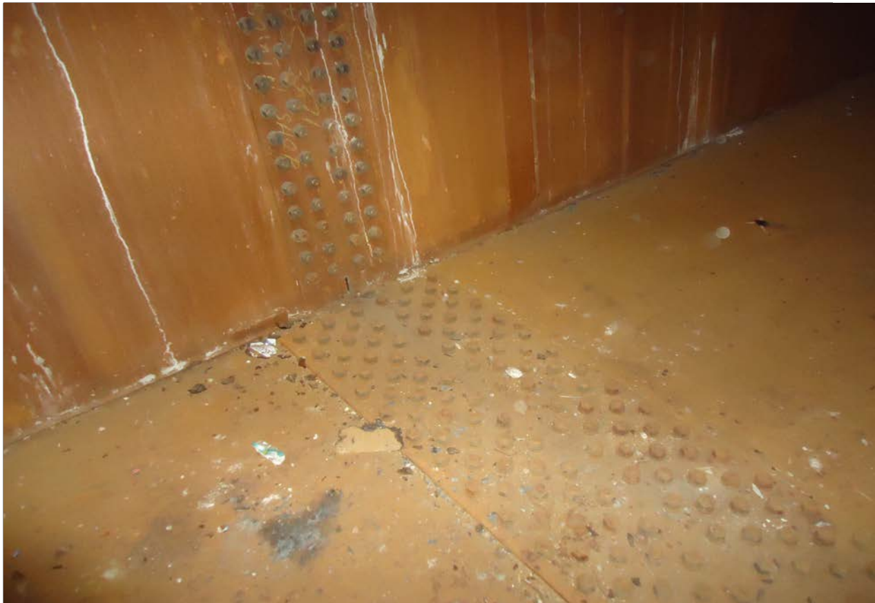
Description of Photo: Photo 43 - Girder Mid Inside
