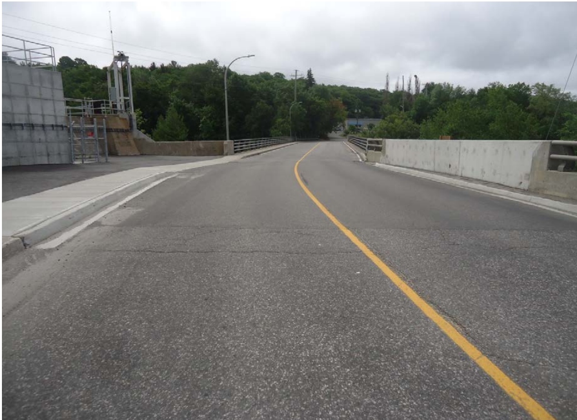
Description of Photo: Photo 29 - South Approach Surface
