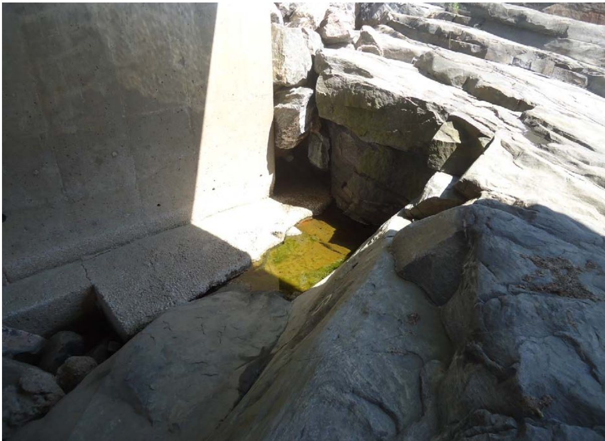
Description of Photo: Photo 20 - North Foundation
