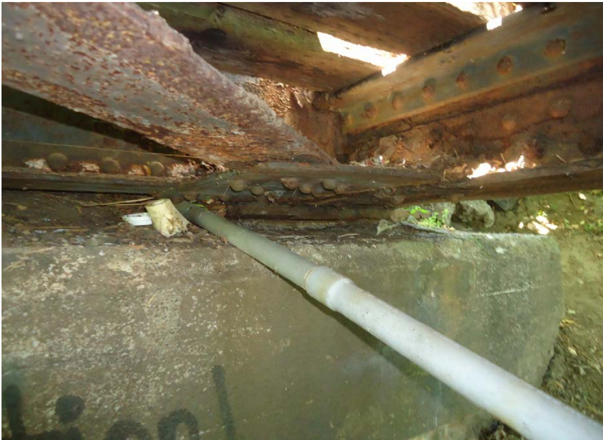
Description of Photo: Photo 19 - West Abutment Bearings
