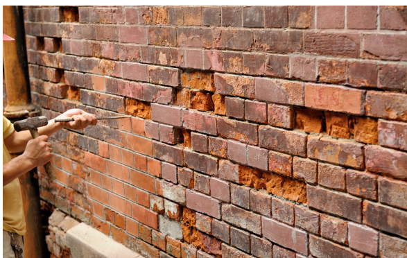
Repairing and repainting old brick walls
