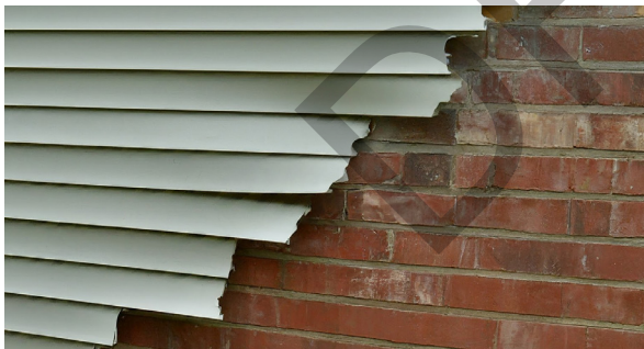
Removing vinyl to reveal brick below
