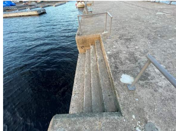
114- Structure D – West Steps (looking North), Stn 0+222 to 0+226
