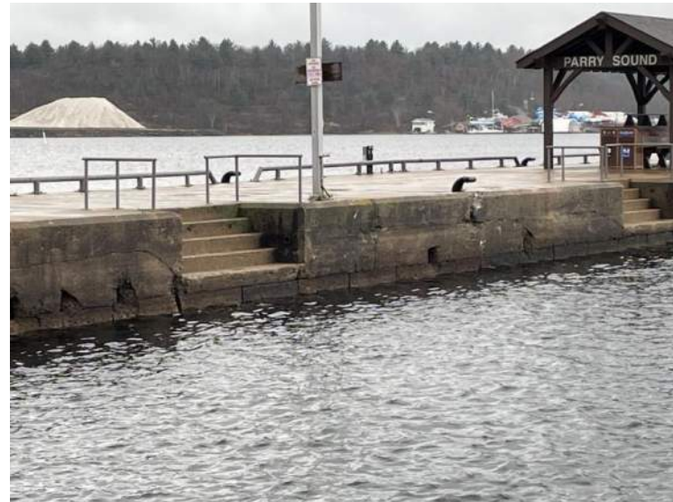
96- Structure D – West Face, Stn 0+220 to 0+240
