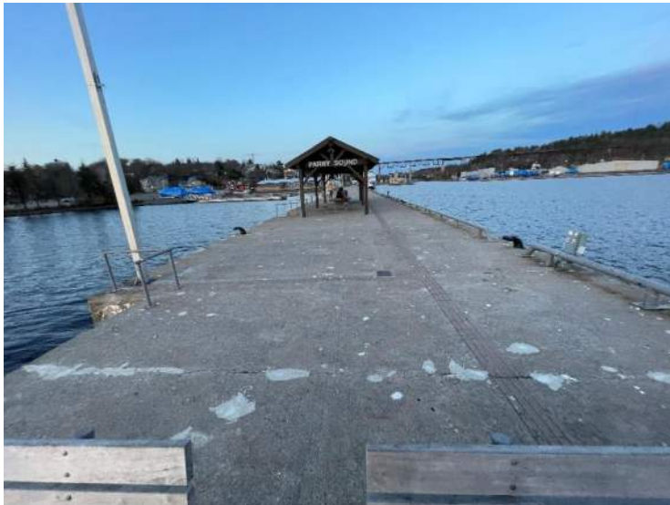
143- Structure D – Concrete Deck (looking North), Stn 0+272
