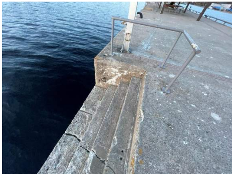
139- Structure D – West Steps (looking North), Stn 0+268 to 0+272
