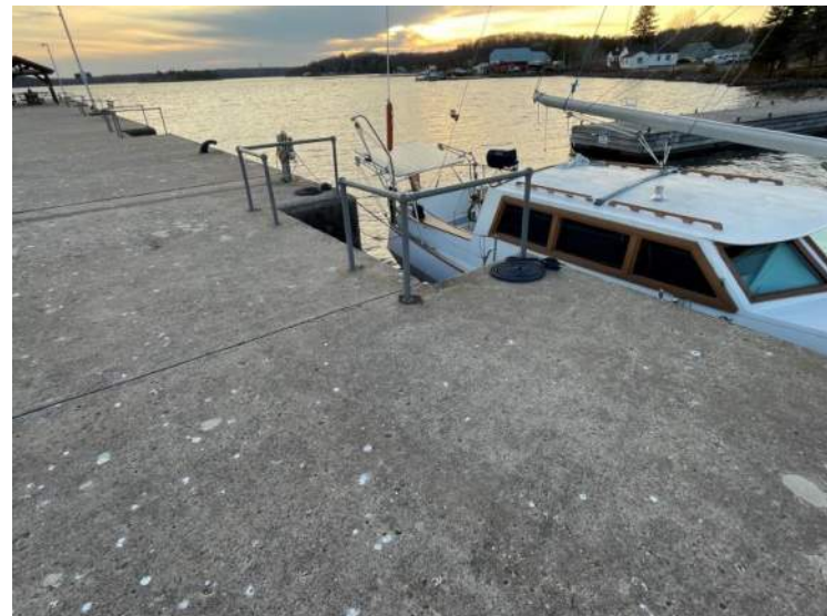
92- Structure D – West Steps, Stn 0+192 to 0+196
