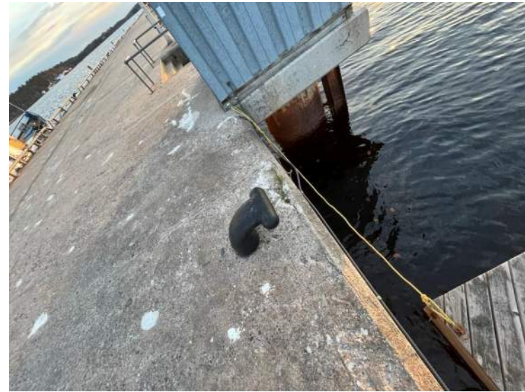
54- Structure D – West Bollard, Stn 0+141
