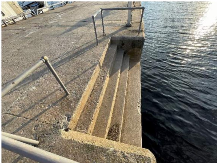
59- Structure D – West Steps (Looking South), Stn 0+146 to 0+150
