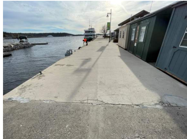
6- Structure B – Newer Concrete Deck Transition, Stn 0+026
