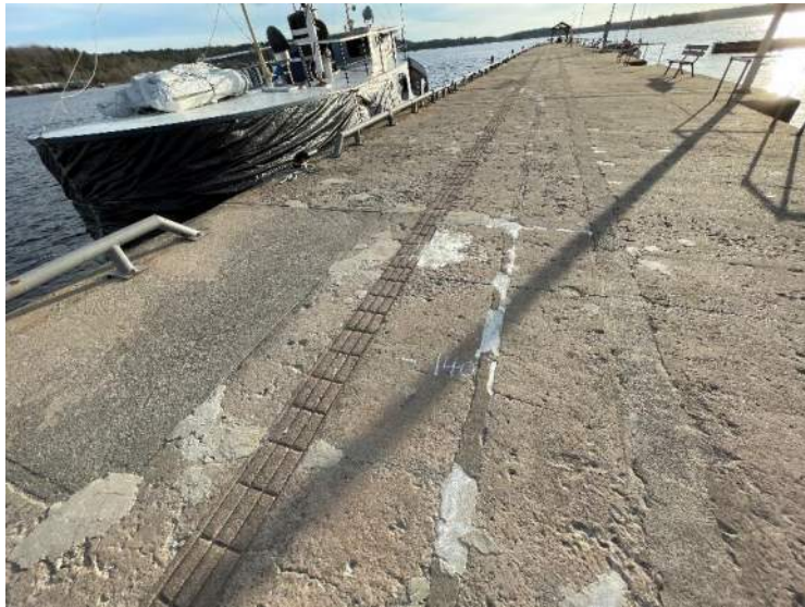
57- Structure D – Buried East Slipway, Stn 0+139 to 0+141
