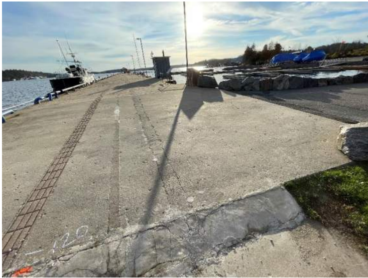
37- Structure D – Newer Concrete Deck, Stn 0+117.8 to 0+126
