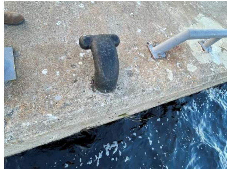
122- Structure D – East Bollard, Stn 0+236
