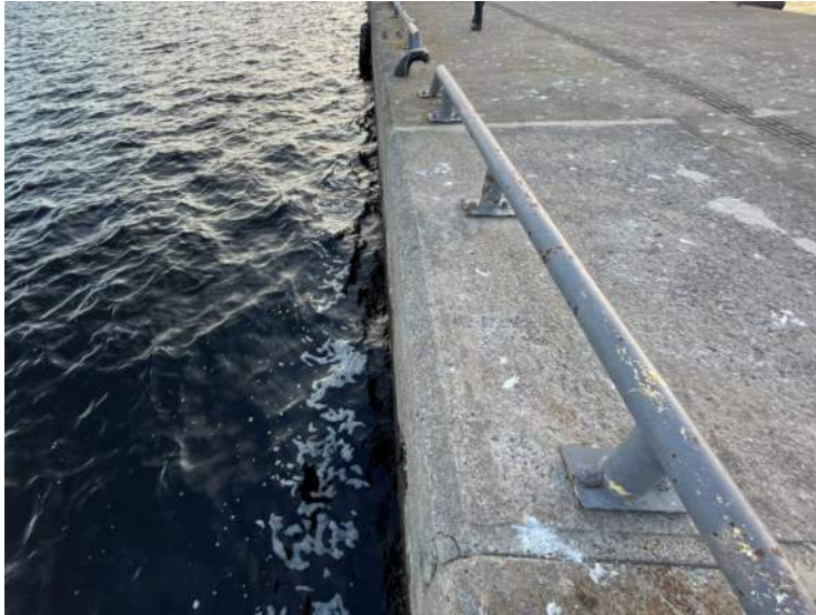
101- Structure D – Buried East Slipway, 0+200 to 0+203
