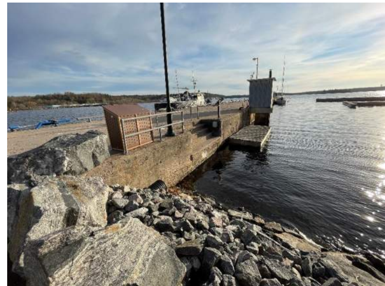
44- Structure D – West Face (looking South from West Shoreline)
