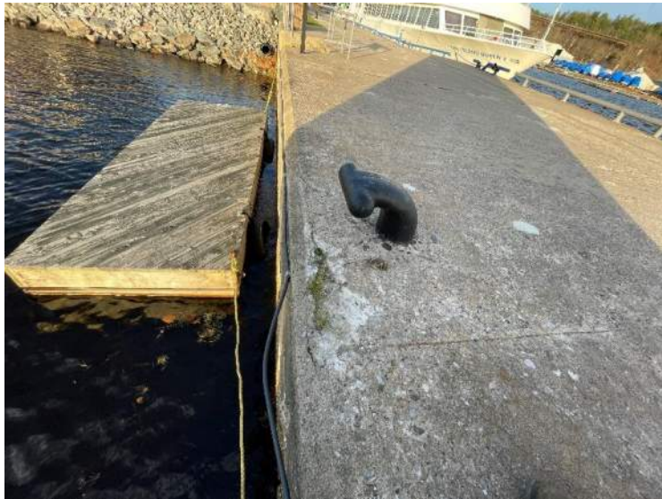
53- Structure D – West Bollard, Stn 0+141
