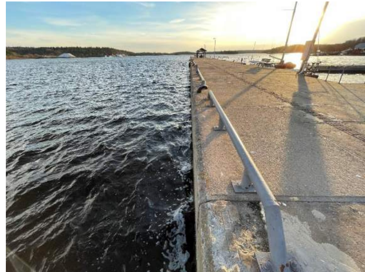
78- Structure D – Buried East Slipway, Stn 0+169 to 0+172
