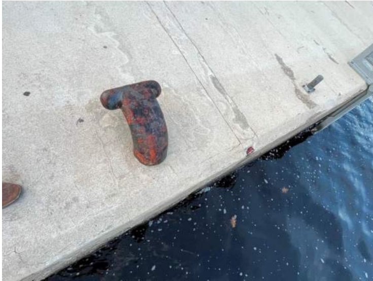
9- Structure B – East Bollard, Stn 0+036
