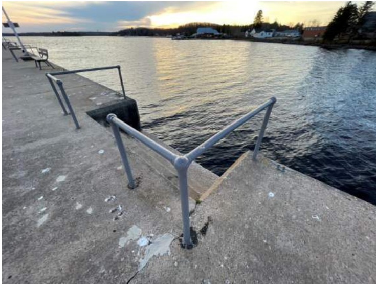
105- Structure D – West Steps, Stn 0+206 to 0+211
