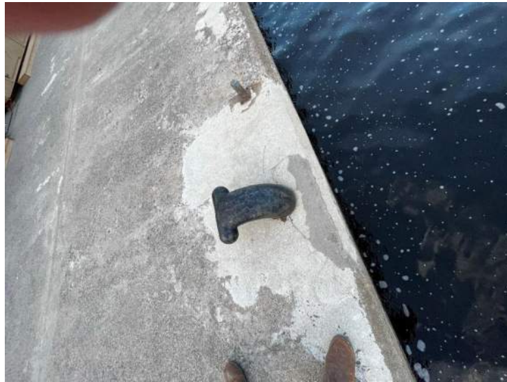
5- Structure B – East Bollard, Stn 0+023
