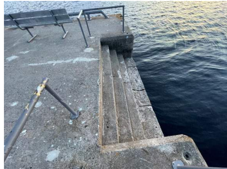
138- Structure D – West Steps (looking South), Stn 0+268 to 0+272
