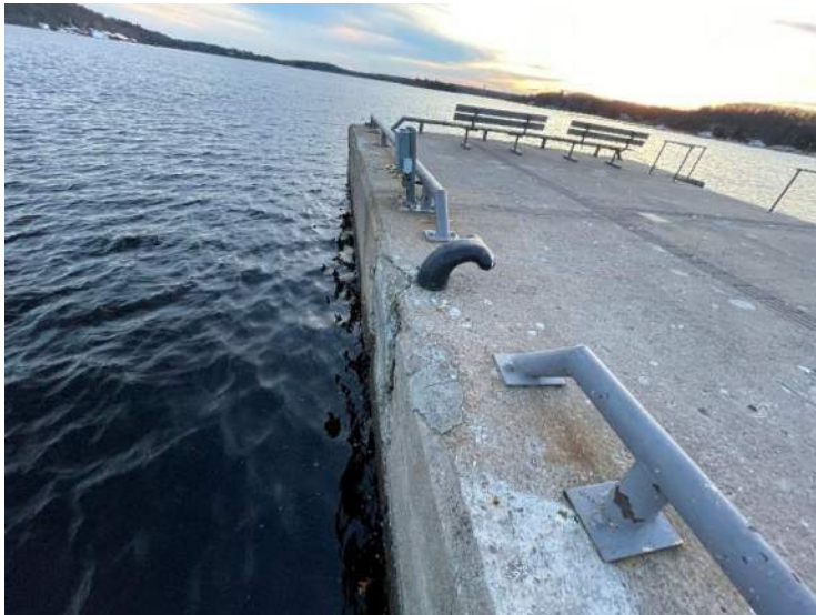
135- Structure D – East Bollard, Stn 0+266
