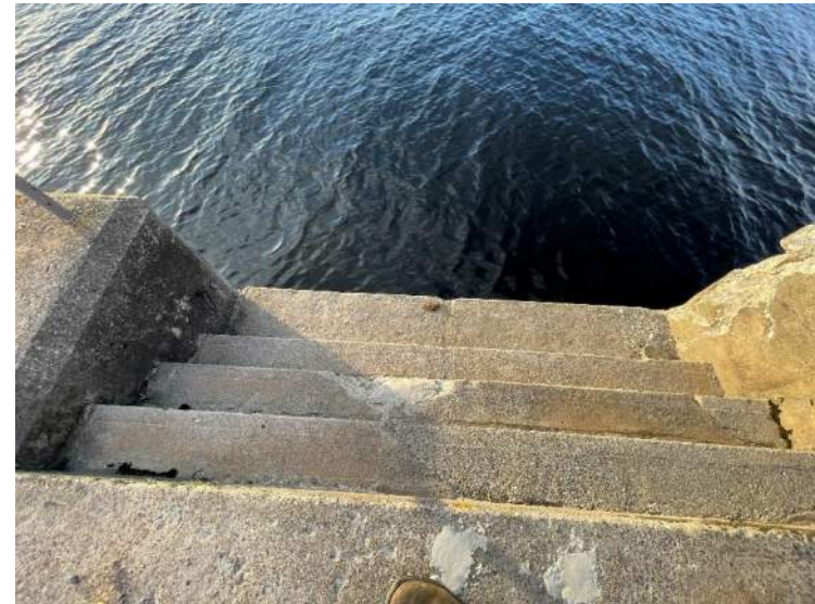
72- Structure D – West Steps, Stn 0+161 to 0+164
