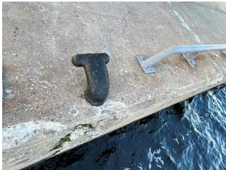
127- Structure D – East Bollard, Stn 0+251
