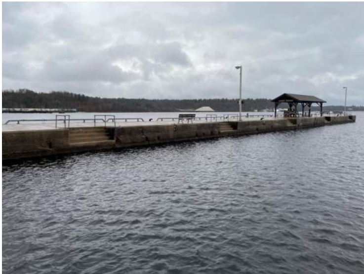
95- Structure D – West Face, Stn 0+200 to 0+273.3
