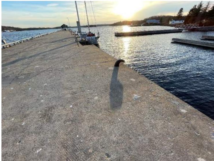
79- Structure D – West Bollard, Stn 0+170
