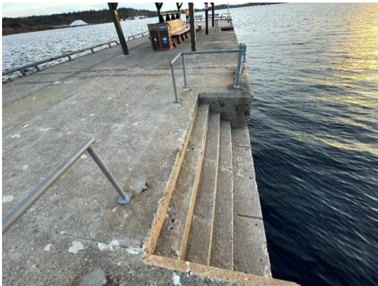
123- Structure D – West Steps (looking South), Stn 0+238 to 0+242
