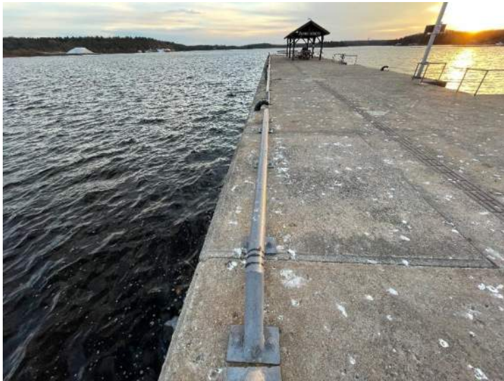
109- Structure D – Buried East Slipway, Stn 0+216 to 0+218
