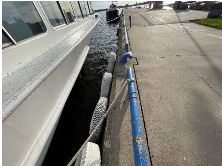
33- Structure C – East Bollard, Stn 0+113
