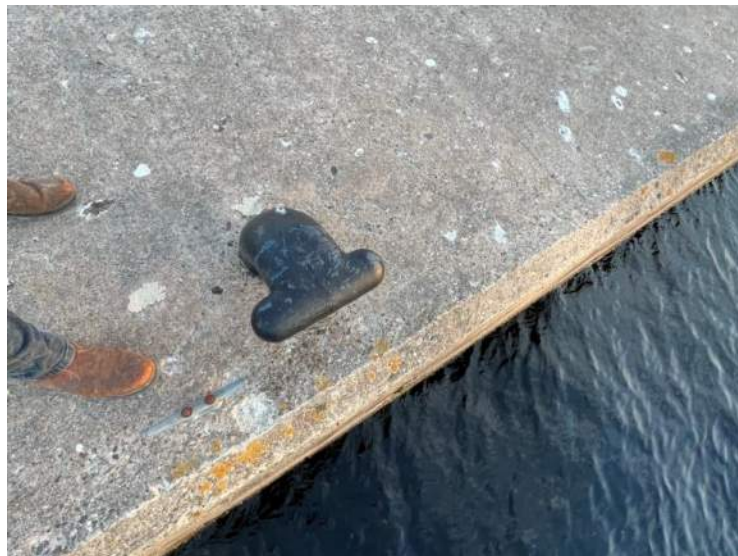
99- Structure D – West Bollard, Stn 0+201
