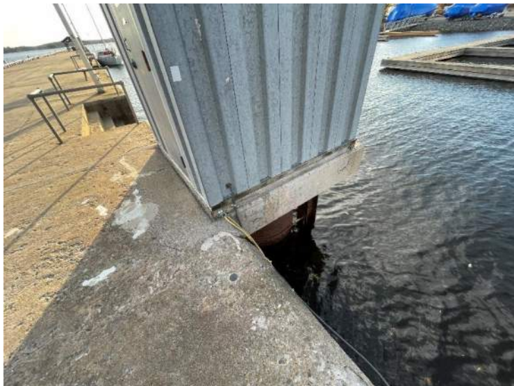
51- Structure D – Water Gage Station Slab (North Face), Stn 0+144
