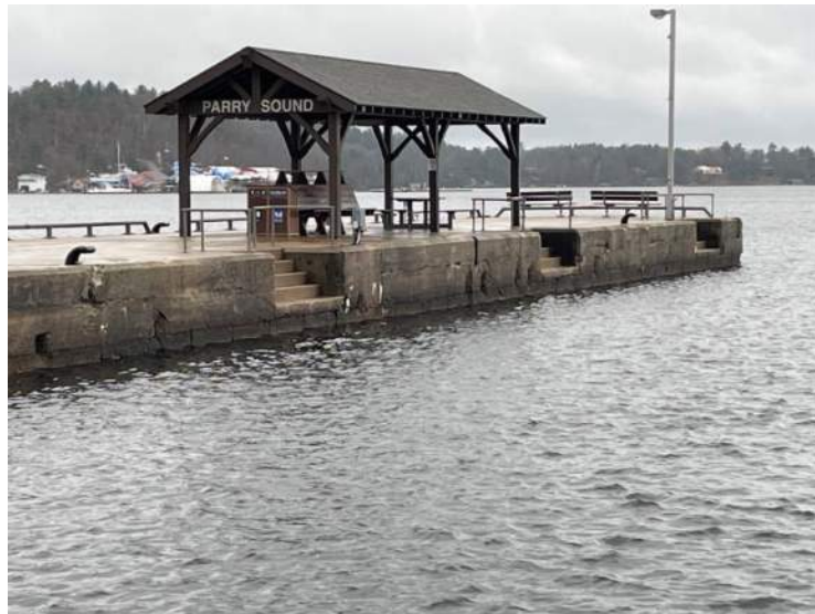
97- Structure D – West Face, Stn 0+230 to 0+273.3
