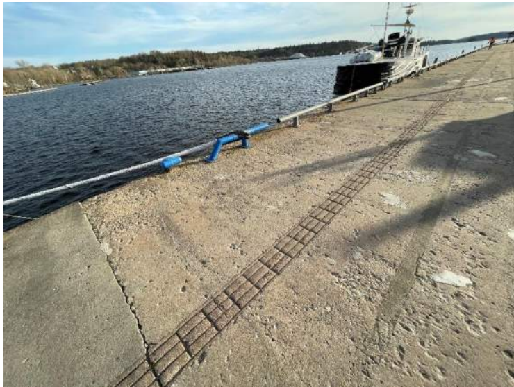
41- Structure D – Section of Curb Rail removed, Stn 0+131
