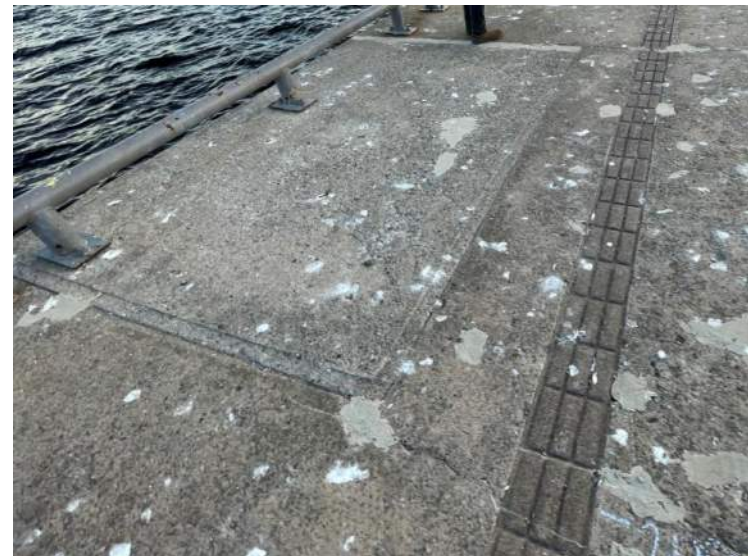
100- Structure D – Buried East Slipway, 0+200 to 0+203
