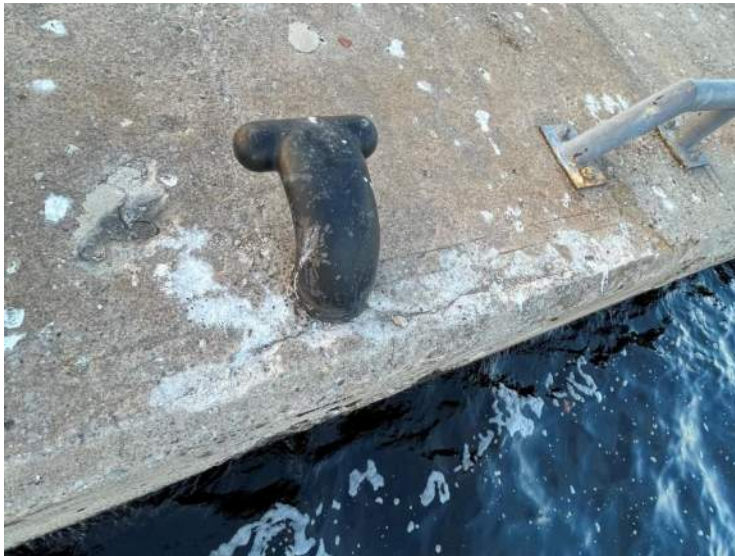
111- Structure D – East Bollard, Stn 0+221
