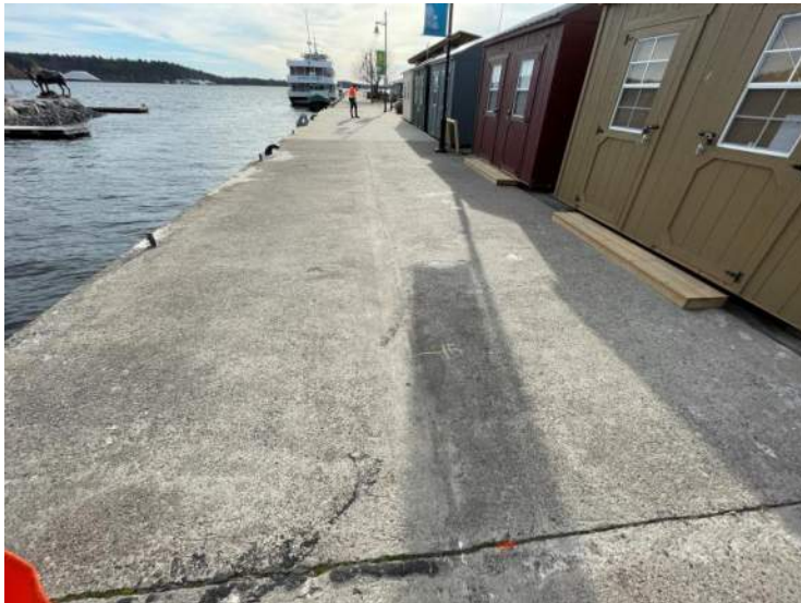
3- Structure A – Concrete Deck
