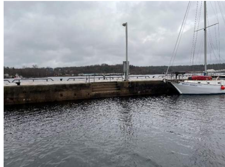
64- Structure D – West Face, Stn 0+169 to 0+189
