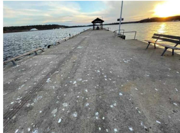
108- Structure D – Concrete Deck, Stn 0+215
