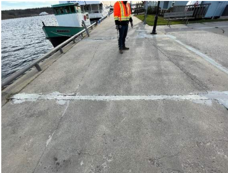
17- Structure C – Buried Conduit, Stn 0+064
