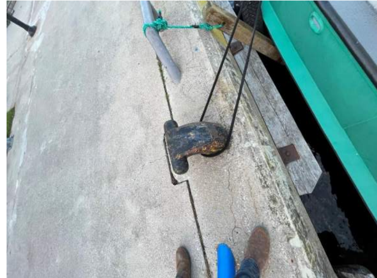
22- Structure C – East Bollard, Stn 0+076
