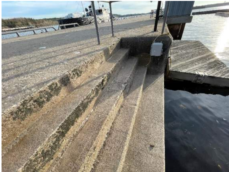
49- Structure D – West Steps (Looking South), Stn 0+131 to 0+134
