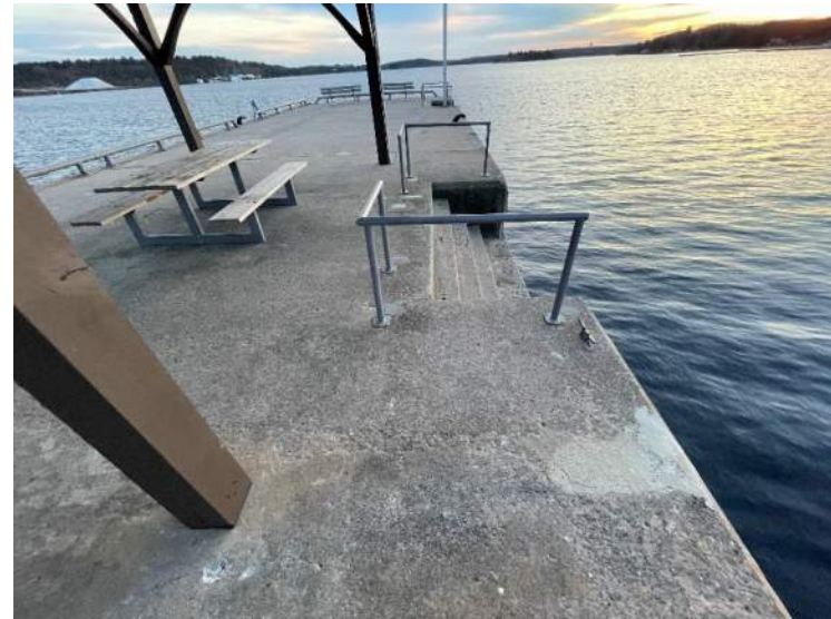
130- Structure D – West Steps, Stn 0+253 to 0+256
