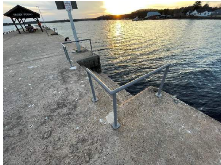
112- Structure D – West Steps, Stn 0+222 to 0+226
