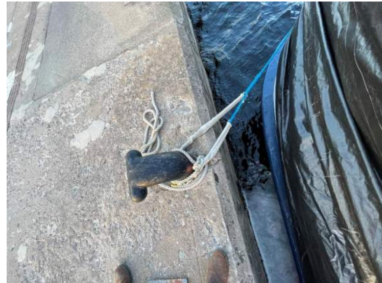
56- Structure D – East Bollard, Stn 0+144
