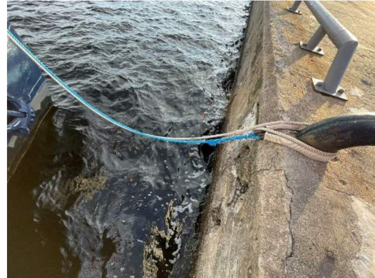
70- Structure D – East Bollard, Stn 0+159
