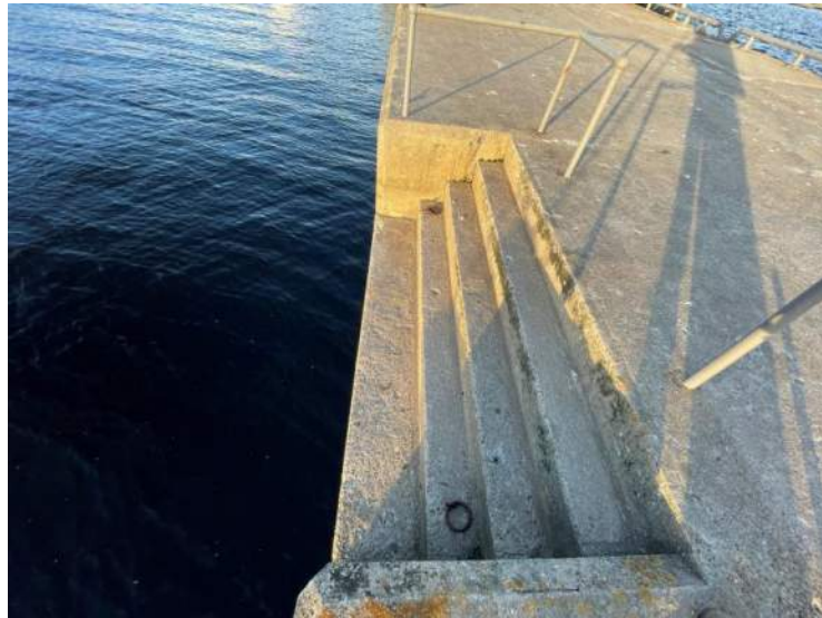
85- Structure D – West Steps (Looking North), Stn 0+176 to 0+180
