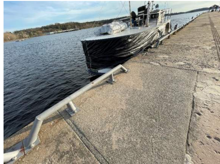
58- Structure D – Buried East Slipway, Stn 0+139 to 0+142
