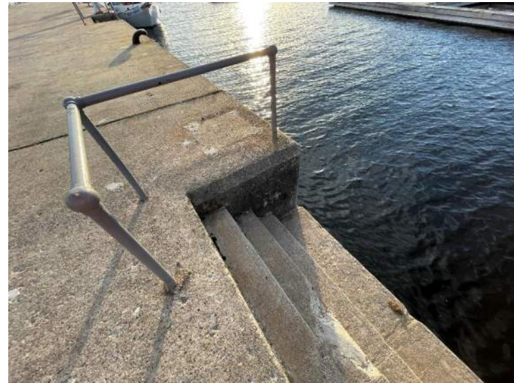
74- Structure D – West Steps (Looking South), Stn 0+161 to 0+164
