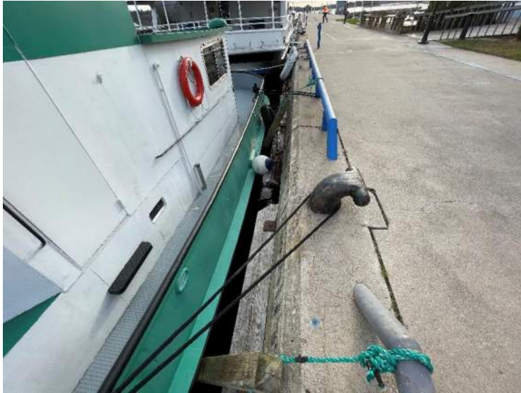
21- Structure C – East Bollard, Stn 0+076
