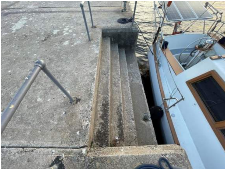
93- Structure D – West Steps (Looking South), Stn 0+192 to 0+196
