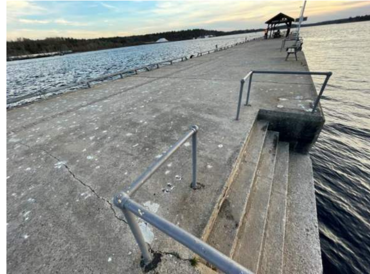
106- Structure D – West Steps (looking South), Stn 0+206 to 0+211
