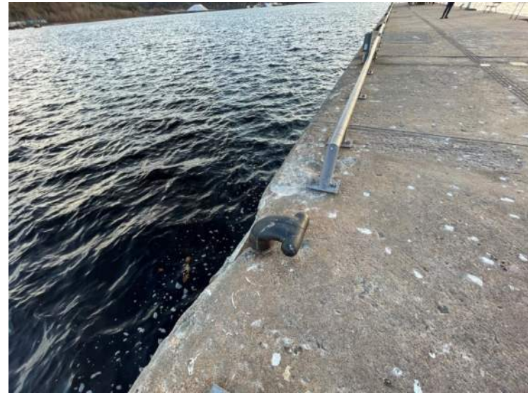
90- Structure D – East Bollard, Stn 0+190
