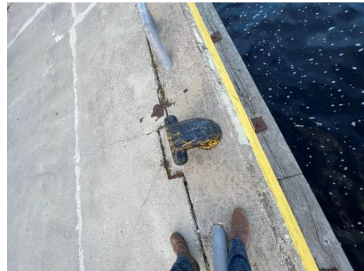
16- Structure C – East Bollard, Stn 0+057
