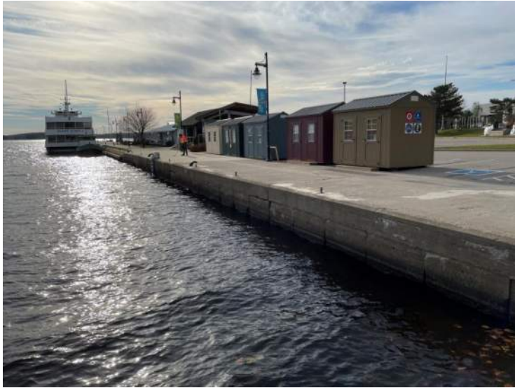
1- Bay St Wharf – East Face (looking South from shoreline)
