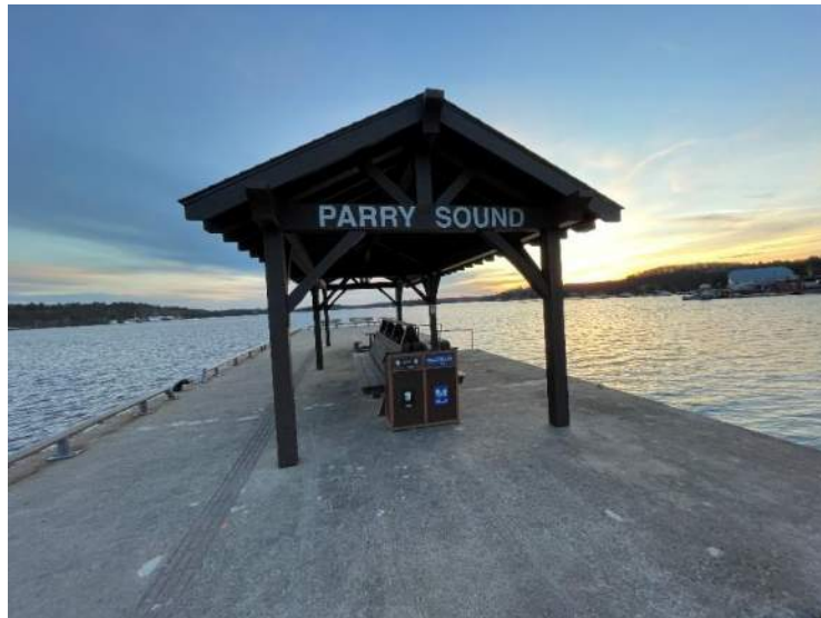
125- Structure D – Town Pavilion, Stn 0+245 to 0+268
