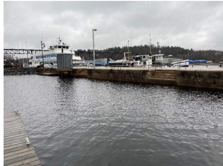
62- Structure D – West Face, Stn 0+126 to 0+168
