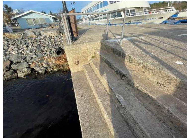
48- Structure D – West Steps (Looking North), Stn 0+131 to 0+134
