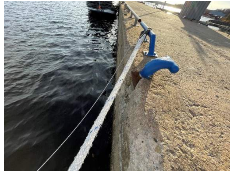
42- Structure D – East Face Bollard, Stn 0+129
