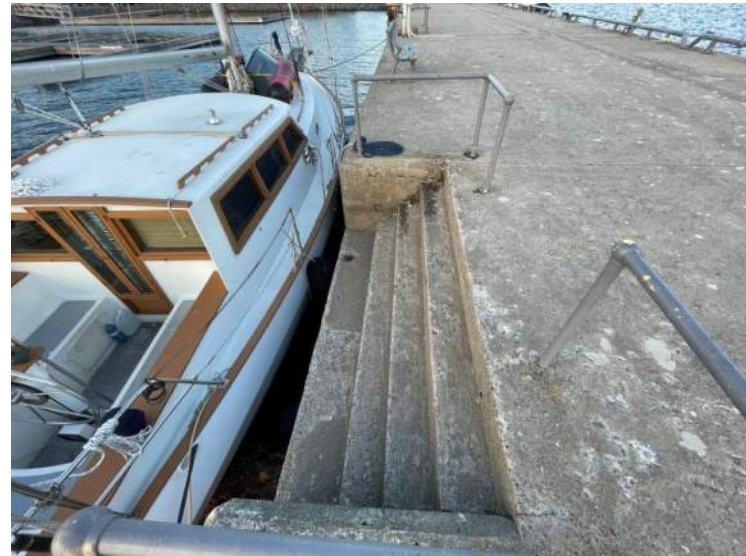
94- Structure D – West Steps (Looking North), Stn 0+192 to 0+196
