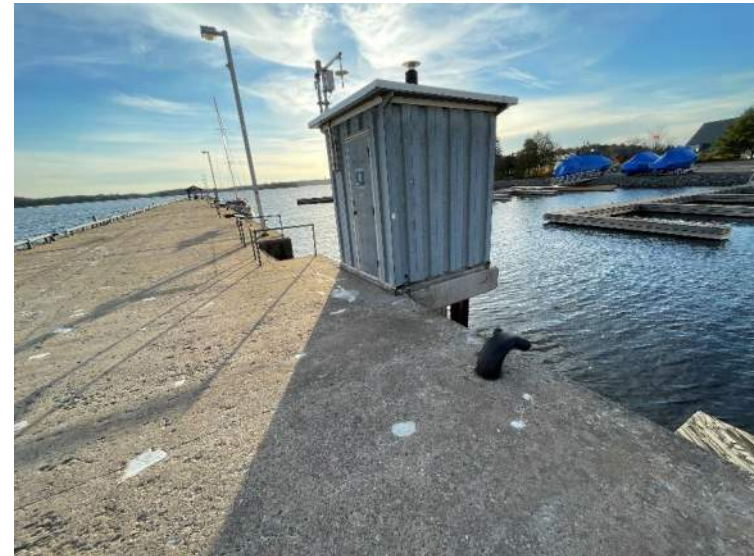
50- Structure D – Water Gage Station at West Edge, Stn 0+144
