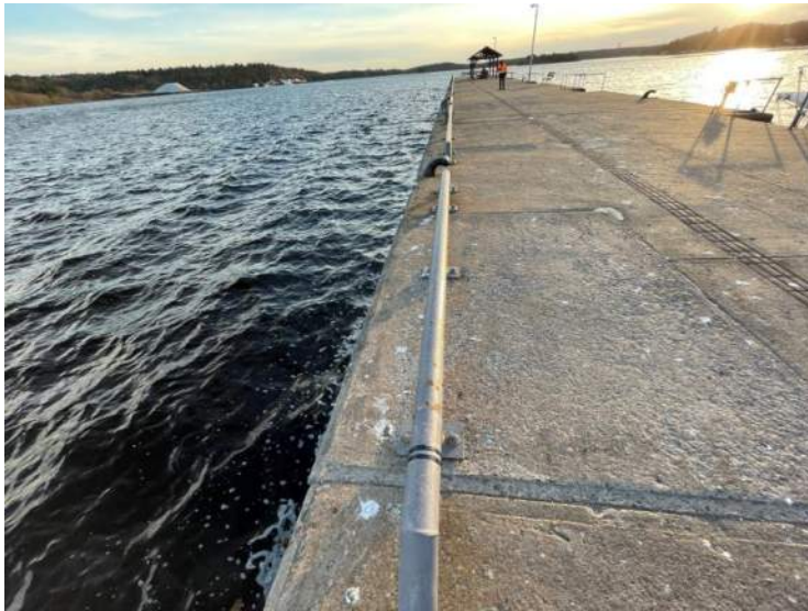
89- Structure D – Buried East Slipway, Stn 0+185 to 0+188
