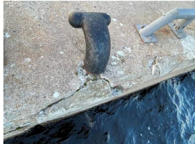
136- Structure D – East Bollard, Stn 0+266
