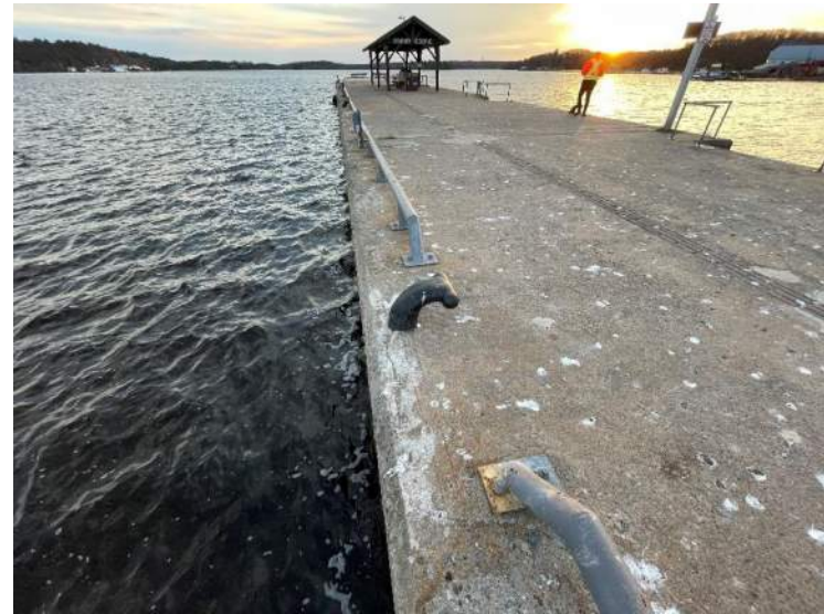
110- Structure D – East Bollard, Stn 0+221
