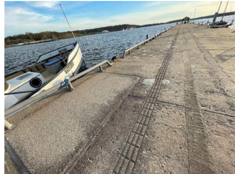
68- Structure D – Buried East Slipway, Stn 0+154 to 0+156
