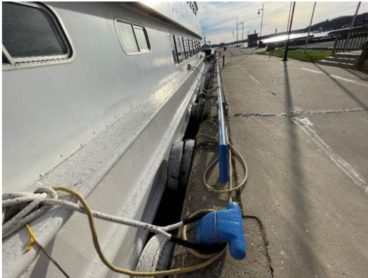
29- Structure C – Fenders along Island Queen Cruise Ship
