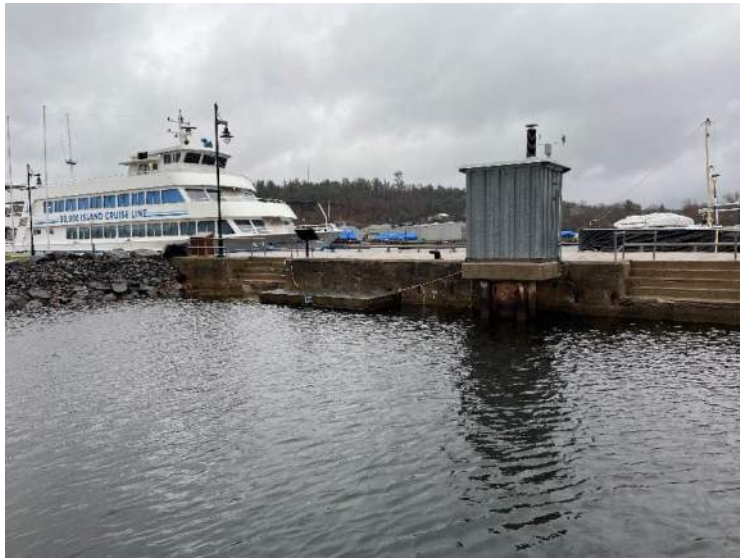
45- Structure D – West Face, Stn 0+126 to 0+148
