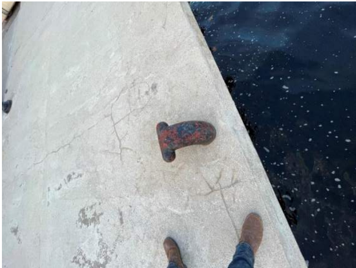
11- Structure B – East Bollard, Stn 0+047
