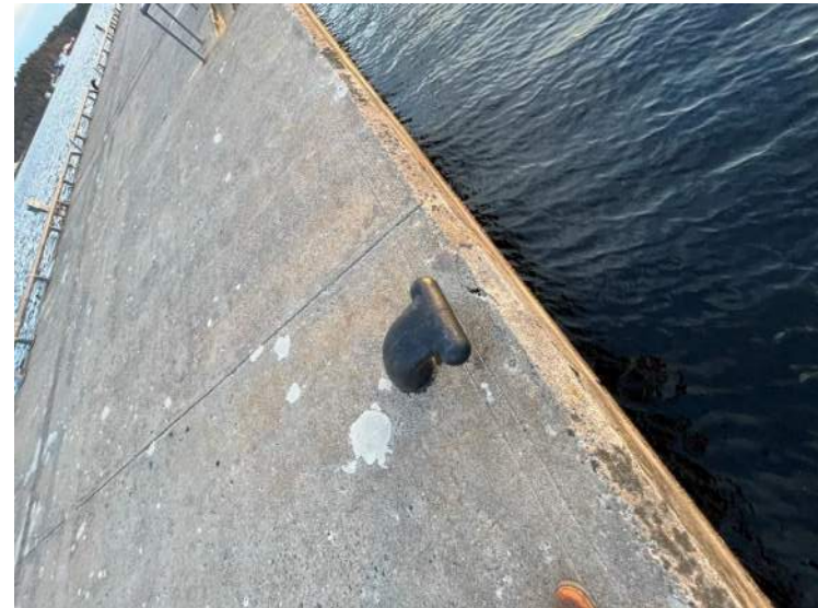
80- Structure D – West Bollard, Stn 0+170
