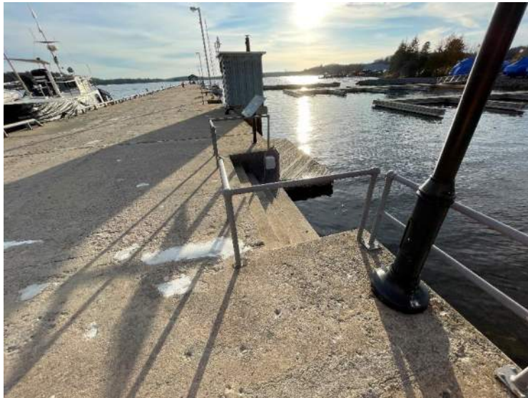
47- Structure D – West Steps, Stn 0+131 to 0+134
