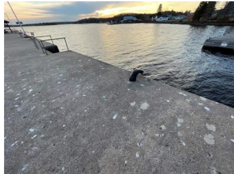
98- Structure D – West Bollard, Stn 0+201
