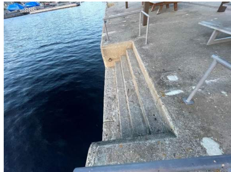
132- Structure D – West Steps (looking North), Stn 0+254 to 0+256
