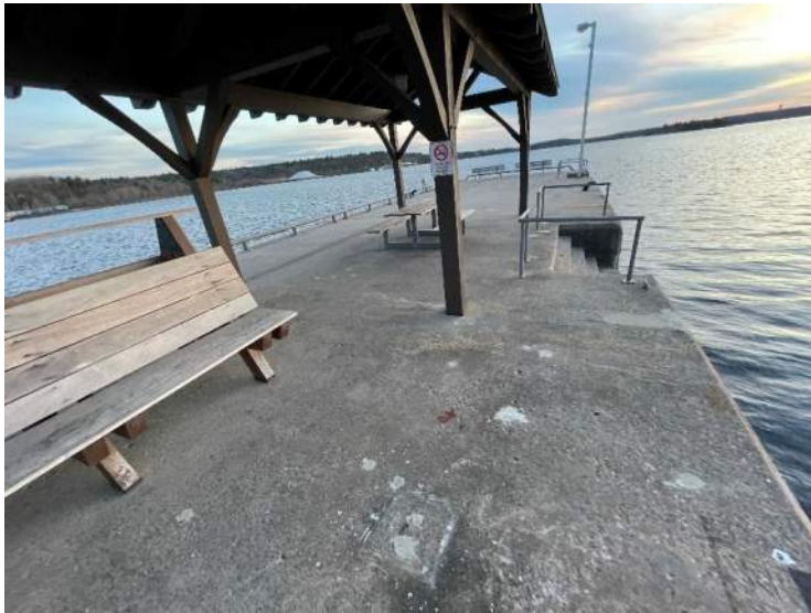
129- Structure D – Concrete Deck, Stn 0+250
