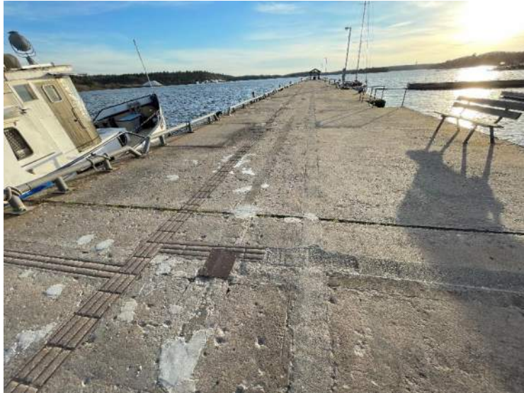
65- Structure D – Expansion Joint and Buried Conduits, Stn 0+151
