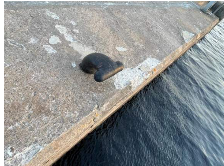
134- Structure D – West Bollard, Stn 0+264
