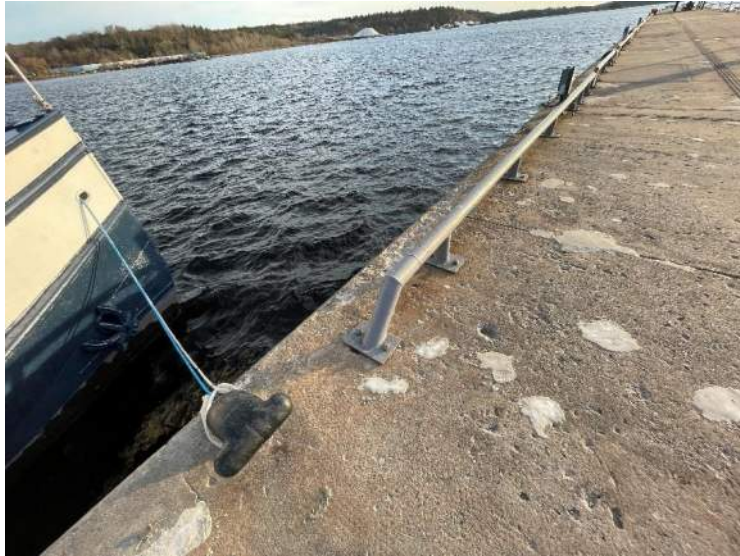
69- Structure D – East Bollard, Stn 0+159
