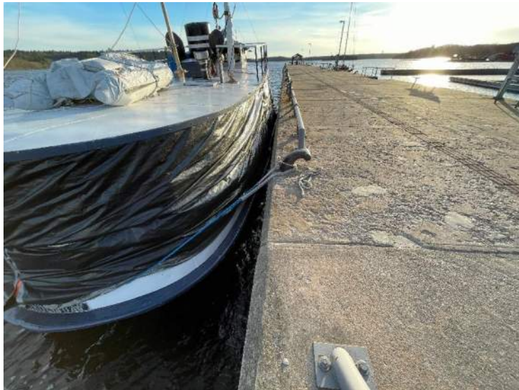
55- Structure D – East Bollard, Stn 0+144
