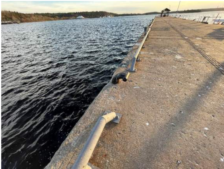
81- Structure D – East Bollard, Stn 0+175
