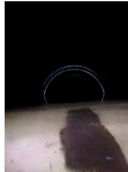
148- Structure B – Culvert Outfall inside Deck, Stn 0+039.5
