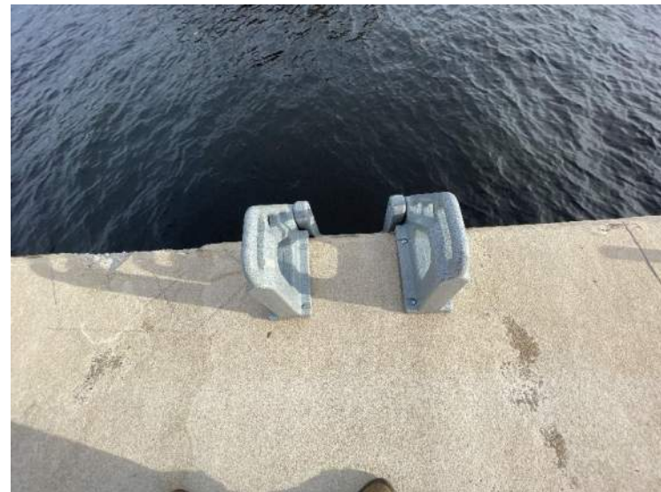
8- Structure B – Plastic Ladder, Stn 0+32
