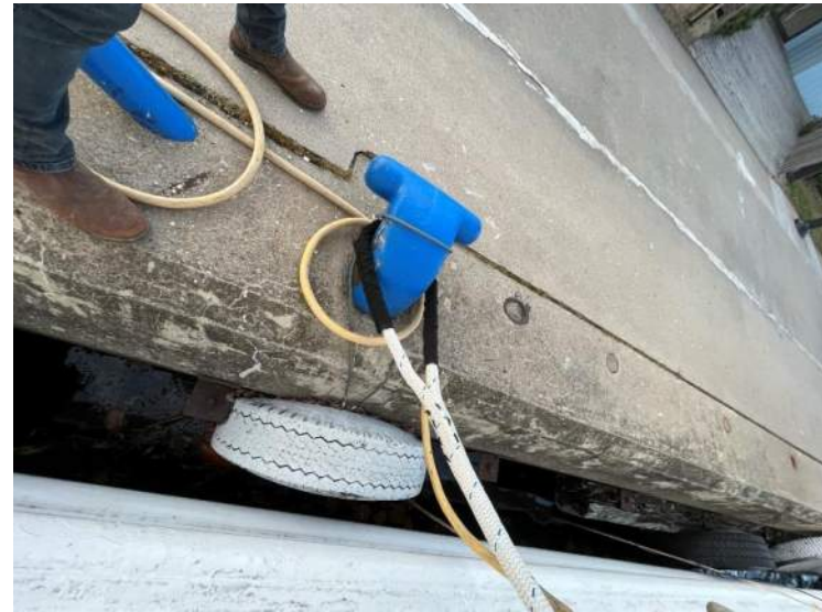
30- Structure C – East Bollard, Stn 0+94
