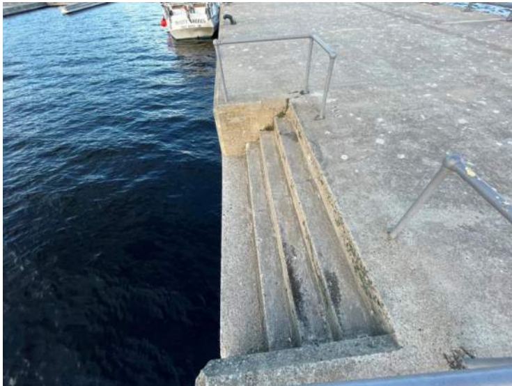
107- Structure D – West Steps (looking North), Stn 0+206 to 0+211
