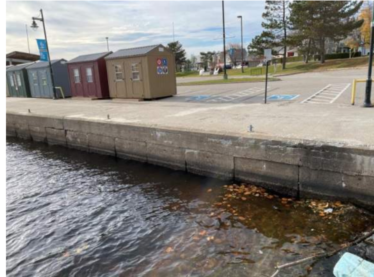
2- Structure A – East Face
