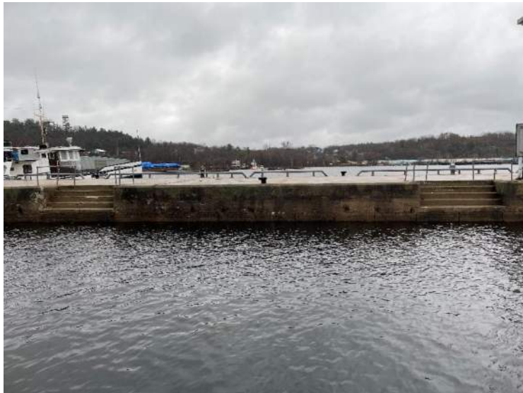
63- Structure D – West Face, Stn 0+160 to 0+180
