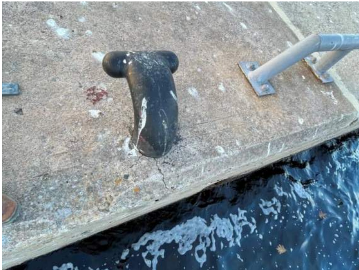
103- Structure D – East Bollard, Stn 0+206
