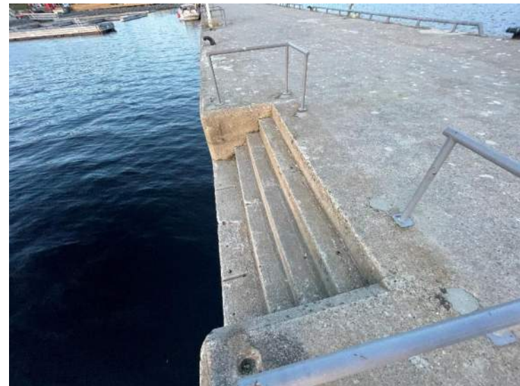
124- Structure D – West Steps (looking North), Stn 0+238 to 0+242
