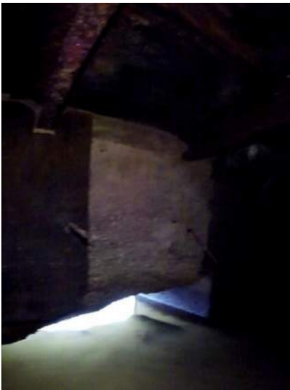
147- Structure B – Wall Opening (view from inside Deck), Stn 0+039.5
