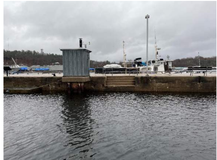
46- Structure D – West Face, Stn 0+135 to 0+155
