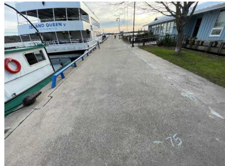
20- Structure C – Concrete Deck, Stn 0+075
