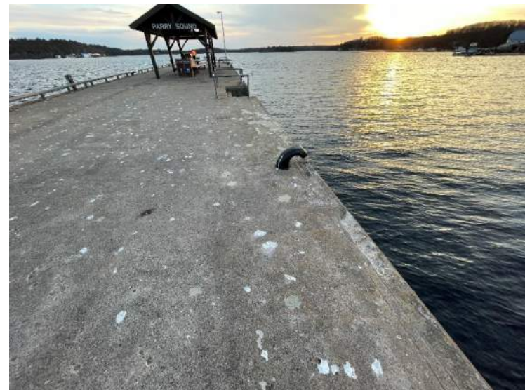
116- Structure D – West Bollard, Stn 0+232
