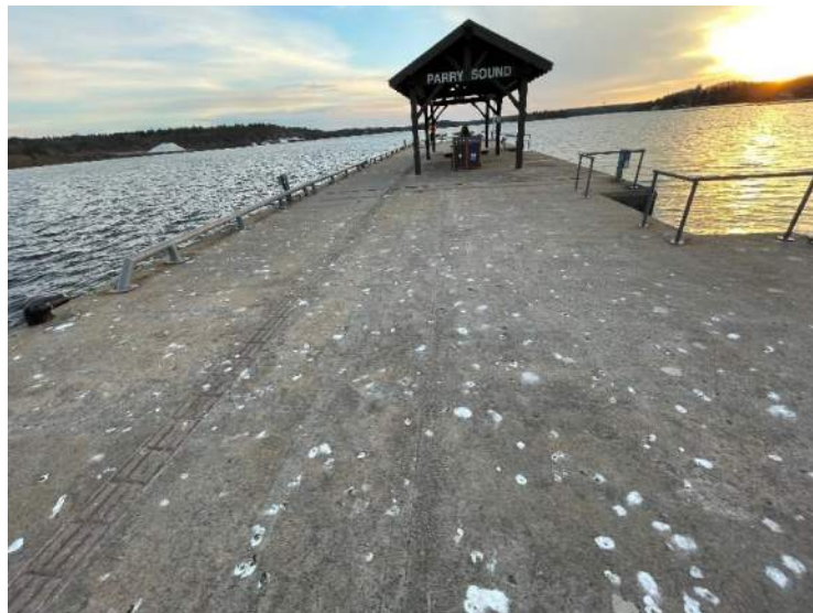
119- Structure D – Concrete Deck, Stn 0+235
