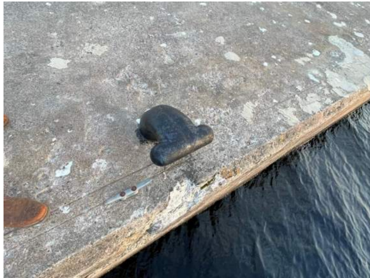
117- Structure D – West Bollard, Stn 0+232
