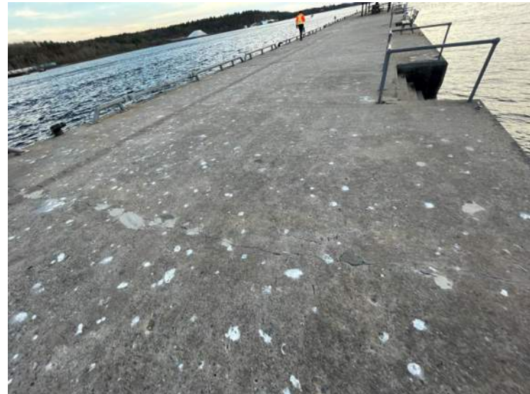
104- Structure D – Concrete Deck, Stn 0+206
