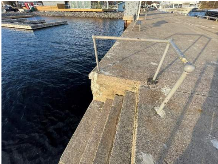
73- Structure D – West Steps (Looking North), Stn 0+161 to 0+164
