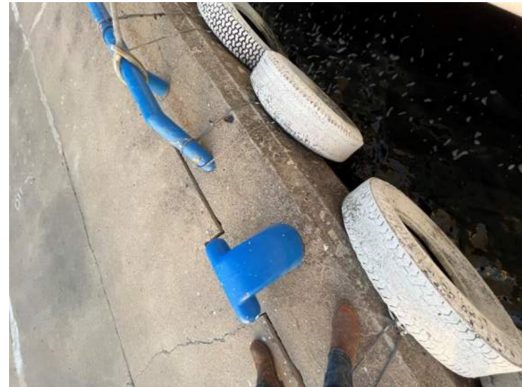
34- Structure C – East Bollard, Stn 0+113
